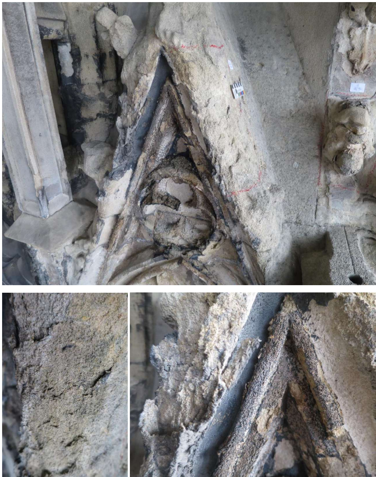
Figure S10. Intermediate restoration state, during the cleaning procedure and before treatment application. The rain exposed surfaces marked in red (top figure) have been used for consolidation purposes in the frame of this work. Bottom figures exhibit the differences in densities and decay patterns.
