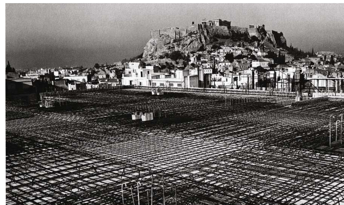
Bottom: Transformation of Athens' building stock with the Polykatoikia housing model and urban expansion through Antiparochi . Reinforced concrete roof slab in central Athens, 1950s (Dimitris Charisiadis, Benaki museum in lifo.gr).
