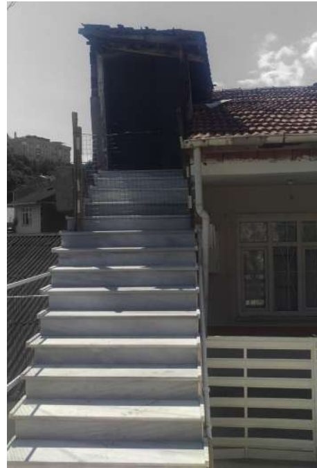
Fig 127 Direct access to the second floor from street via exterior stairs
