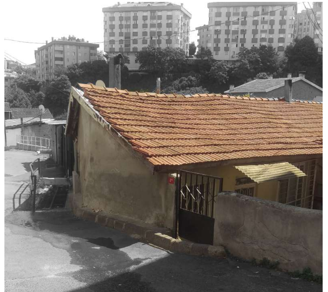
Fig 66 Typical one-storey buildings
