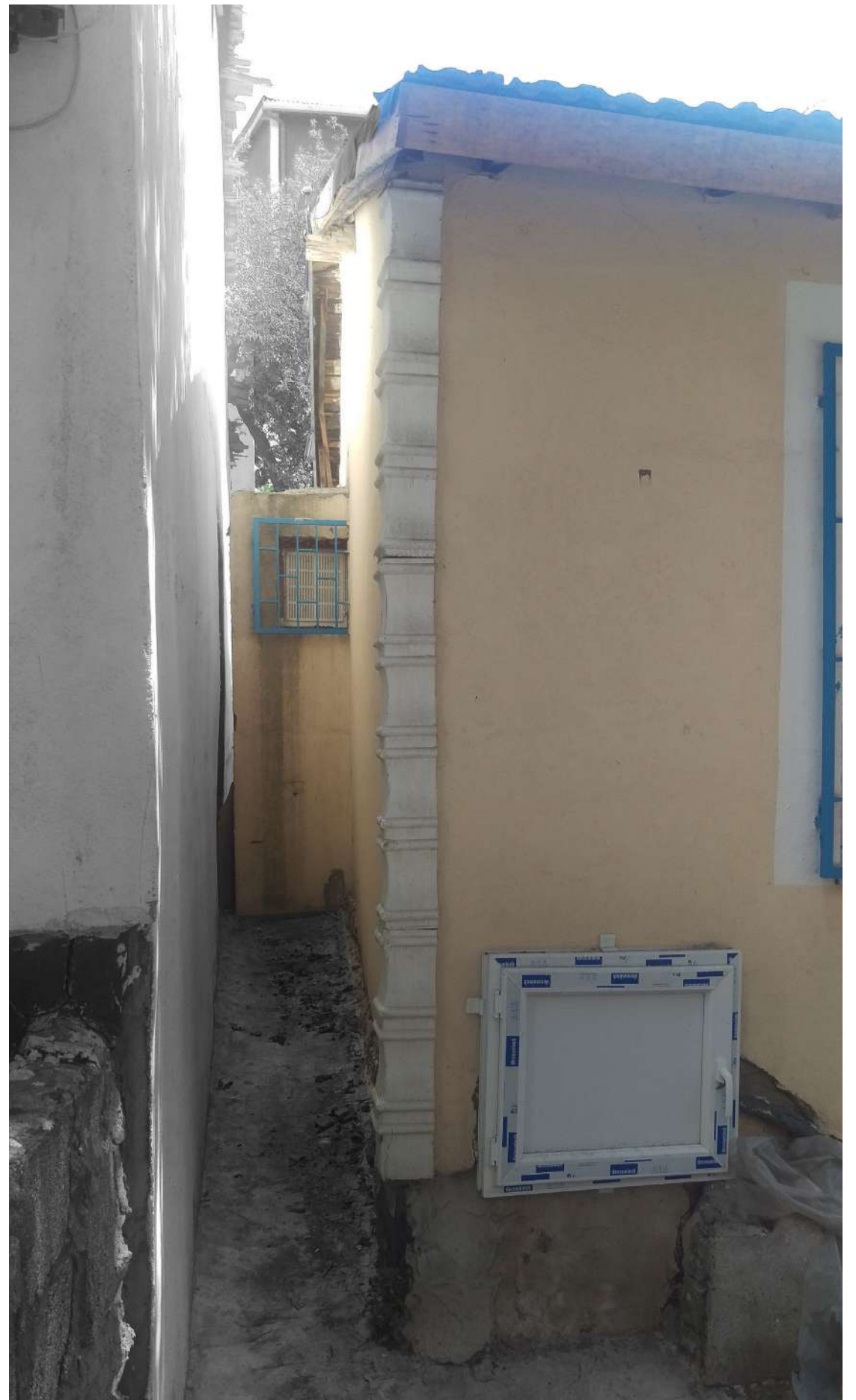
Fig 135 Problems with not used spaces due to construction without plan and later made expansions
