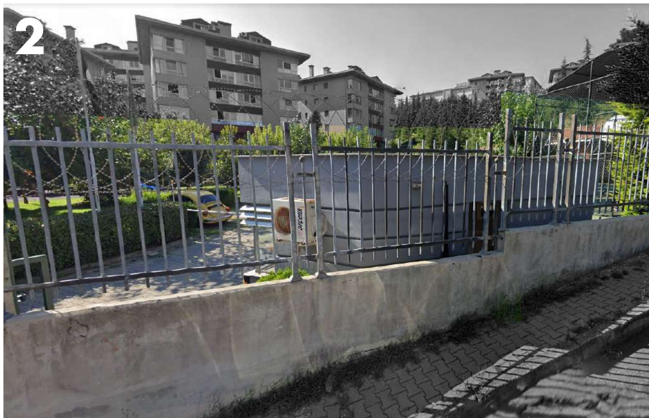
Fig 113 Protection Wall of Gated Community
