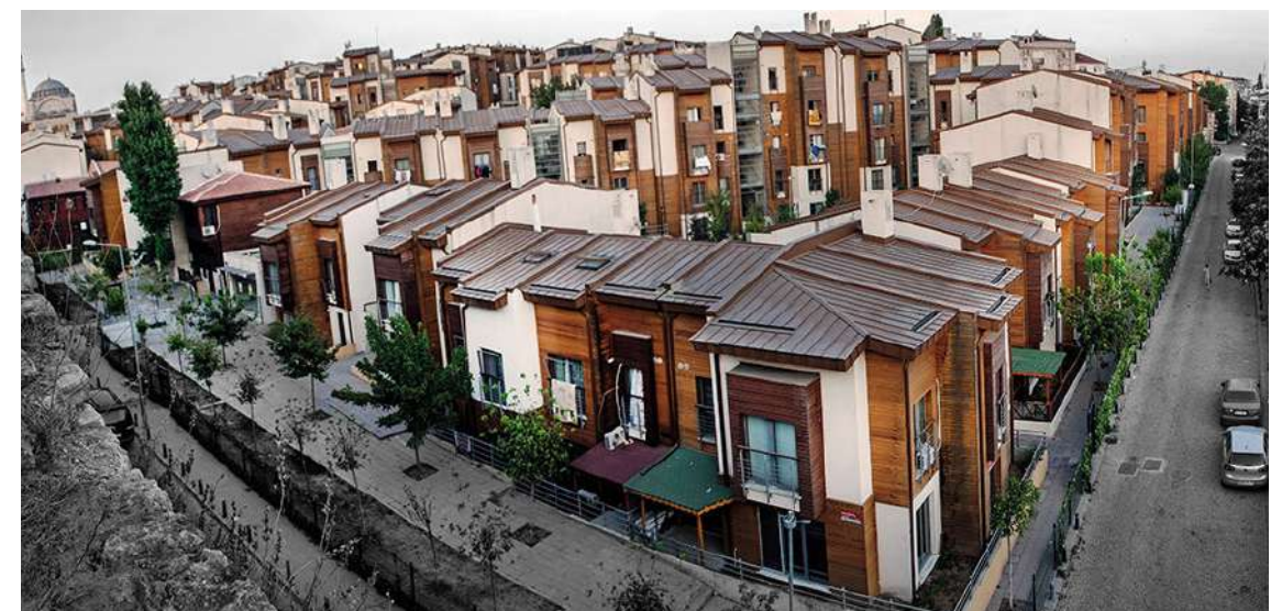
Fig 21 Sulukule Implemented Project
