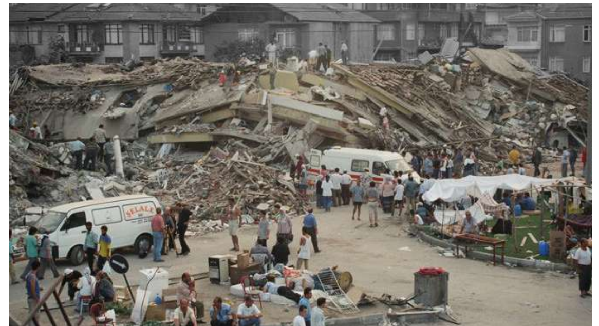
Fig 9 Debris after the earthquake in Marmara Region in 1999
