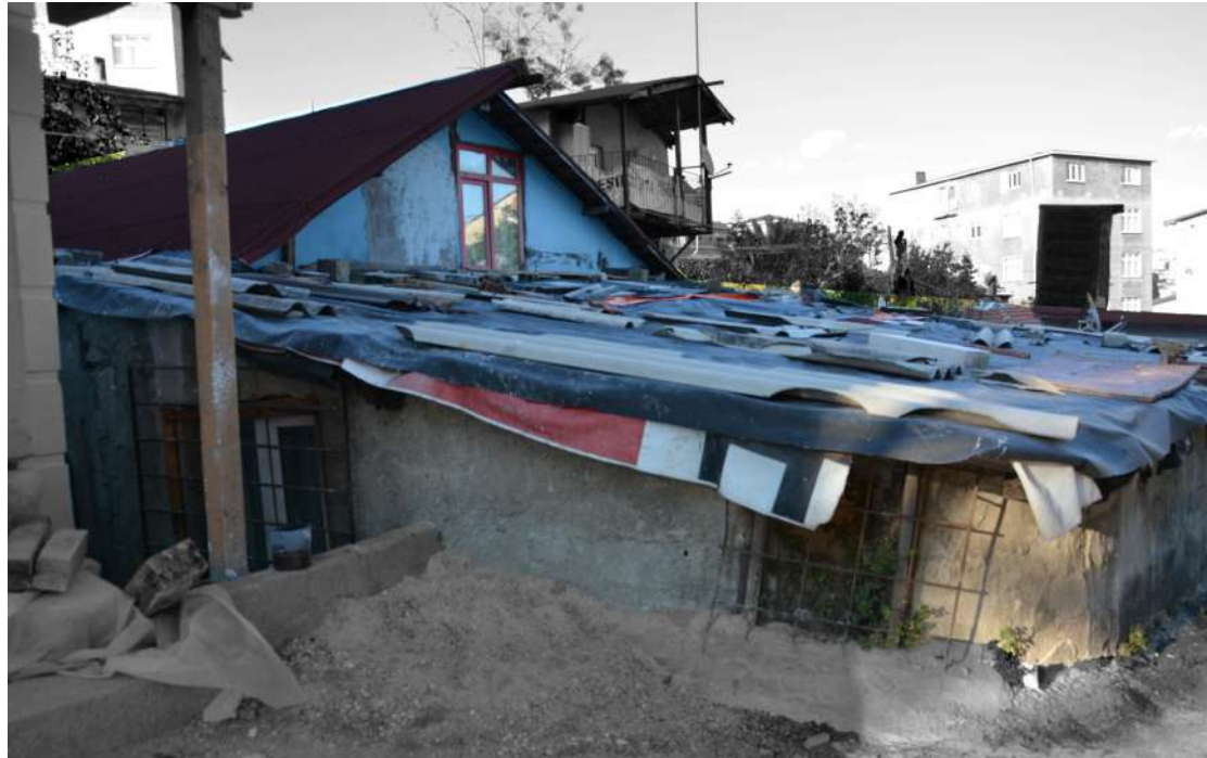
Fig 130 Problems with privacy and lighting due to street window positioning
