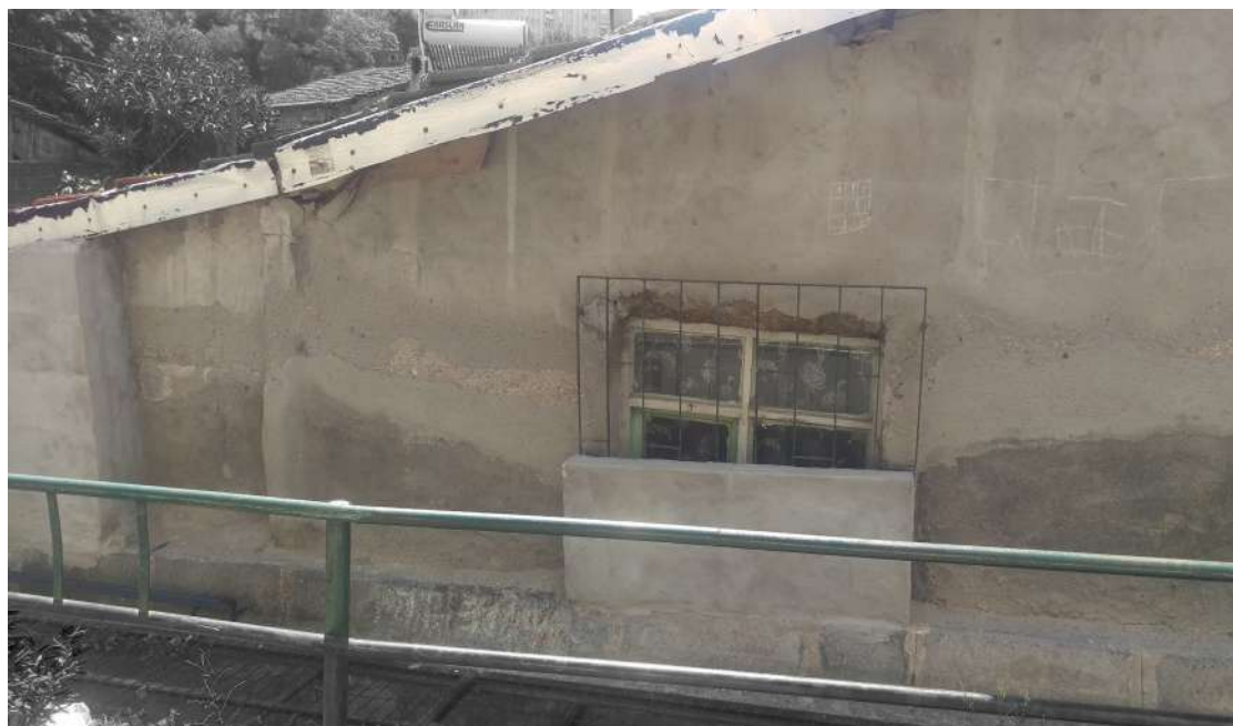
Fig 132 Problems with lighting and ventilation due to street house height relation
