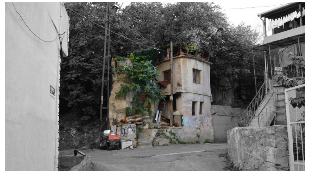
Fig 133 Run down houses without any possibility of repair
