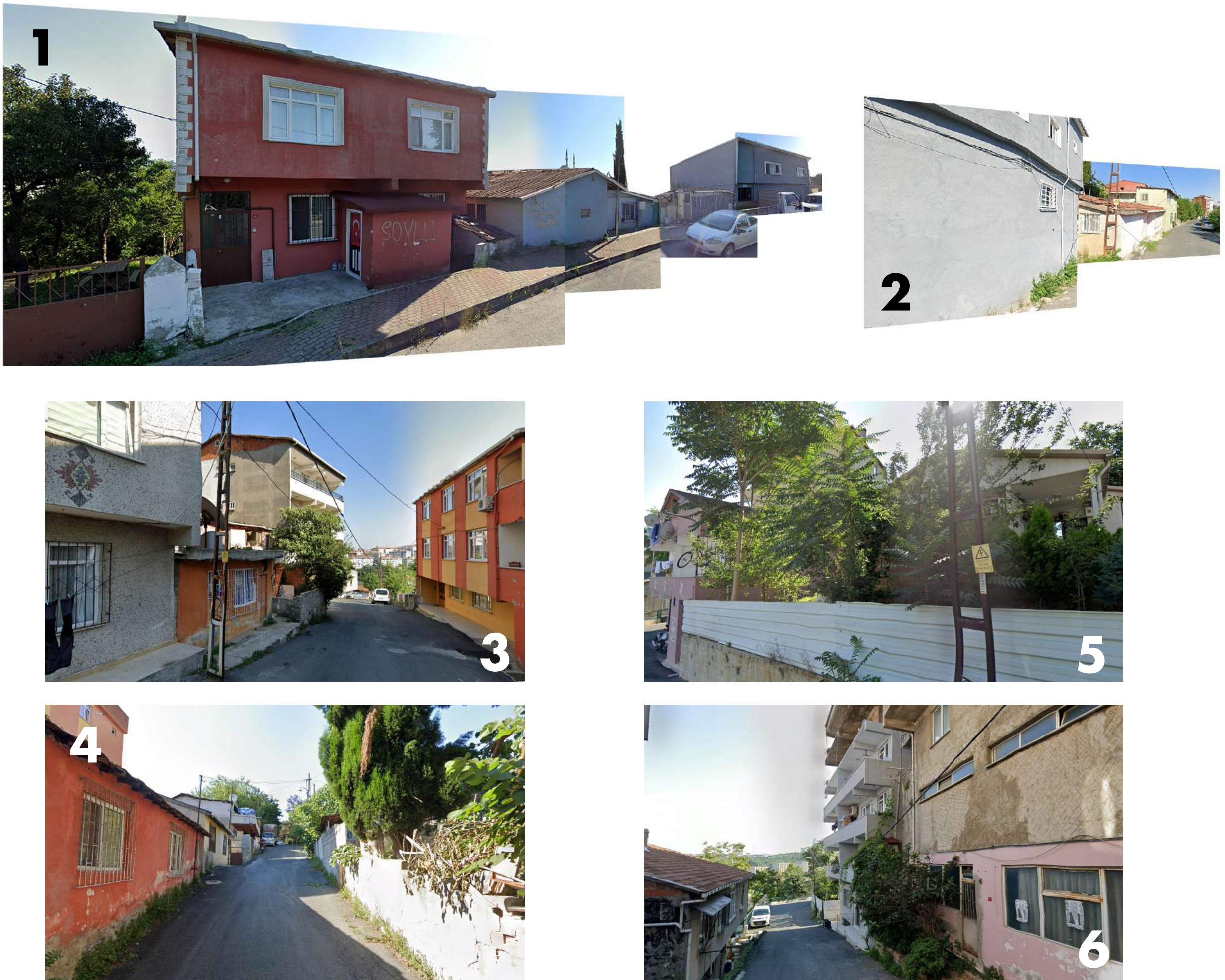
Fig 150 Fotos of the existing structure in the Interventionpoint 1
