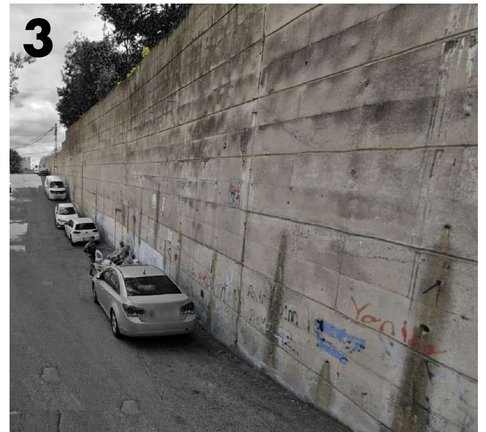
Fig 114 Protection Wall of Darüssafaka Education Facility
