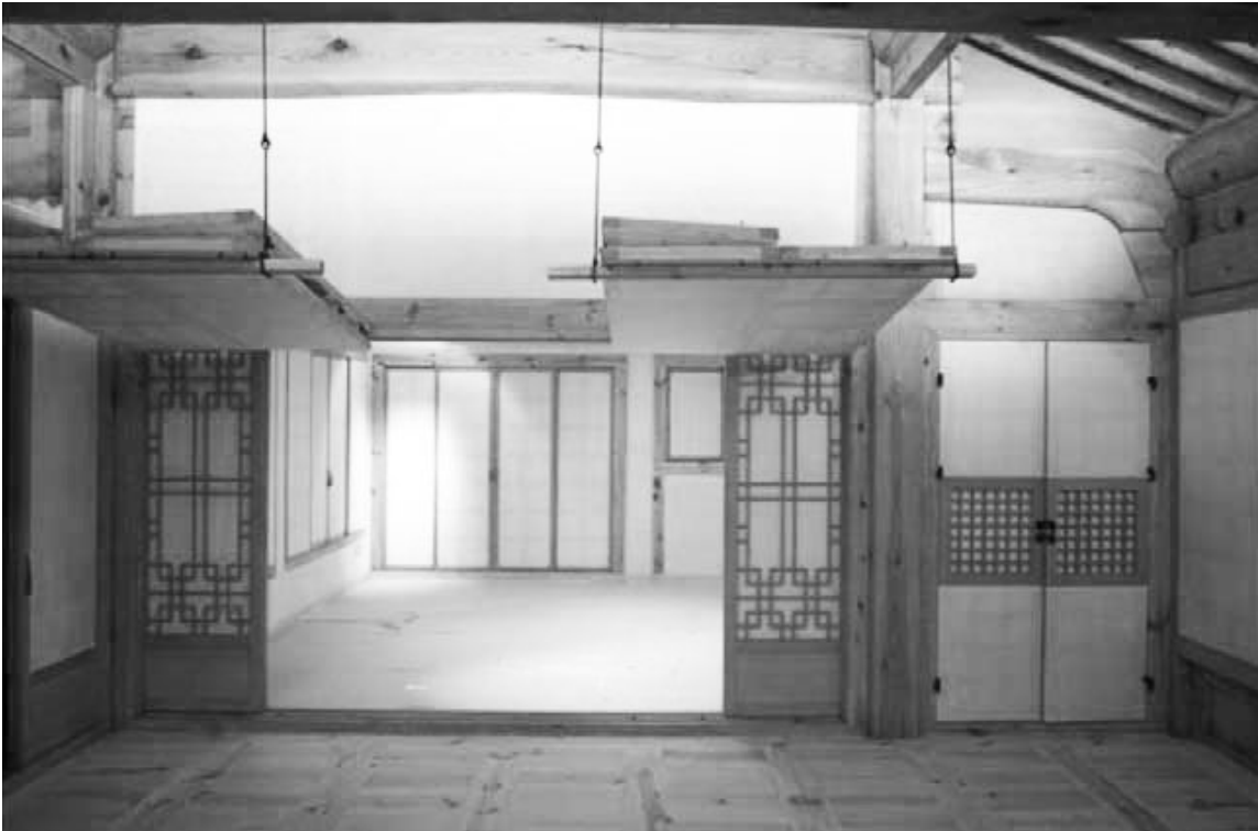
Opened bunhap-mun of a Korean traditional house (Haksajaein Gangwha, 2000)
