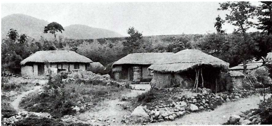
Hanok and Choga with straw fence
