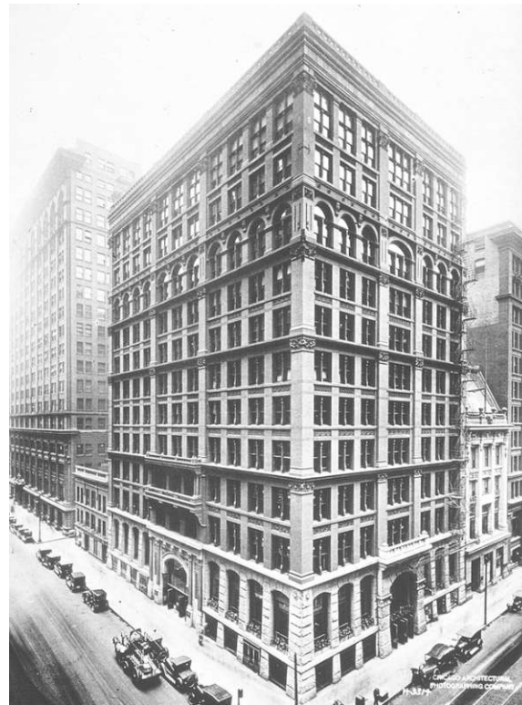
Fig.9: Home Insurance Building, Chicago, 1894
