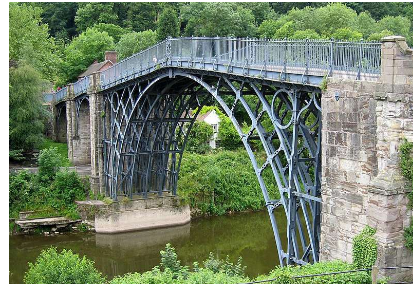
Fig.6: The first Cast Iron Bridge, Coalbrookdale
