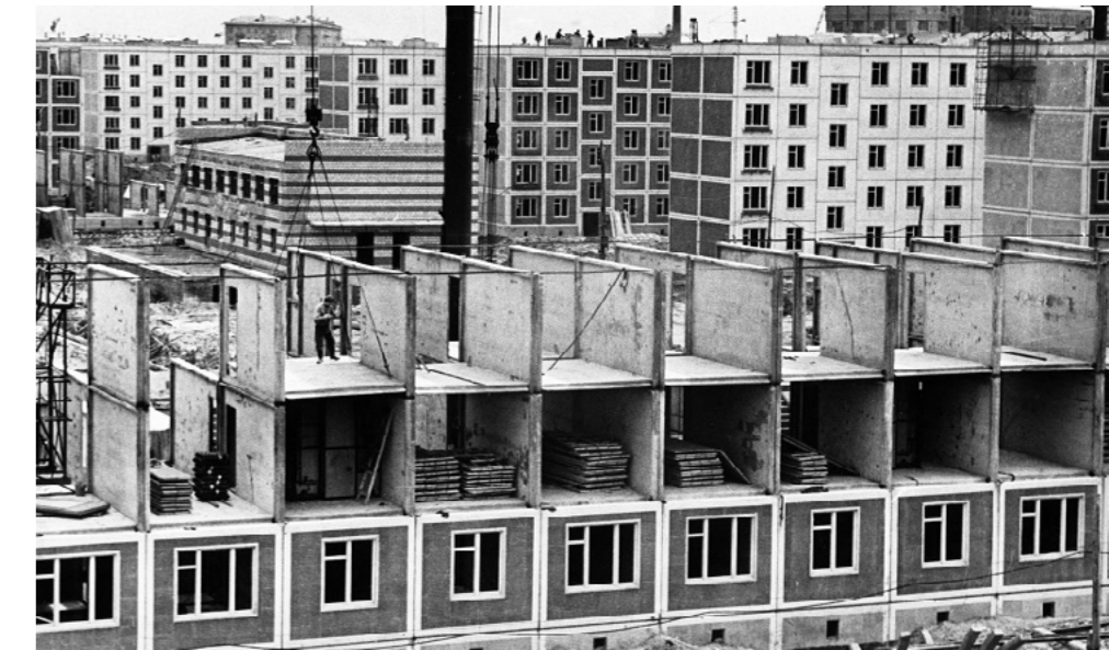
Construction in progress. [25]
