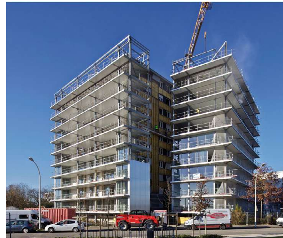
During the reconstruction of houses in Saint-Nazaire, in addition to expanding the facade due to glazed terraces, two significant in size volumes were completed on the sides of the building. Lacaton & Vassal Architectes, Saint-Nazaire, France. [5]
