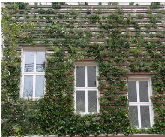
Figure 15 GRG 7, facade greening systems
