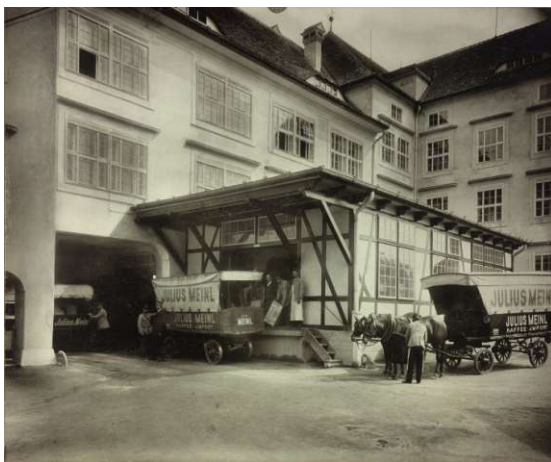
Figure 31 Julius Meinel factory yard (1925)
