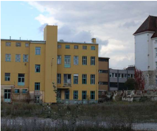
Figure 34 existing storage building
