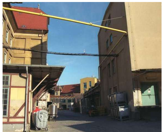
Figure 33 Julius Meinel factory yard (1999)
