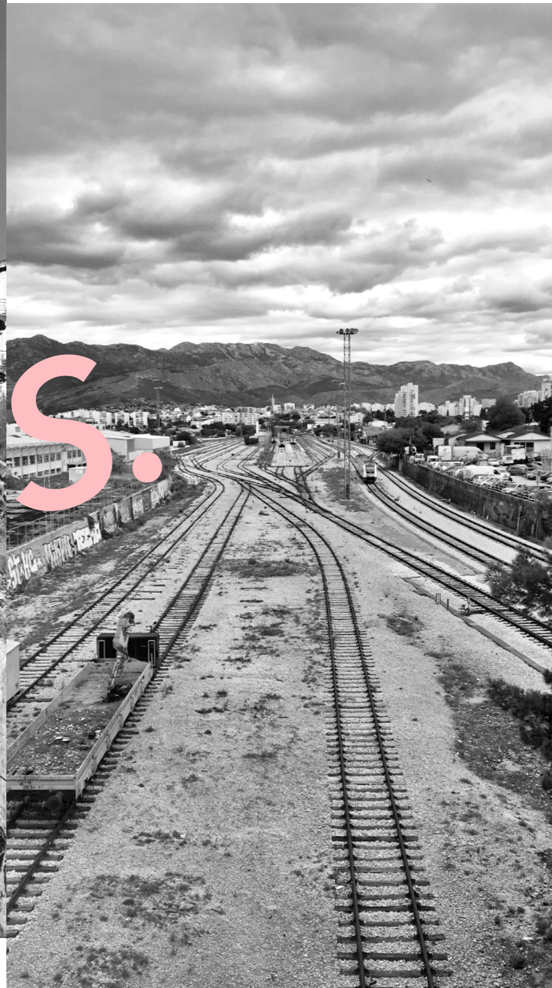
Fig. 132. Split Predgrade station
