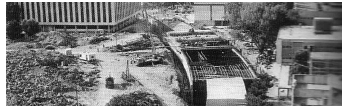
Fig. 43. Construction of a subway station
