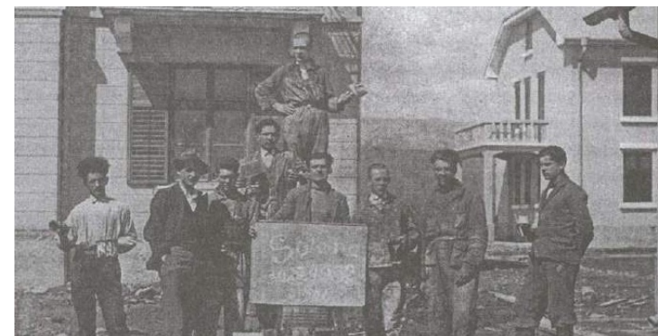
Fig.9 Construction workers in 1932
