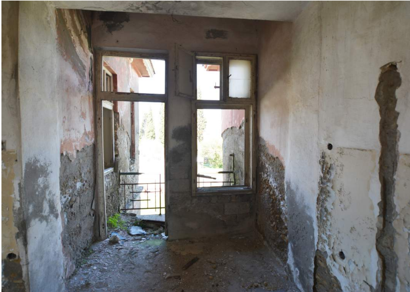
Fig.106 Current hall situation
