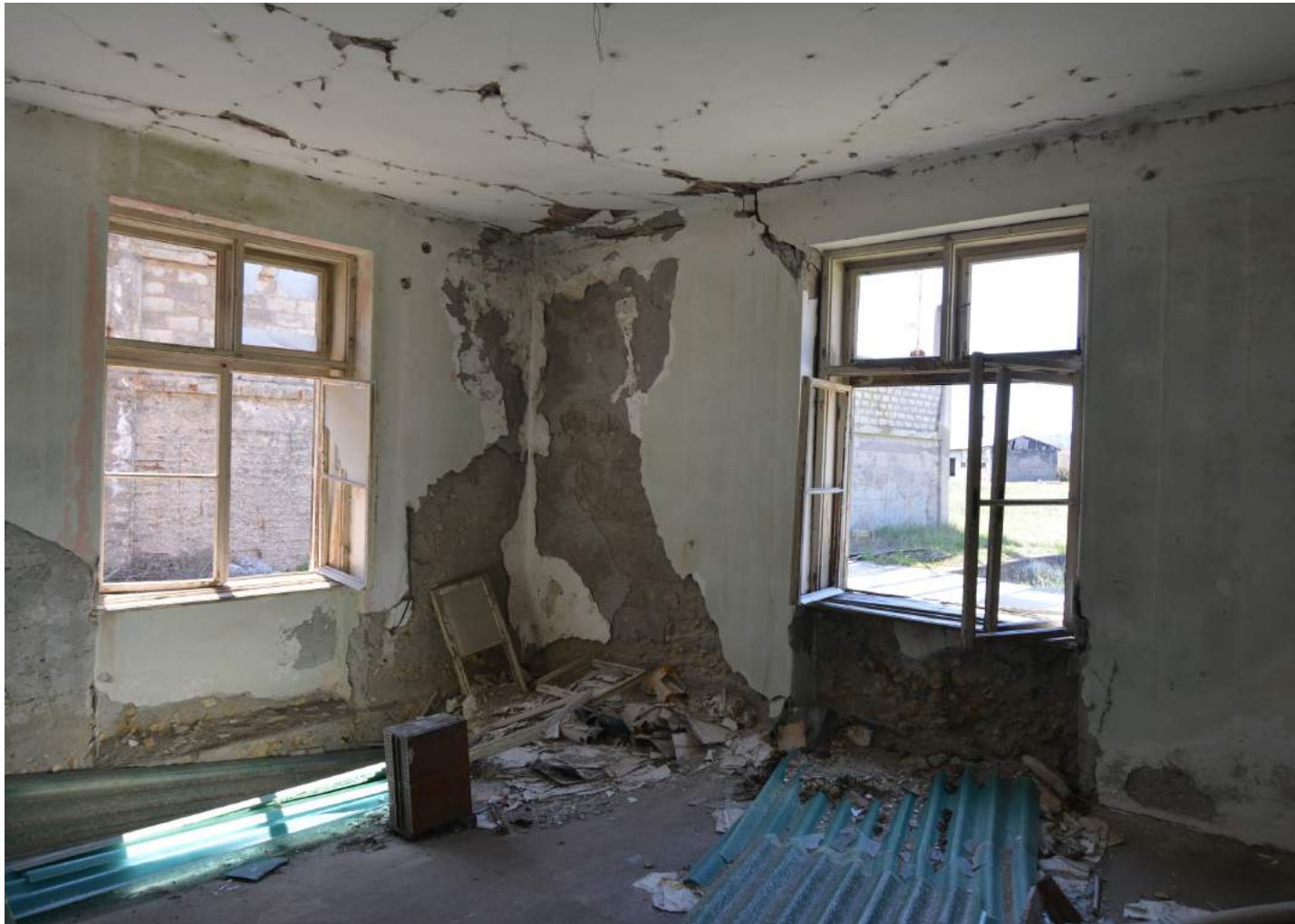
Fig.97 Current room situation
