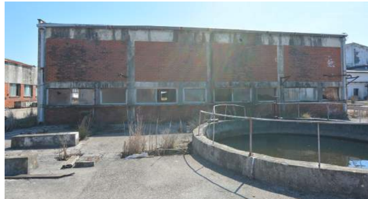
Fig.71 Air compressor station
