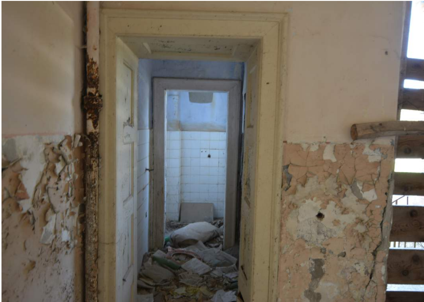
Fig.99 Current toilette situation
