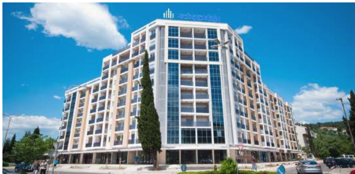
Fig.130 The new residential building that has taken its place
