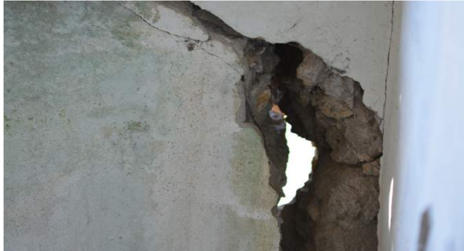
Fig.152 Interior wall cavity
