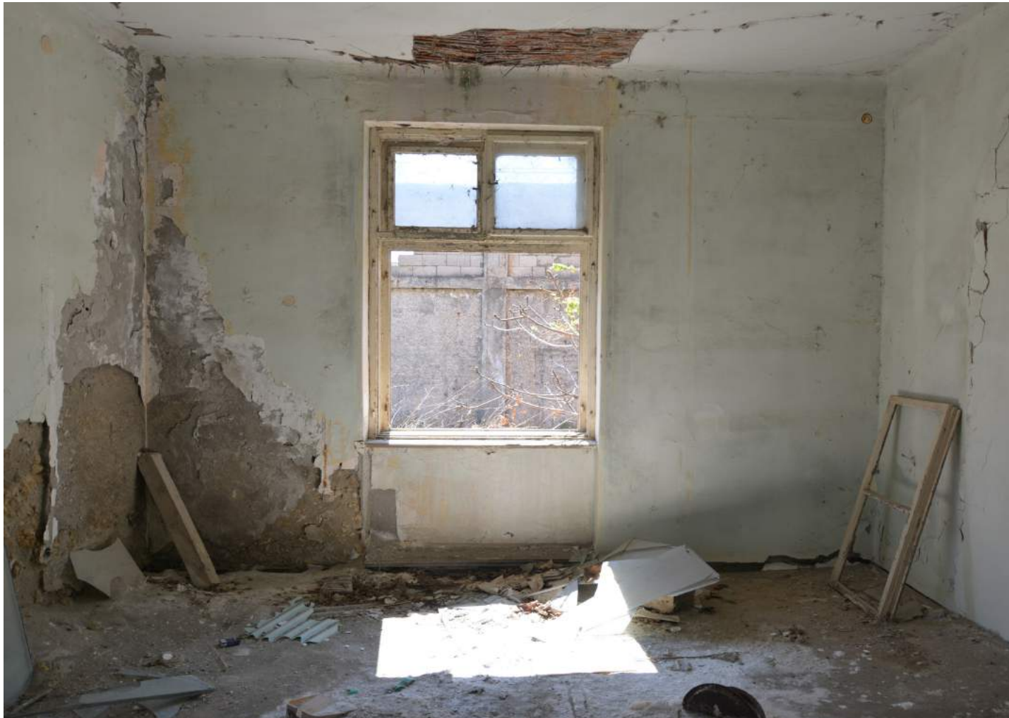
Fig.91 Current room situation
