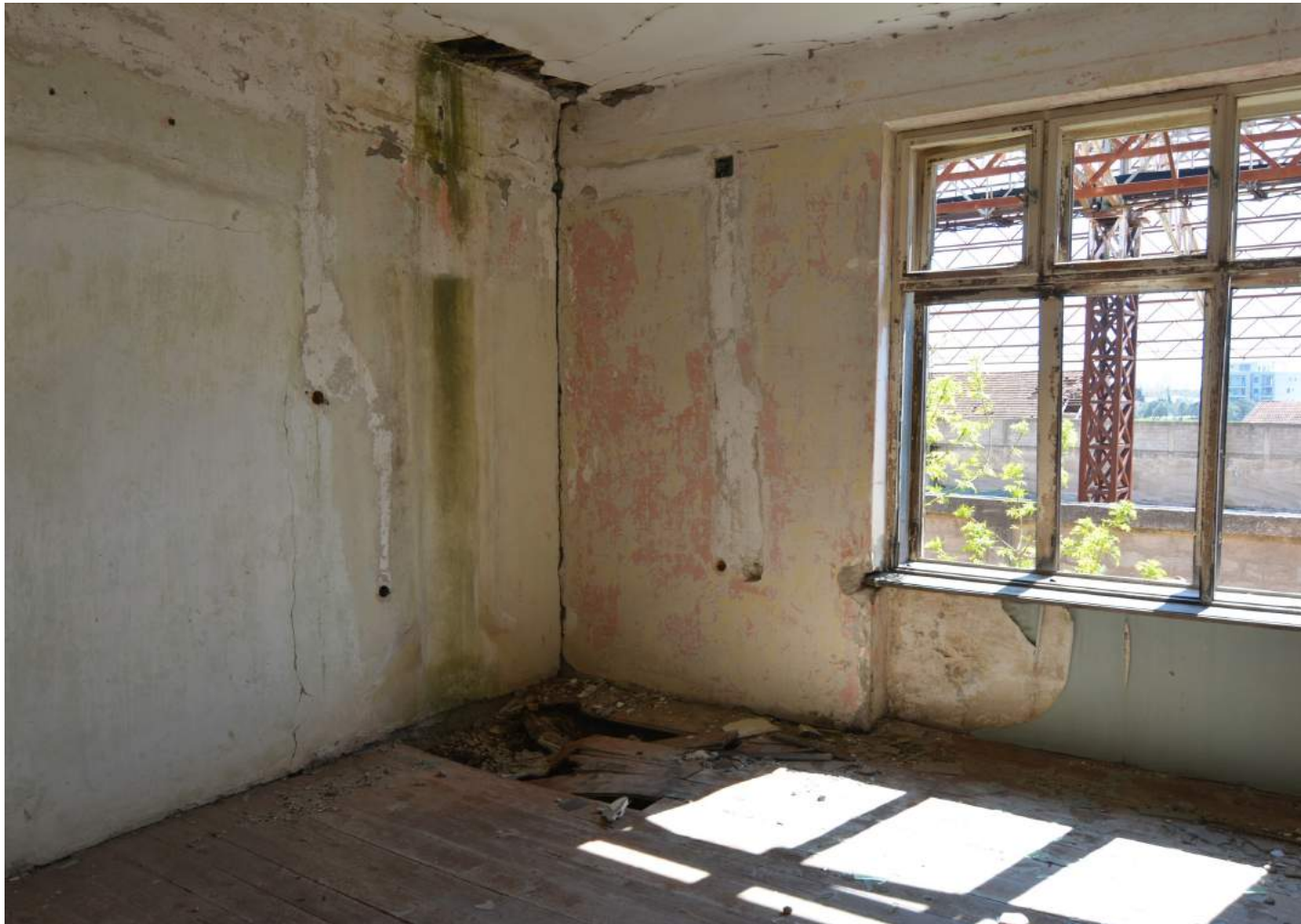
Fig.107 Current room situation
