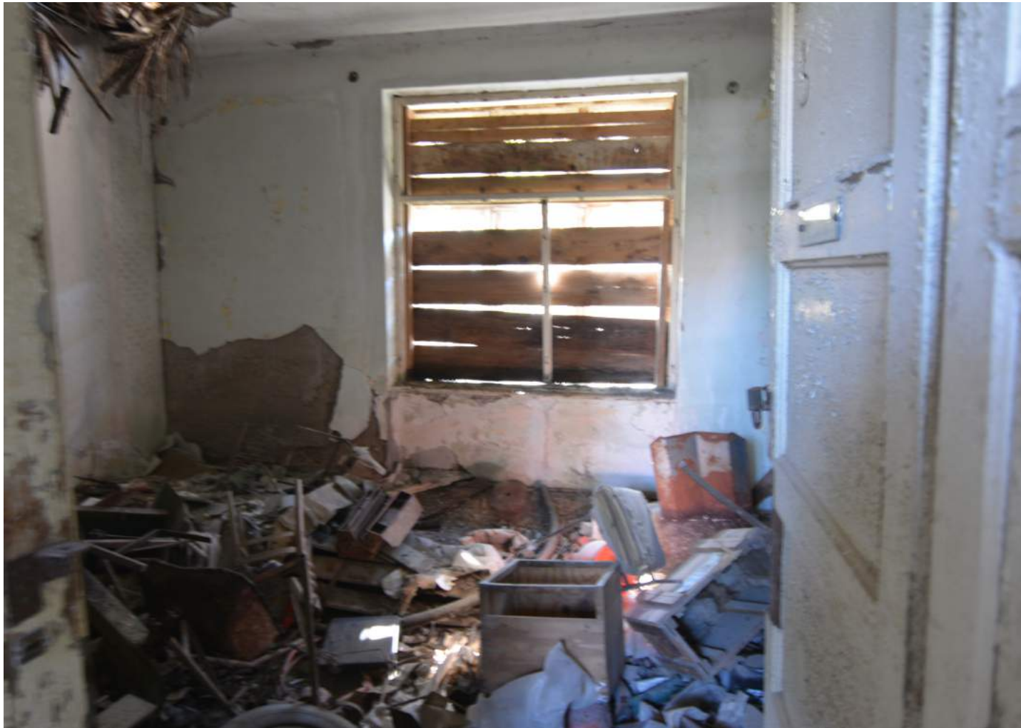
Fig.96 Current room situation
