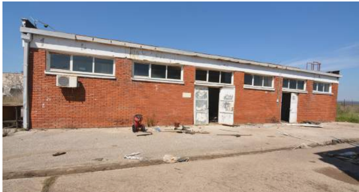
Fig.68 Spare parts warehouse
