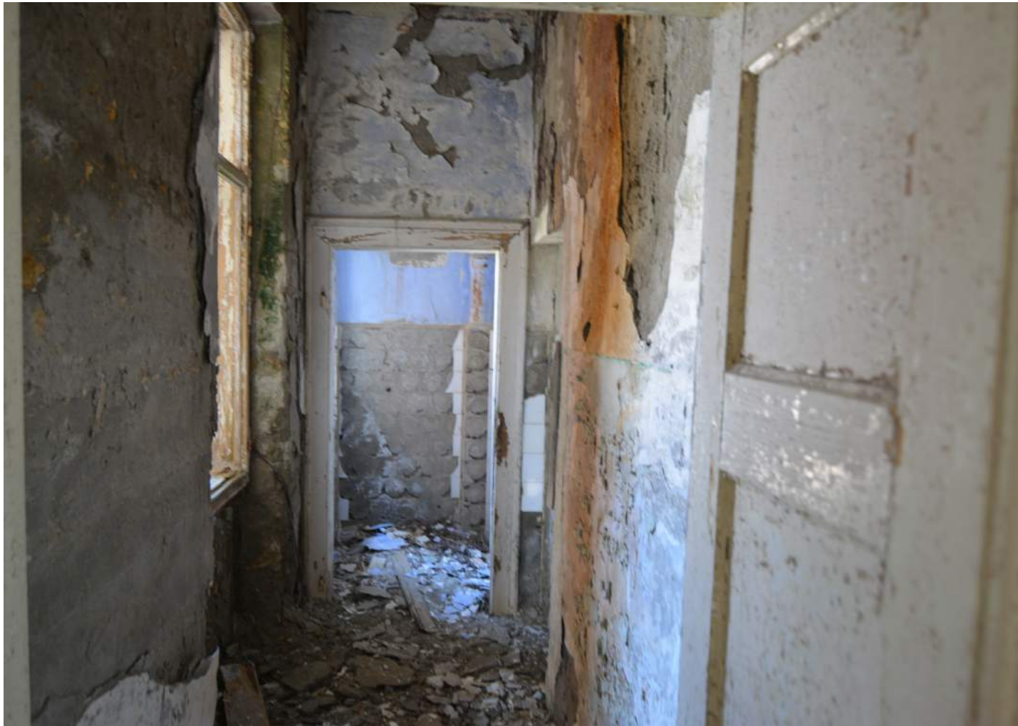
Fig.105 Current toilette situation
