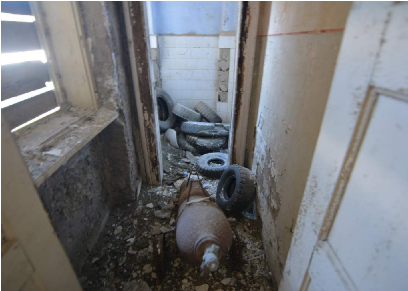
Fig.93 Current toilette situation
