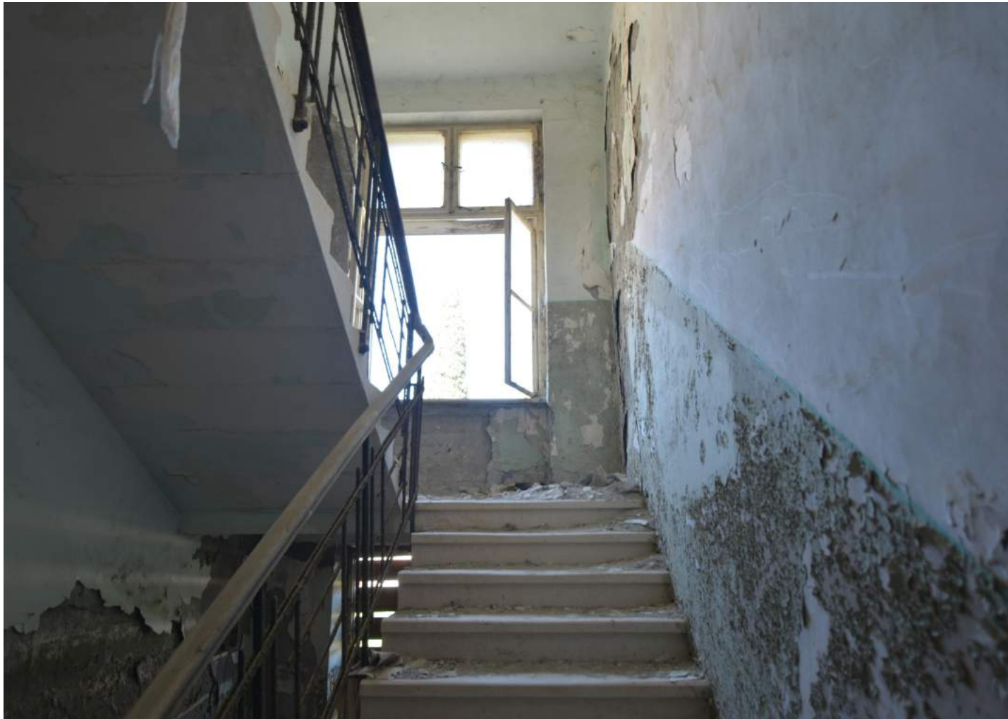
Fig.100 Current staircase situation
