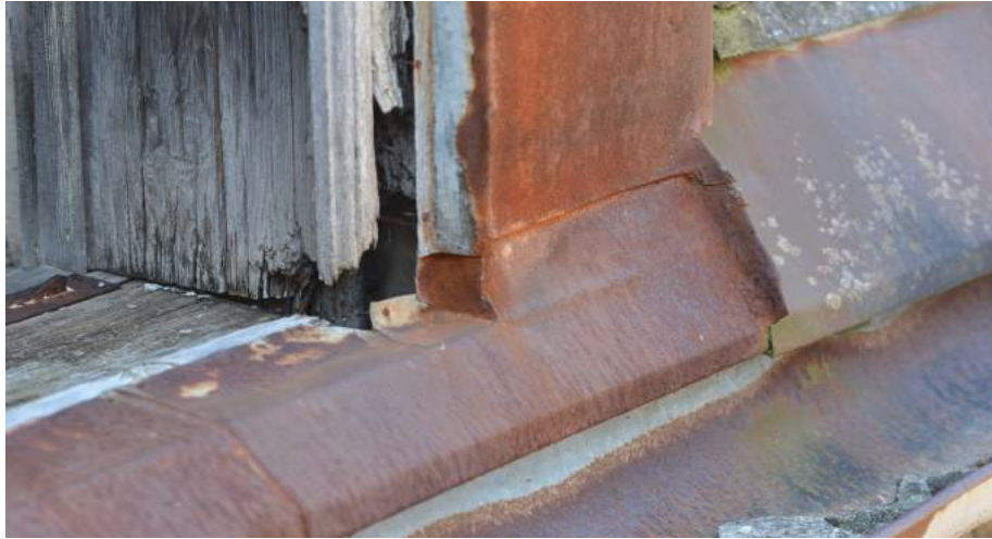
Fig.163 External metal framing and rain gutter
