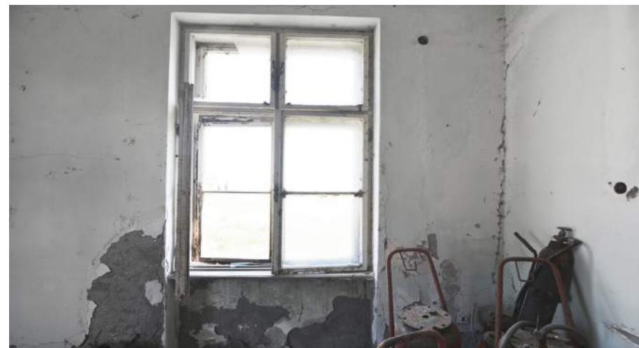
Fig.139 All radiators have been removed
