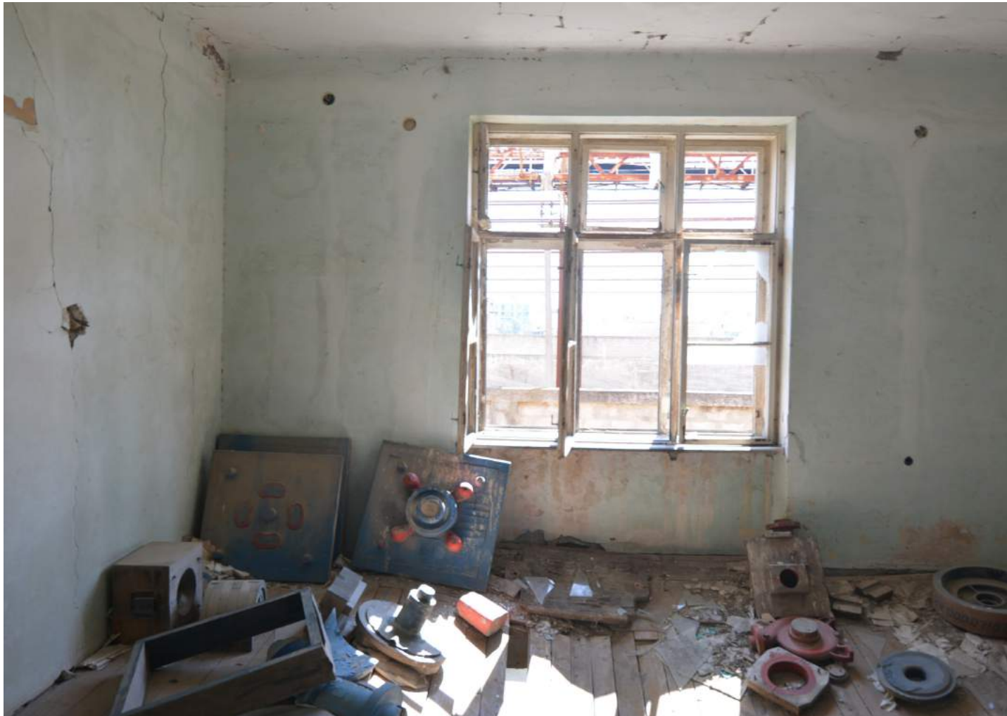
Fig.104 Current room situation
