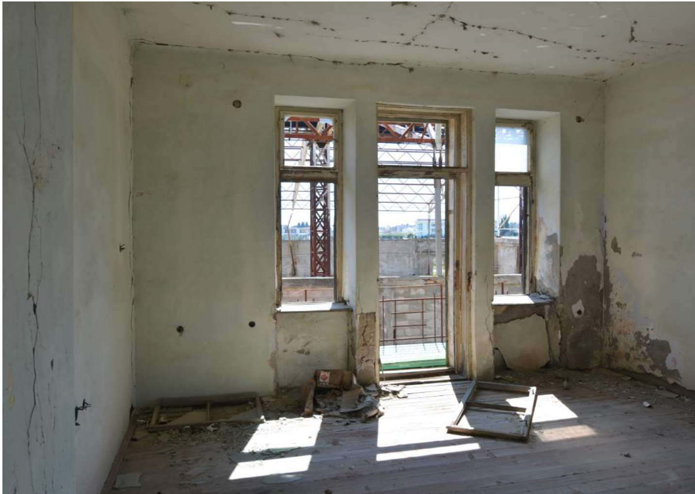
Fig.108 Current room situation
