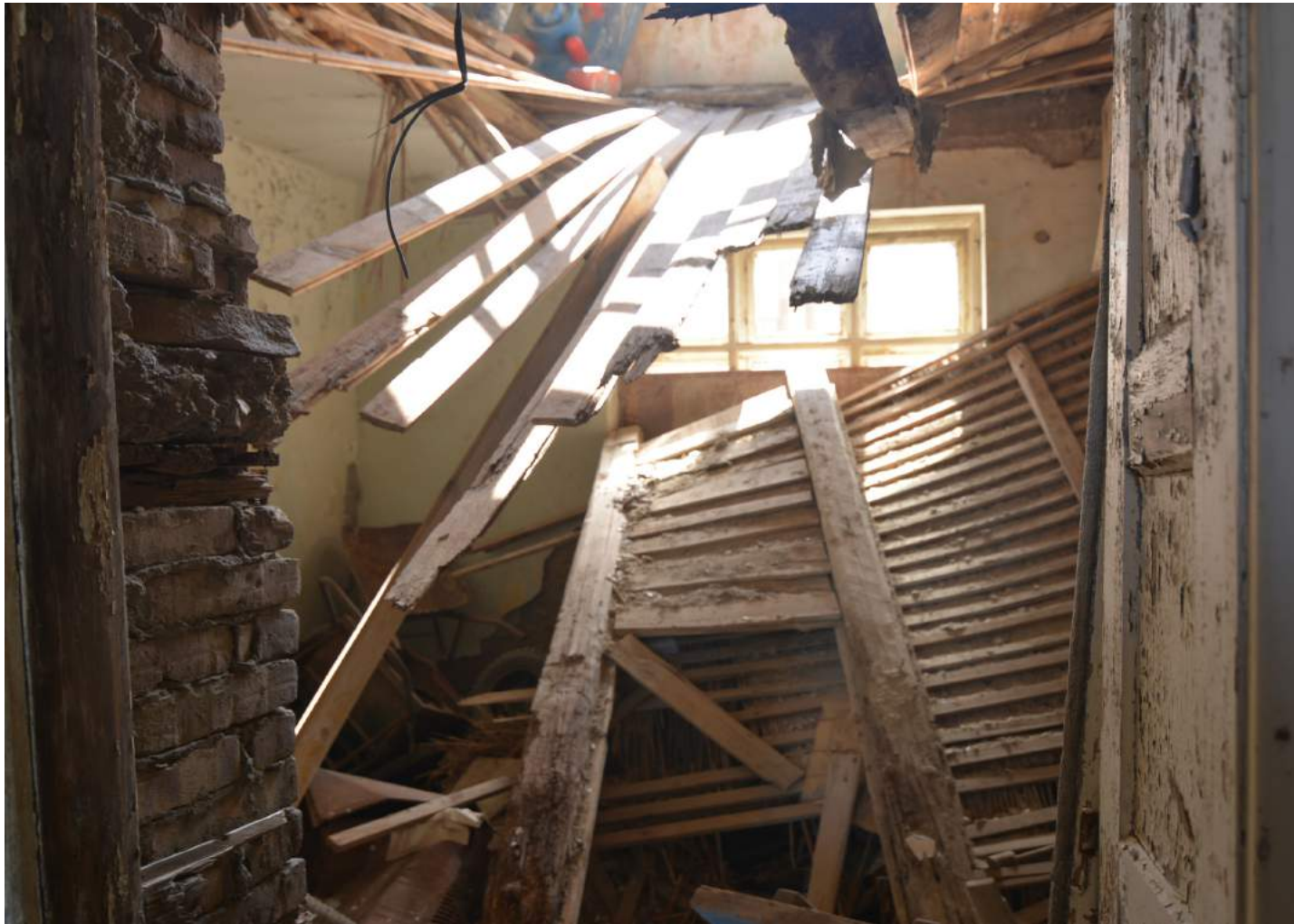
Fig.92 Current room situation
