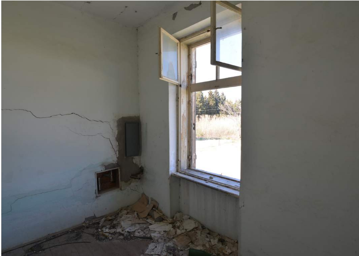
Fig.111 Current room situation
