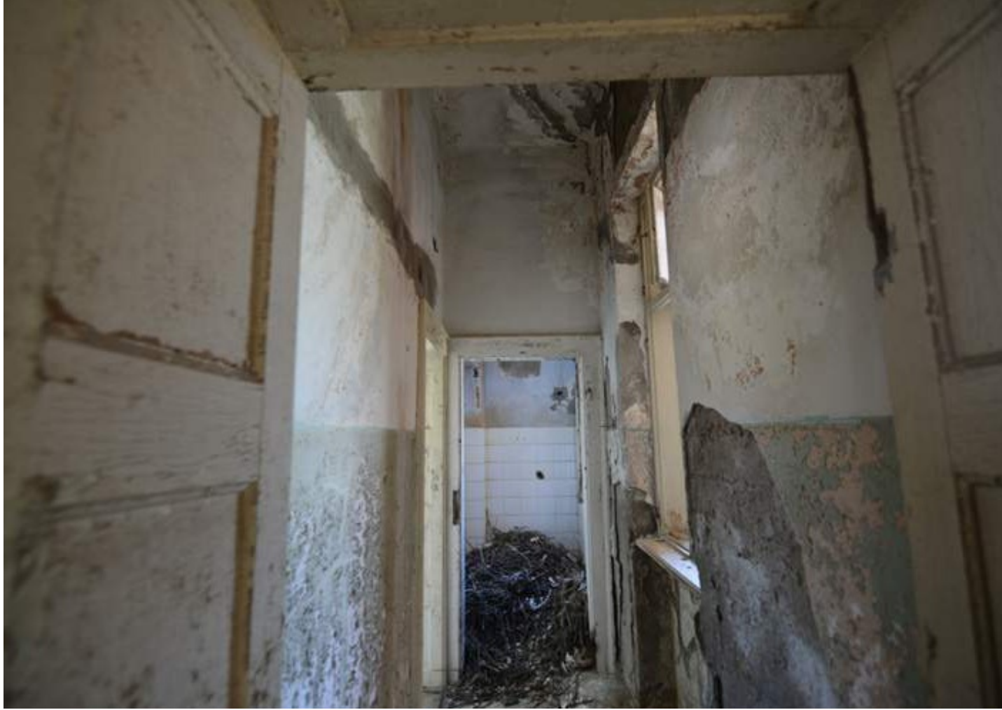
Fig.112 Current toilette situation
