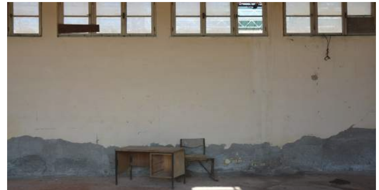
Fig.63 Inside of the Warehouse II
