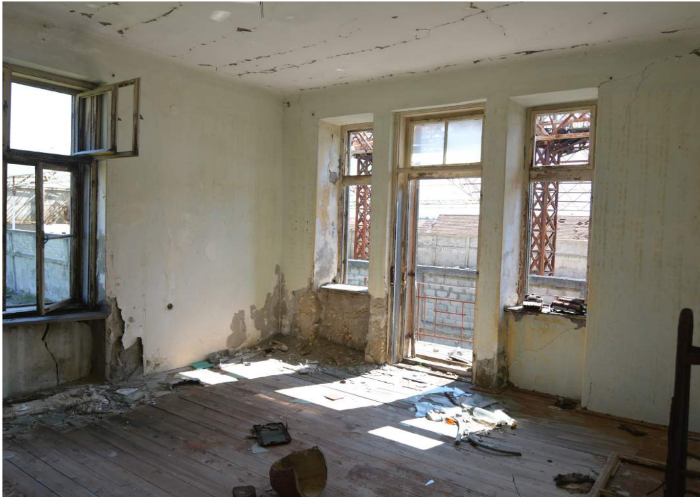
Fig.103 Current room situation
