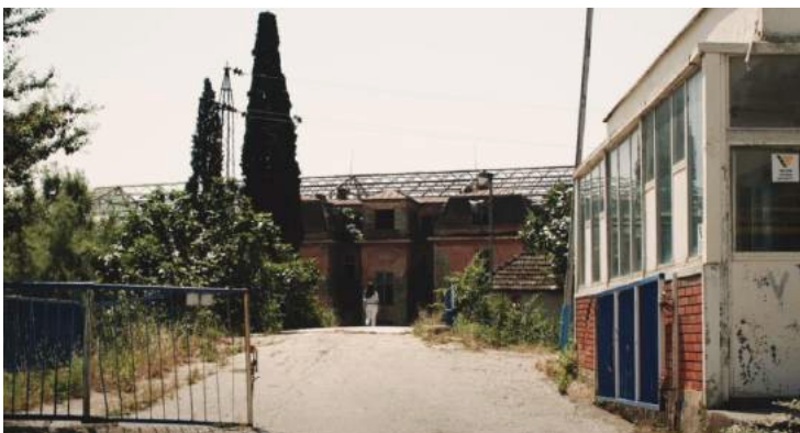
Fig.55 View from the entrance
