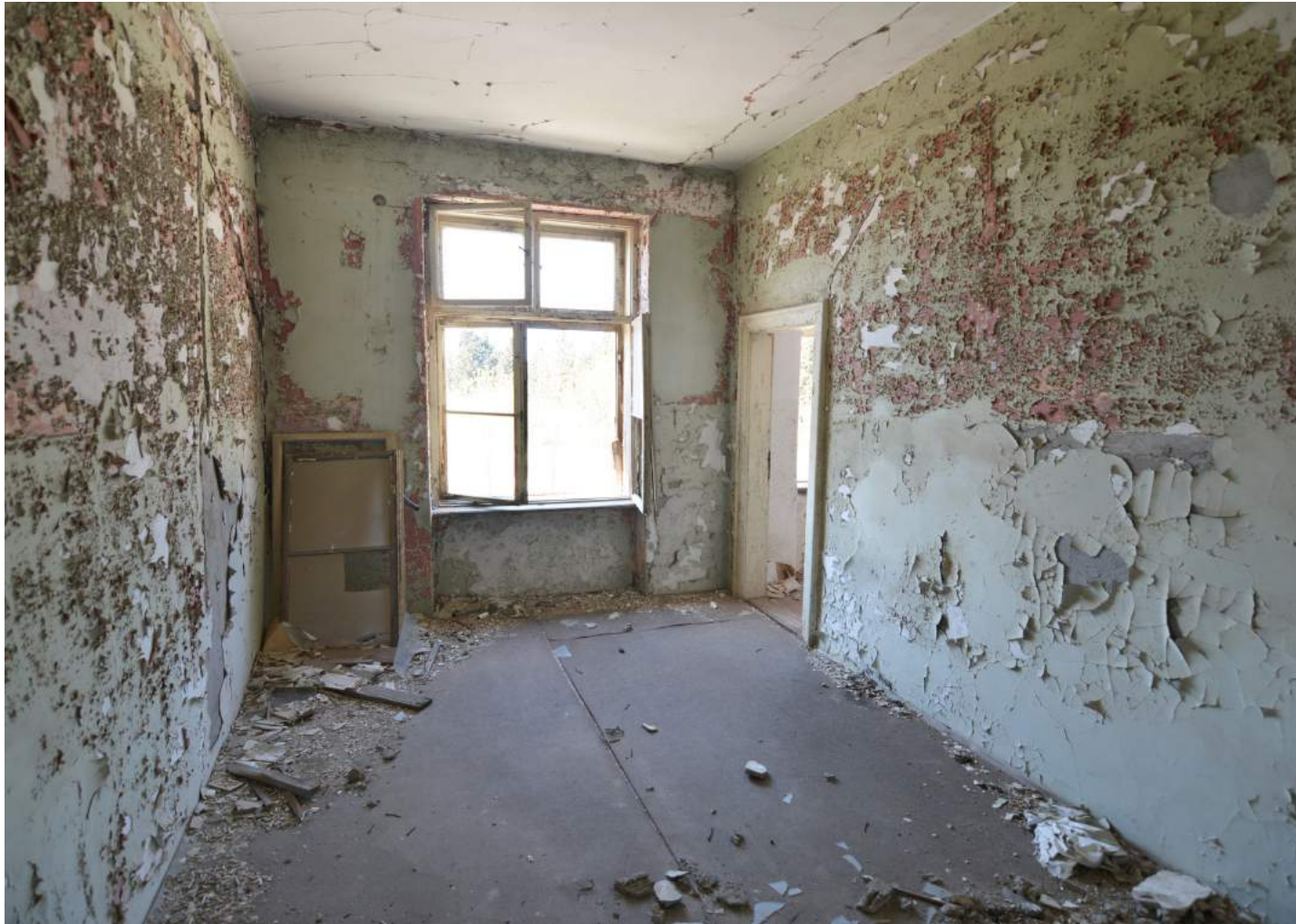
Fig.109 Current room situation
