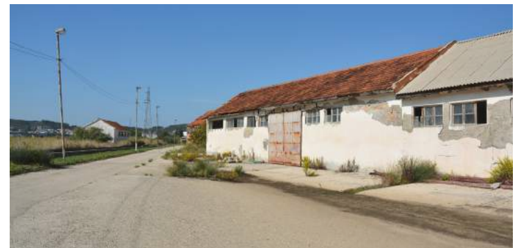
Fig.64 Warehouse II and III
