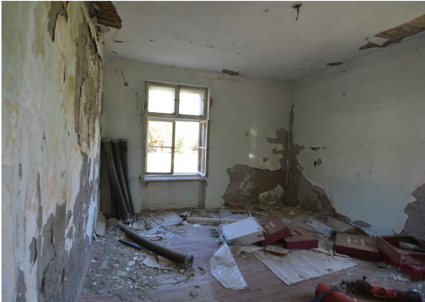
Fig.90 Current room situation
