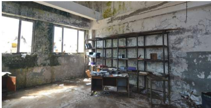
Fig.72 Air compressor station
