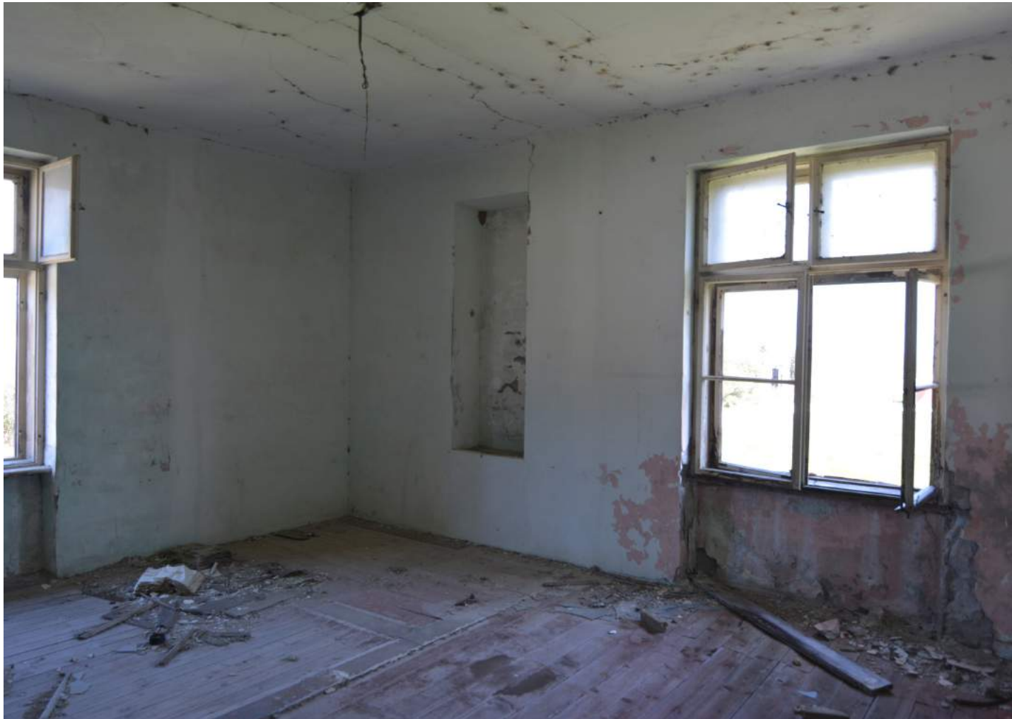
Fig.102 Current room situation
