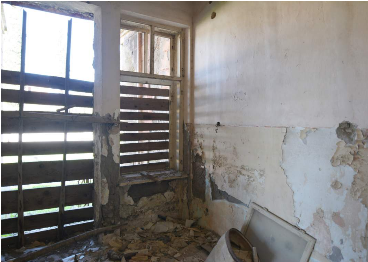
Fig.95 Current hall situation
