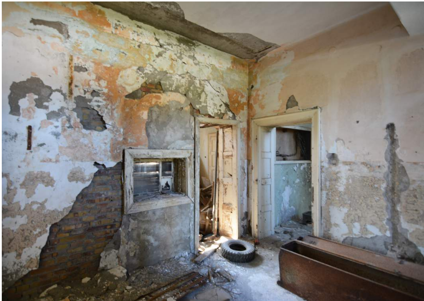
Fig.89 Current hall situation
