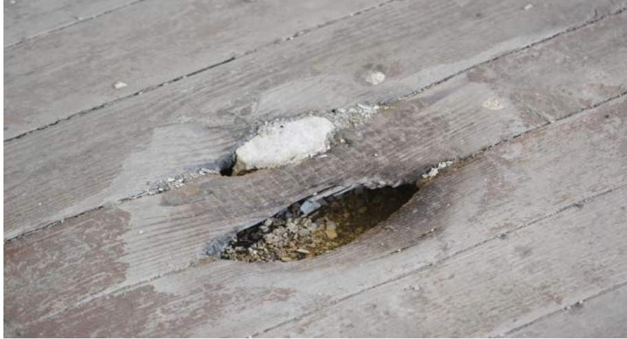
Fig.171 Floor cavity
