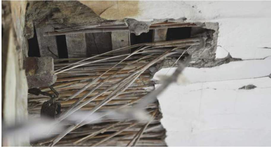
Fig.154 Exposed ceiling construction
