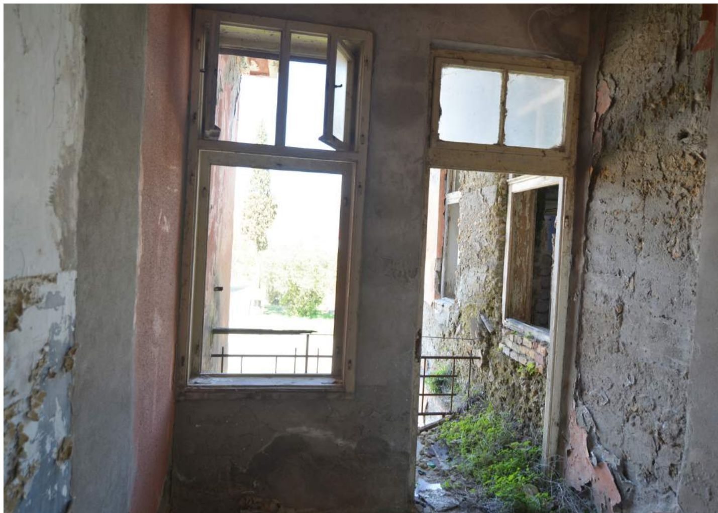
Fig.101 Current hall situation
