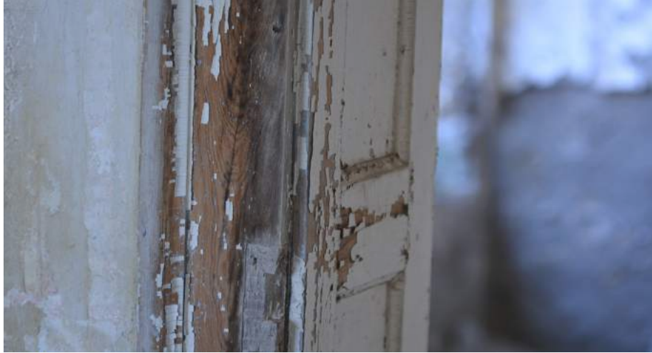
Fig.146 Wooden door detail
