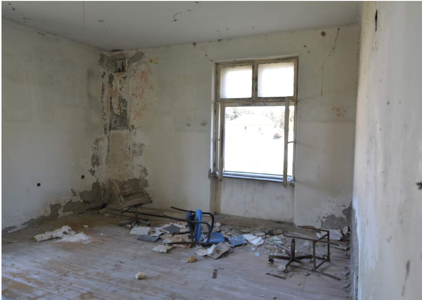
Fig.98 Current room situation
