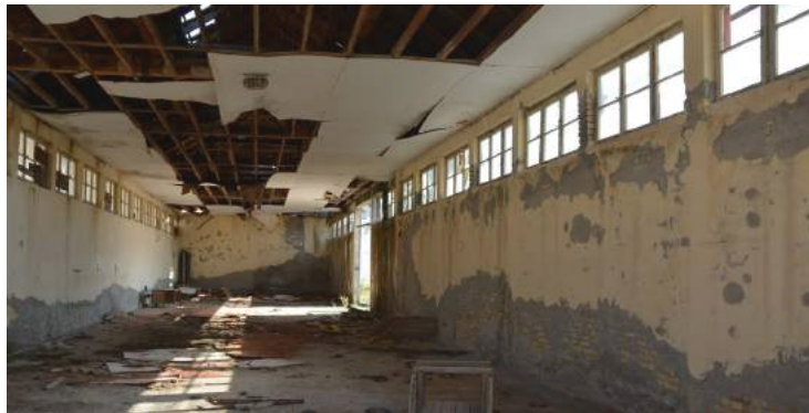
Fig.60 Inside of the Warehouse II
