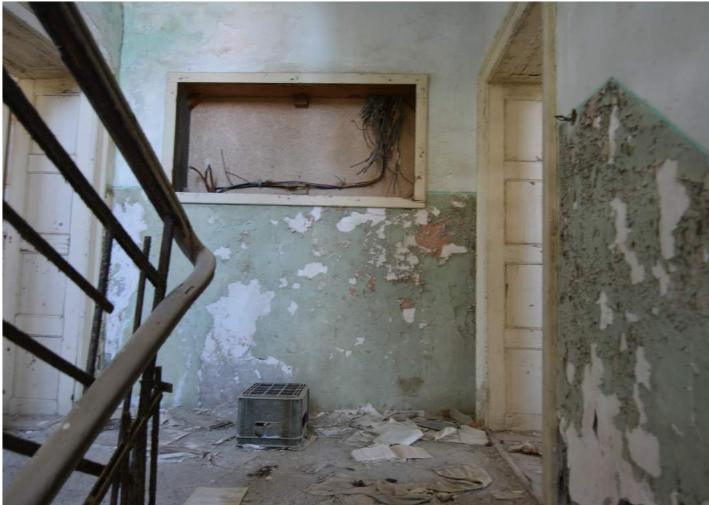
Fig.94 Current entrance hall situation
