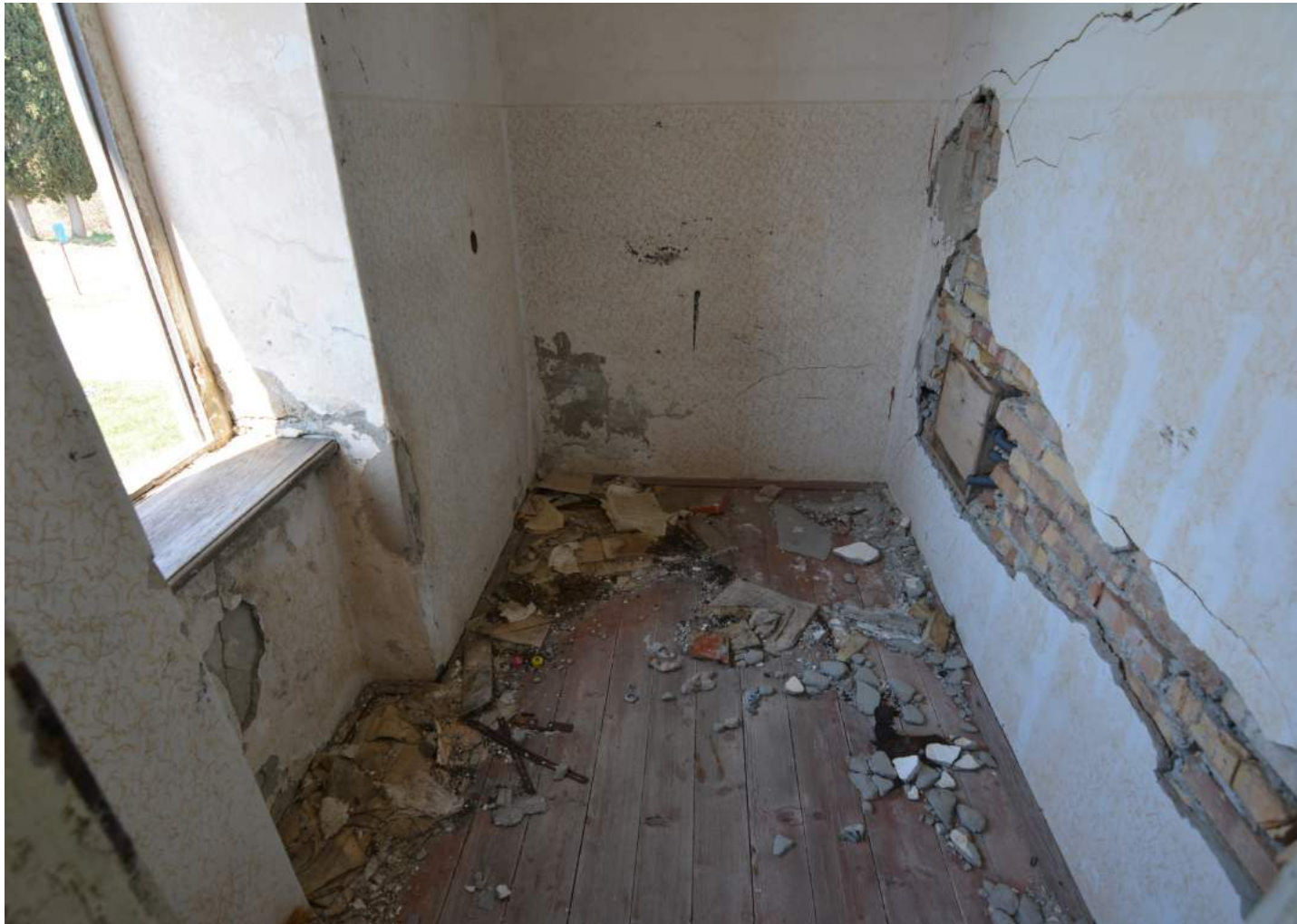
Fig.110 Current room situation
