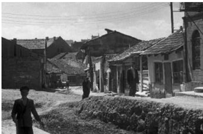
Figure 8: Demolition of the bazaar in Pristina.
