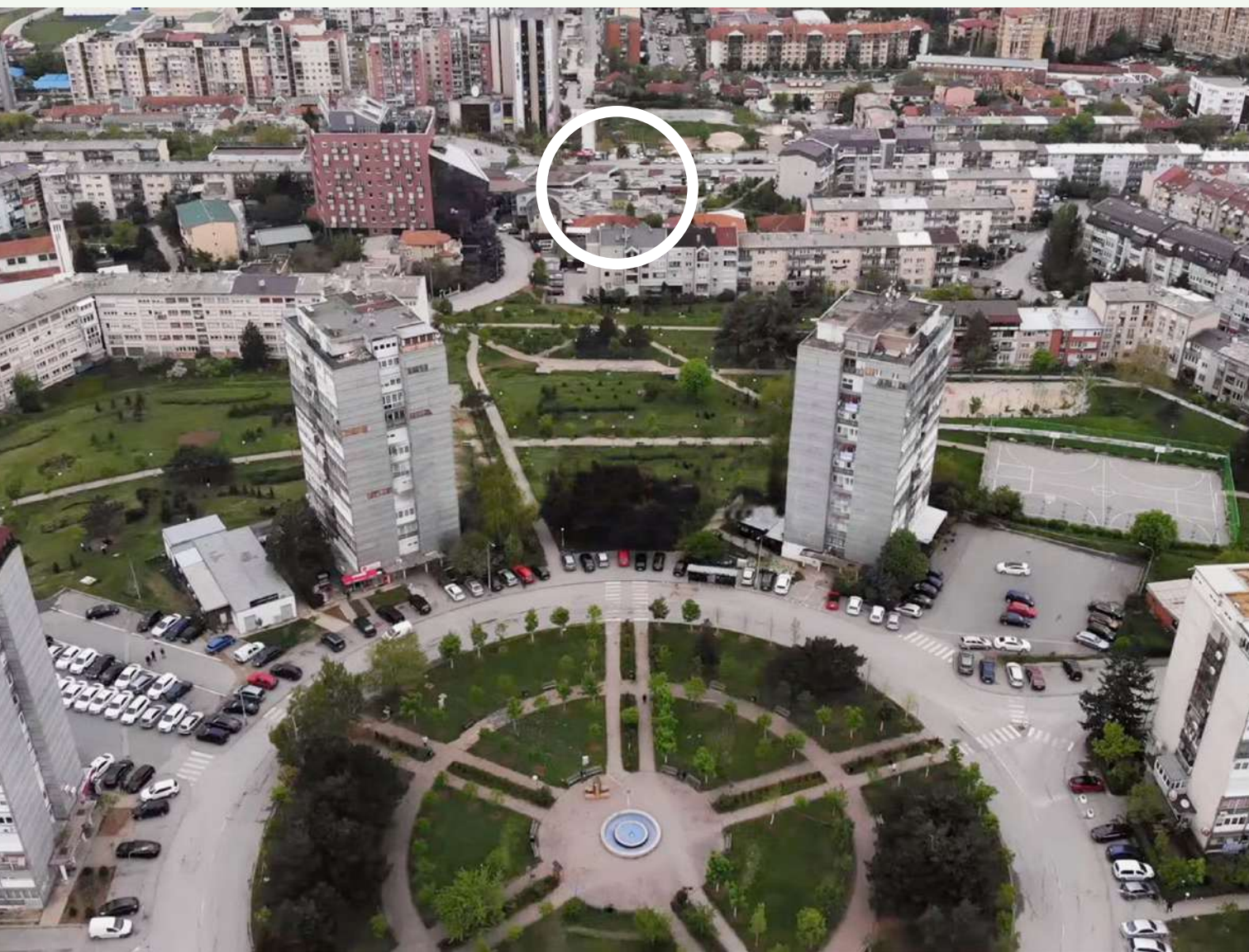
Ulpiana neighborhood and our building site
