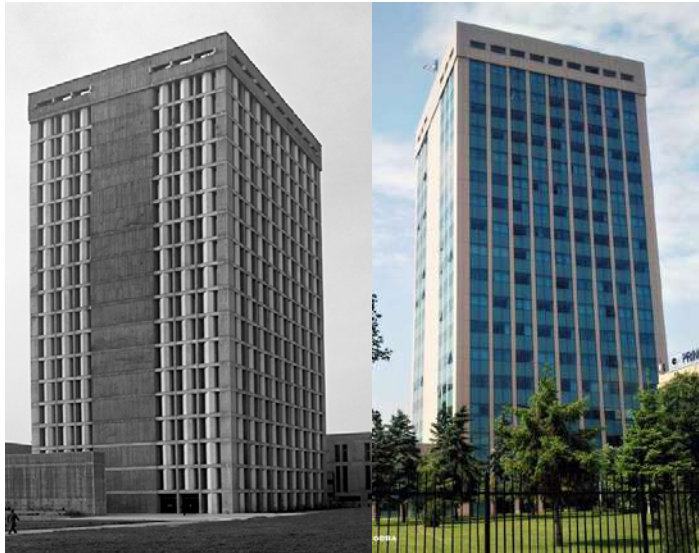
Figure 16: Rilindja Media Palace during '70s and today.
