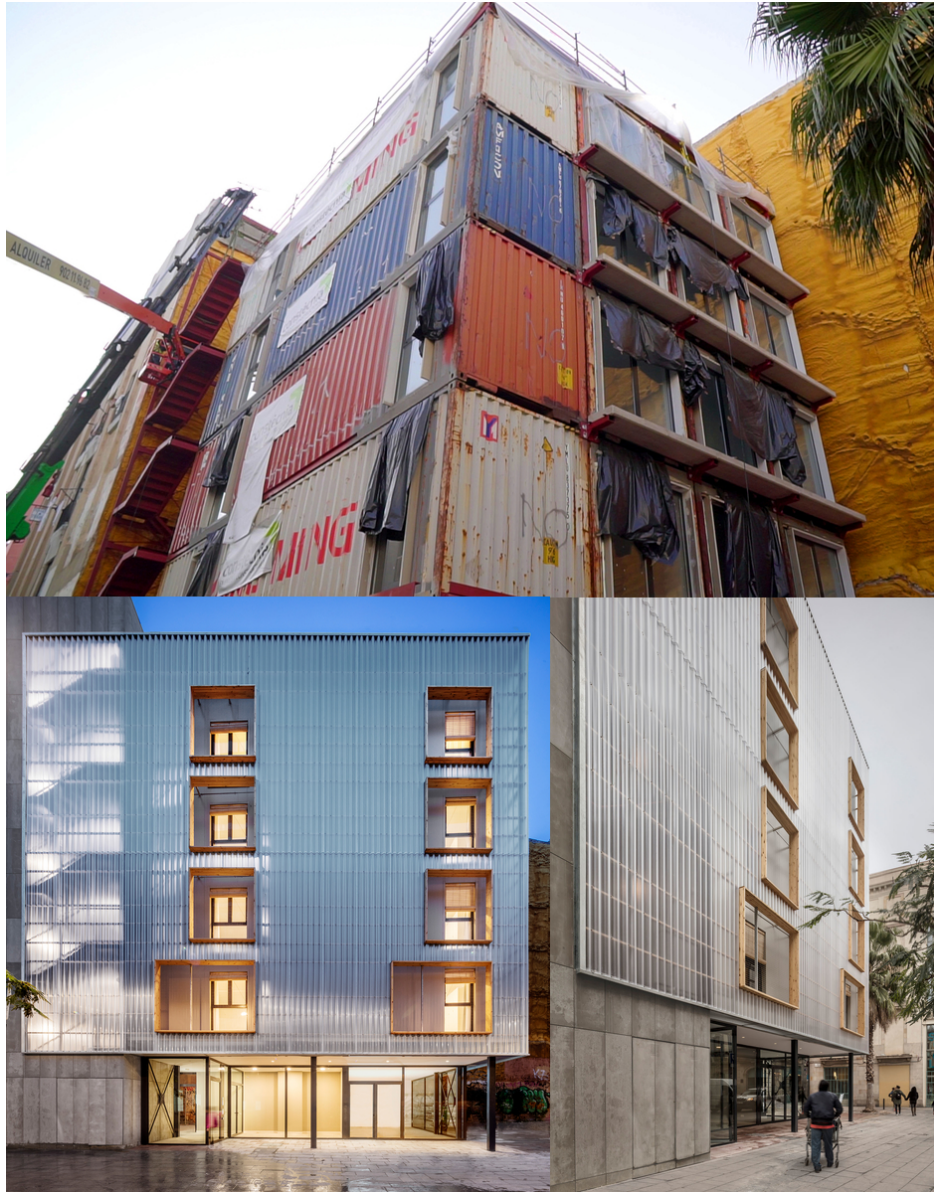
Figure 15: Office & residential building in Barcelona, Spain. Constructed from 48 modified SCs in the narrow, uneven and historic gothic quarter of the city. (Zettel 2020)
