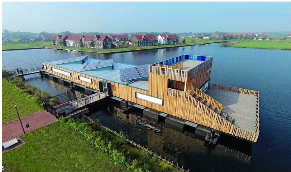
Figure 12: Offices on water in Groningen, the Netherlands. 32 modified SCs with wood cladding, a 140 panel PV system, and mobile design by ELA container. (Deutsche Bauzeitung 2017)
