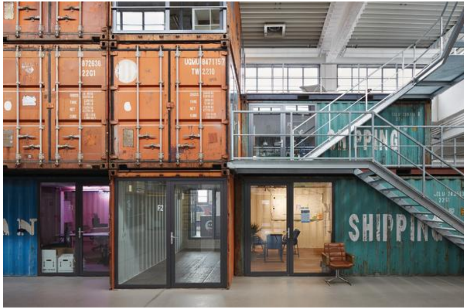
Figure 11: ‘Gründerzentrum’ in Karlsruhe, Germany. 68 modified end of life SCs within the old market hall offer affordable space for arts, design, theatre, literature, and journalism. (Deutsche Bauzeitung 2014)
