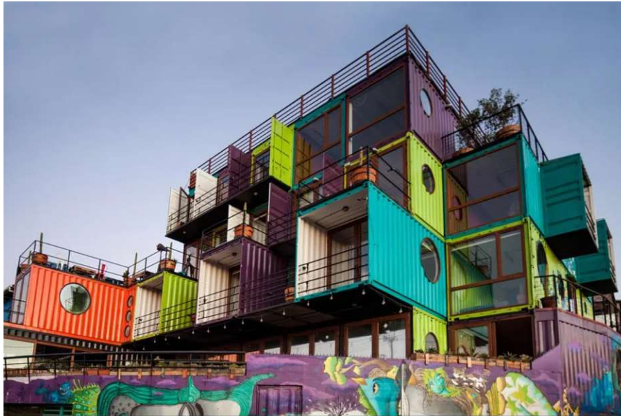
Figure 3: Hotel WineBox in Valparaiso, Chile designed by architect Camila Ulloa using 25 recycled SCs, constructed in 2017 (win 2019)
