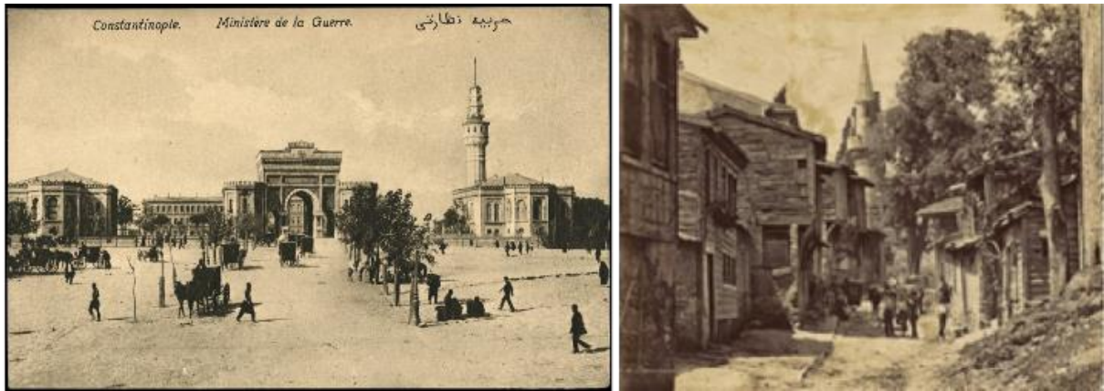
Fig. 3.4 Two contrasting images of masonry official edifices around Harbiye Nezareti (today Beyazıt Meydanı) versus a street view with wooden housing fabric in Uskudar from late 1800s; Author's archive.
