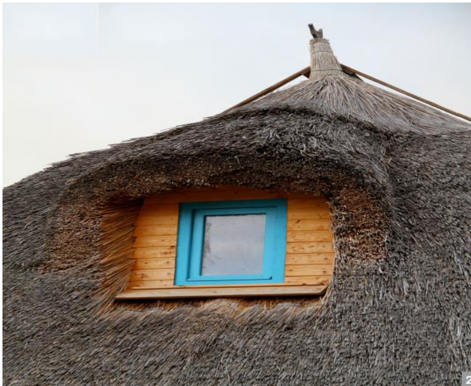
Figure 14 – Roof window (Union of Architects from Romania, 2016)
