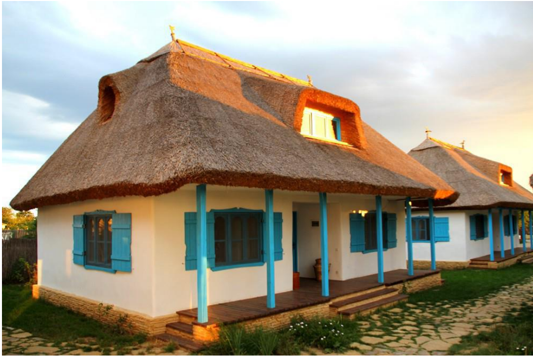
Figure 10 – Typical vernacular Danube Delta house (Union of Architects from Romania, 2016)
