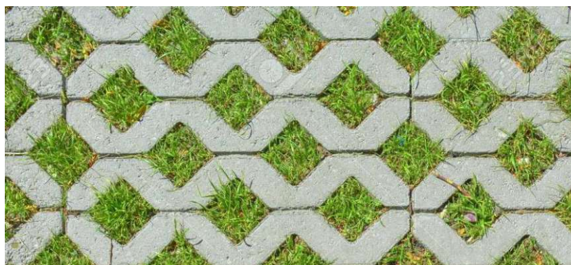
Figure 4. Grass concrete tiling grid (wikiwand, 2007)
