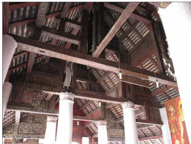
Fig. 3.39 Transverse frames of the viharn
