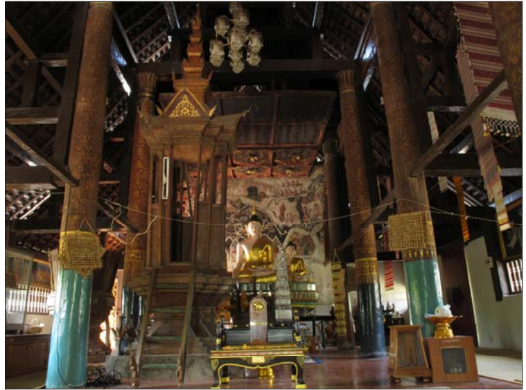
Fig. 3.77 Carpenter inserted longitudinal bracing along nave pillars
