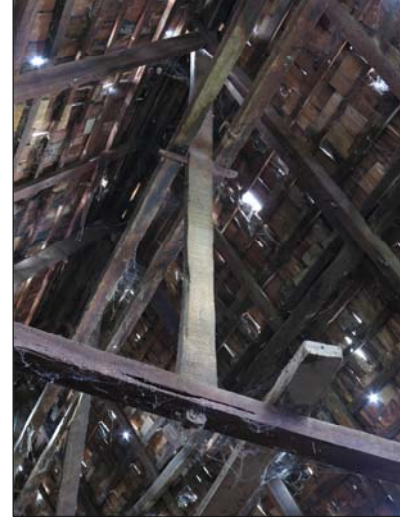
Fig. 4.18 The vertical element supporting the ridge purlin is detached from the pair of tang yo ; therefore this element behave differently from a kingpost
