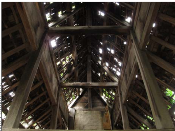
Fig. 4.22 Nave roof structure of the ubosot of Sri Auan is in deteriorate stage (surveyed in 2013)
