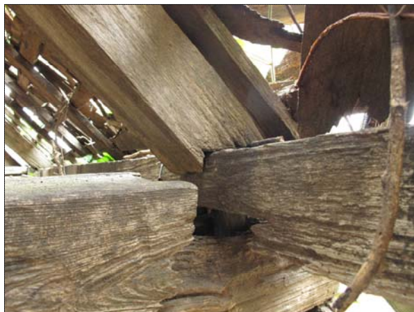
Fig. 4.23 The top edge of main purlin exceeds the surface of the main crosswise beam by 4 cm, it provides a place for bird's mouth connection of the tang yo's lower end
