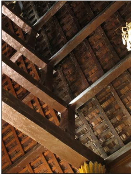
Fig. 3.76 Nave roof structure consists of four levels of crosswise beam
