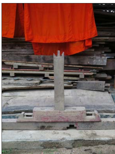
Fig. 2.7 Ridge supporting pillar presenting v-shape recessed with additional tenon
