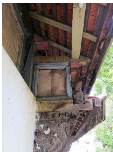
Fig. 2.4 yang sone pae , a sample from the viharn of Suchada monastery, Lampang province
