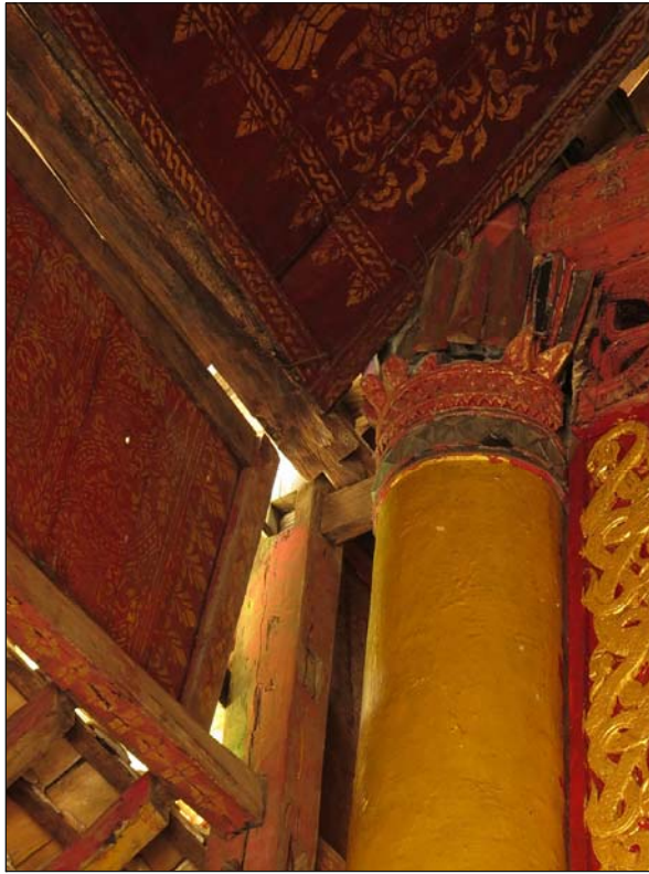
Fig. 5.37 The carpenter cut notch in recessed dovetailed bottom, sample from the viharn of Baan Kyen
