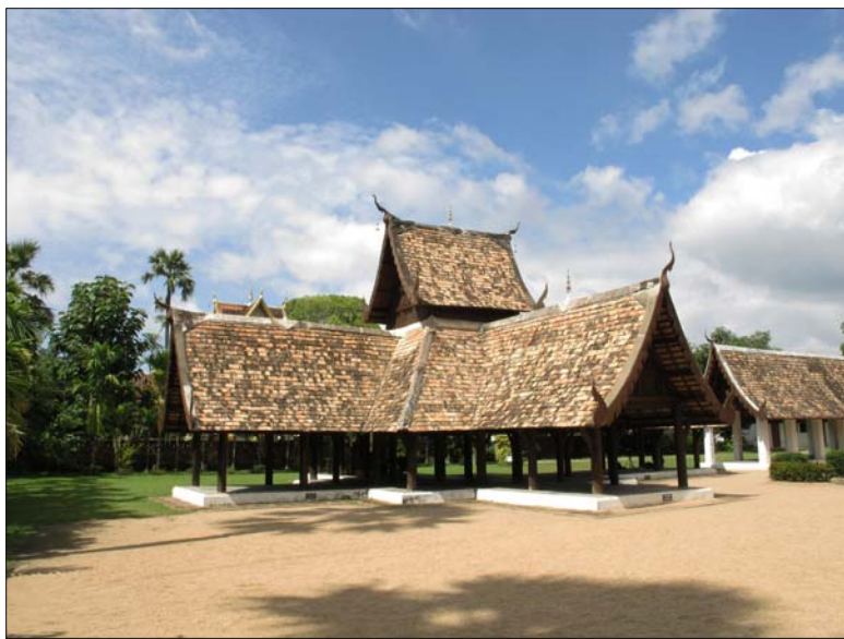
Fig. 4.42 Mandapa of Ton Kwen monastery situated on the sand open filed
