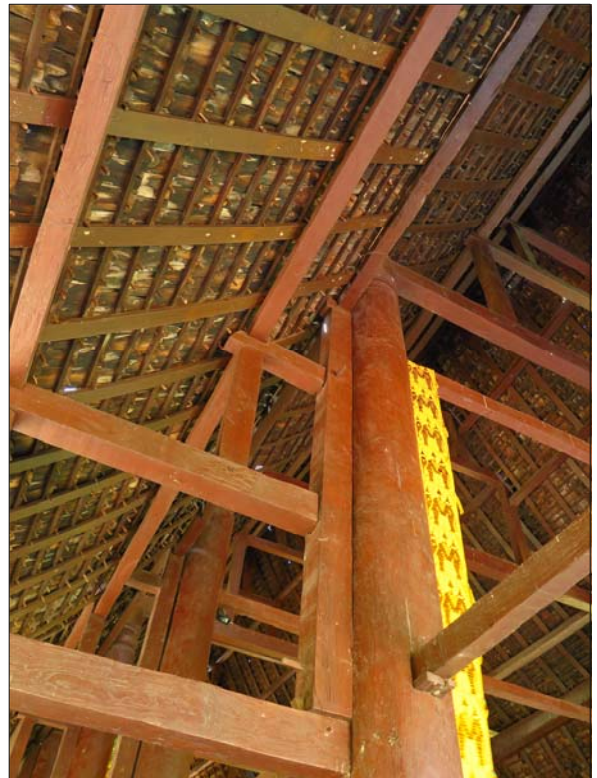
Fig. 3.81 Flanking pillar reaches until the bracket arm supporting uppermost aisle purlin; it is disassociated from the main crosswise beam
