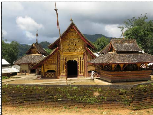
Fig. 5.14 Frontal facade of the grand viharn of Baan Saen monastery
