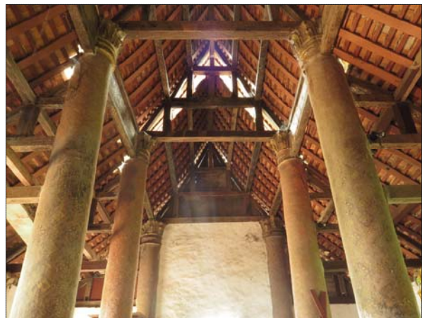
Fig. 5.7 Carpenter elevated to roof defining the principal hall
