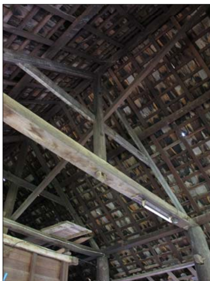
Fig. 4.13 A collar beam braced tang yo frame
