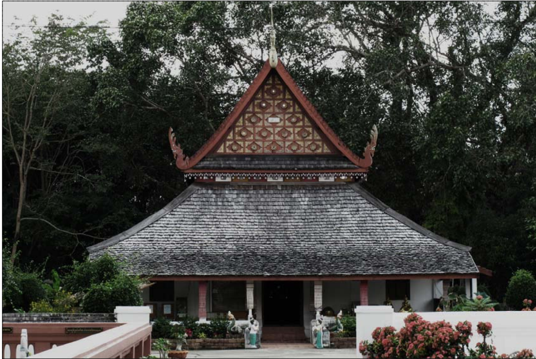
Fig. 4.2 Pediment of the viharn of Nong Daeng; we can observe a pair of tang yo assembled on each side
