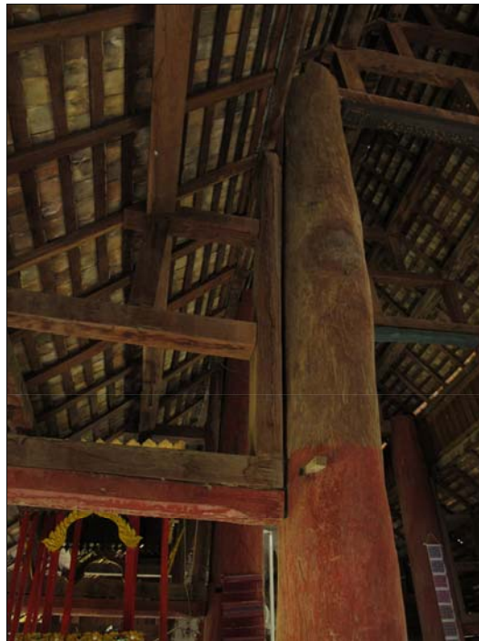
Fig. 6.4 and 6.5 Sample from the viharn of Tor Ruear monastery and viharn of Huay Rin monastery show a significant role of flanking pillar to adapt a measurement between flanking pillar and nave pillar
