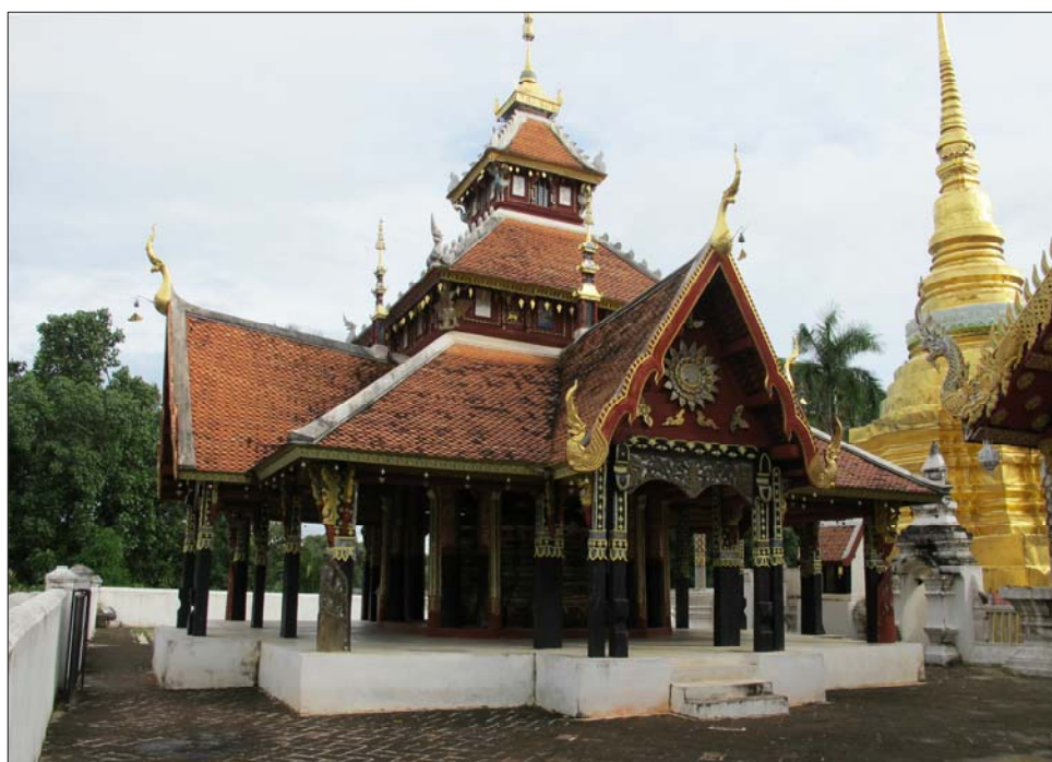
Fig. 2.2 viharn of Pong Sanuk monastery characterized by four outlying porches; Penth assumed that this building represents the mandapa type
