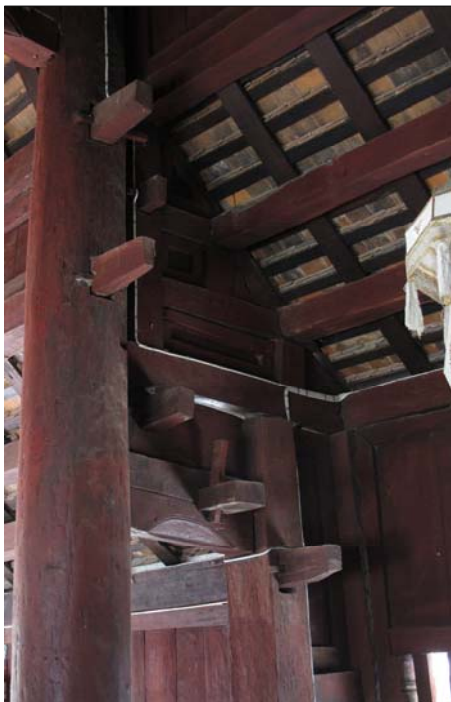
Fig. 3.61 Purlins from the first bay meeting the second transverse frame in aisle roof
