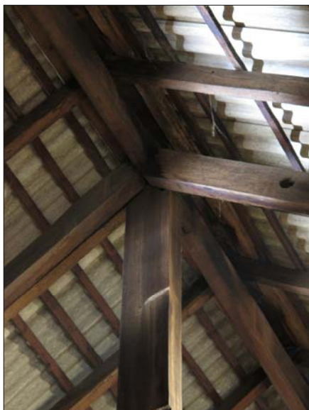
Fig. 4.47 Ridge purlin notched above tang yo and kingpost
