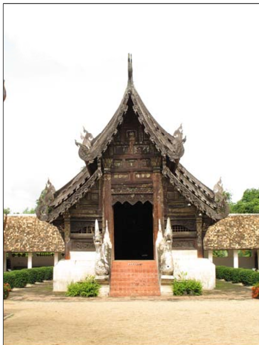
Fig. 3.53 First transverse frame at frontal facade
