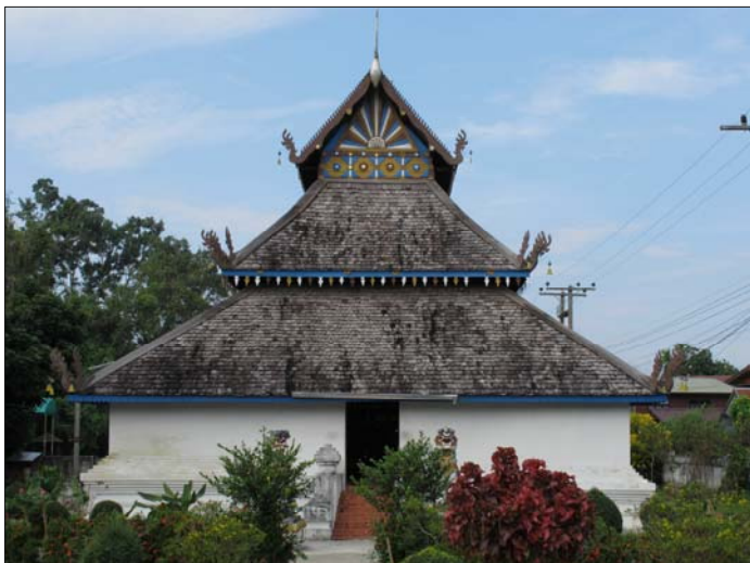
Fig. 4.7 Frontal facade of the viharn presents uppermost curved gable, upper-lower hipped roof
