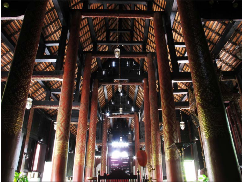
Fig. 3.70 Roof structure of the viharn of Phrasat monastery; seeing from the principal hall toward the first transverse frame at the frontal facade
