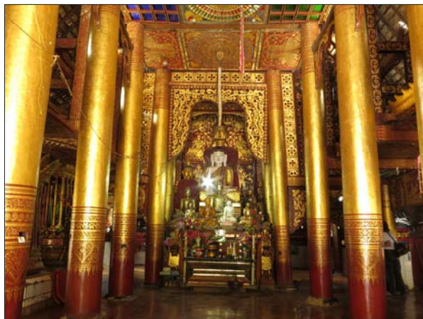
Fig. 5.15 Interior of the grand viharn; at the transverse frame in front of principal Buddha image, the carpenter infilled the gap between nave pilars and flanking pillar with decorative elements as these nave pillars moved innerward
