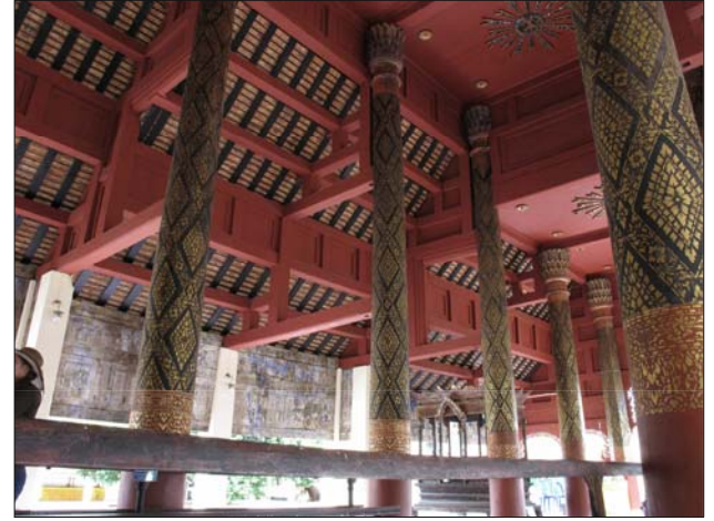
Fig. 3.23 Double layered aisle roof structure with additional neck part ( korgeeb )
