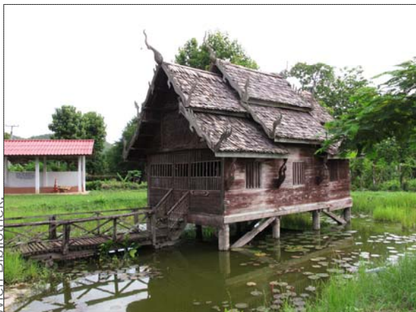
Fig. 4.25 Ubosot of Phra Bath Mae Thai was erected in the middle of the pond reflecting an idea of "water ubosot"
