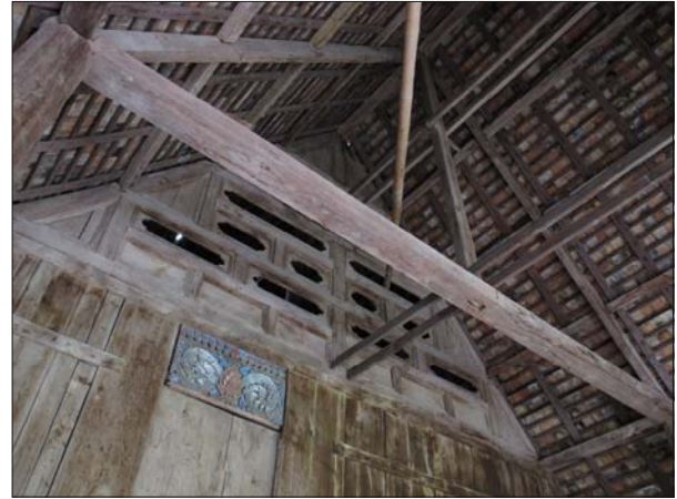
Fig. 4.32 Roof structure of the larger living unit presenting three levels of intermediate purlins
