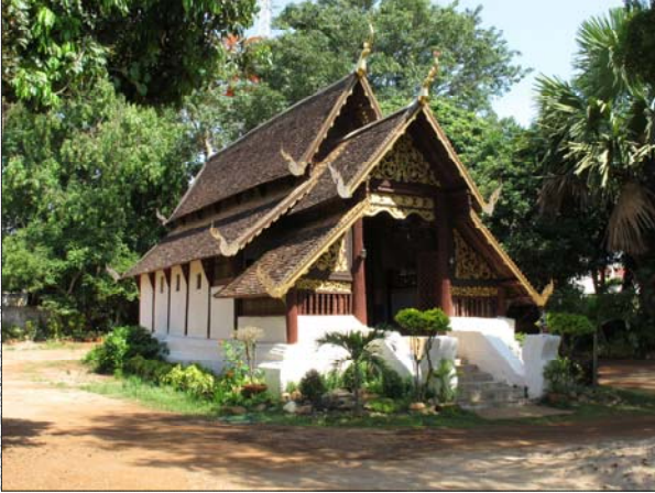
Fig. 4.36 Viharn of Klong Kak monastery; the structure of porch and principal hall are made of different structural principles
