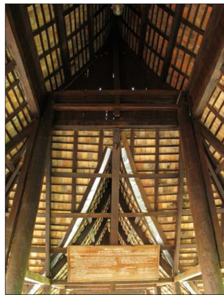
Fig. 4.43 Detail of inner ridge purlin end; the carpenter recessed ridged purlin into tenon, secured by key wedge
