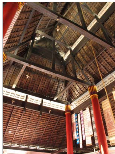
Fig. 4.8 Roof structure of the viharn; the carpenter connected first and second transverse frames by bridging beams
