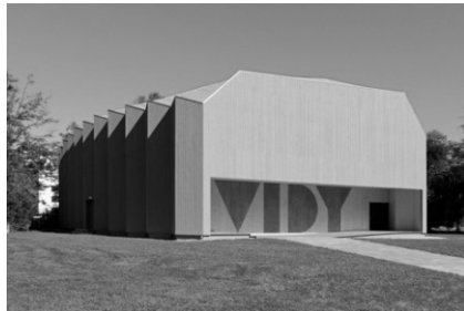
Abbildung 28: Theatersaal in Vidy
