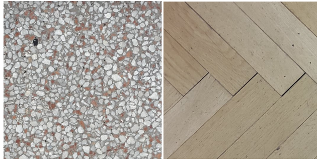
Figure 6.6: Mosaic and wooden floor structure.
