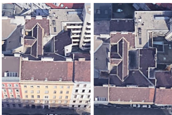
Figure 10 Fourth sample building's aerial view (source: Google Earth)
