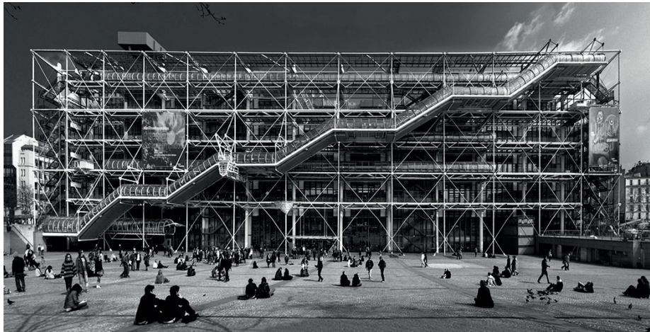
Centre Pompidou in Paris
