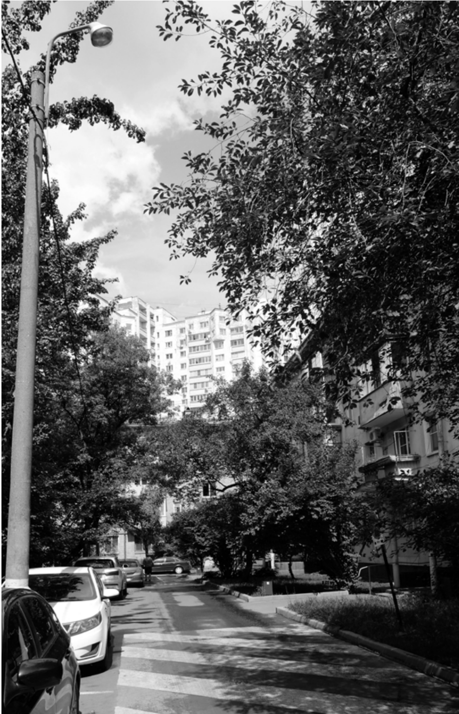
Figure 79. The experimental block in Novye Cheryomushki nowadays. The old buildings almost disappear in the luscious green. In the background stands a much higher and denser development from the Luzhkov Program. Moscow, July 2018
