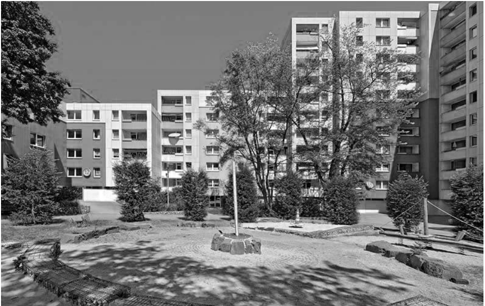
Figure 120. (top) Renovated and modernized residential complex in Clarenberg
