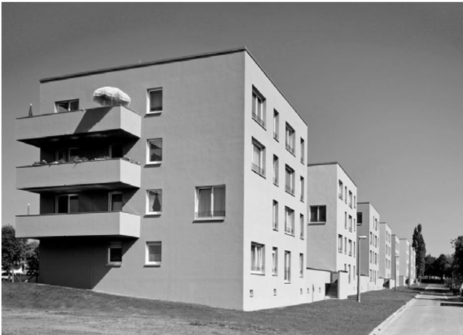
Figure 137. Leinefelde Haus 7 before and after the renovation: This could possibly be the most prominent and radical approach to the transformation of industrial mass housing. The original 180 m long apartment building lost one story and was then split into 8 detached "City Villas" connected by a shared ground floor
