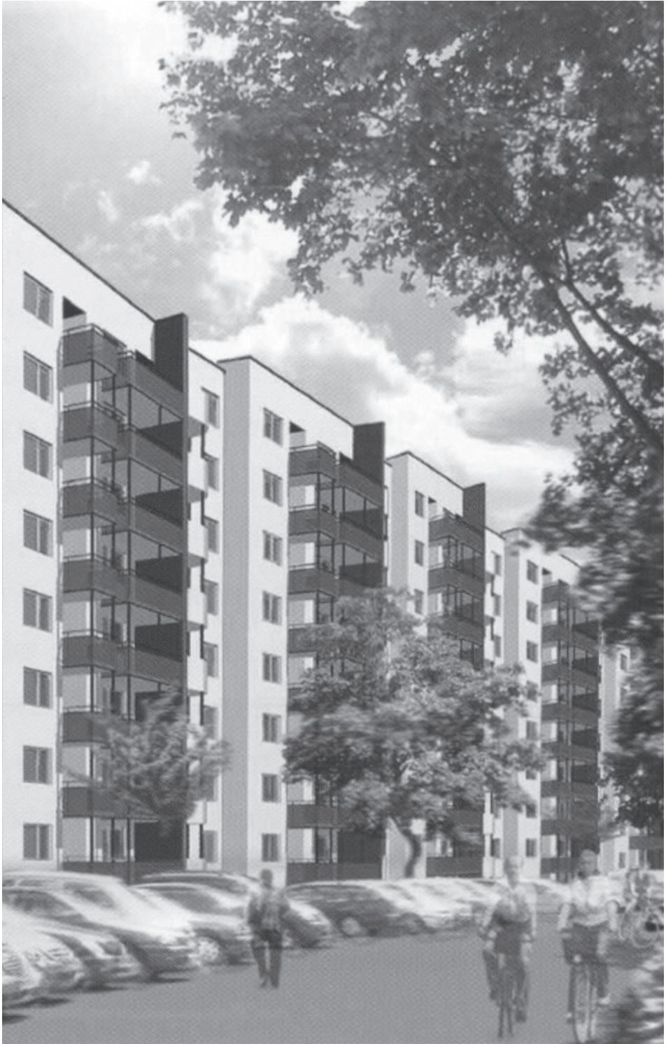
Figure 125. Architectural modernization concept is a part of the holistic concept for the renovation of Mümmelmannsberg
