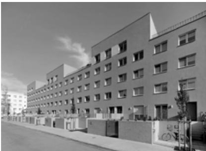
Figure 136. Leinefelde Haus 1 (1999): This reconstruction put a start to the transformation process in the commune Leinefelde in Germany. The brick wall running along two adjacent buildings forming an "L" serves a few purposes: it forms a base of the building and separates the private areas from the street.
