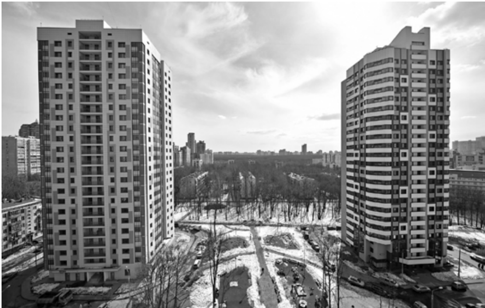
Figure 98. (top) House transferred to the Renovation Program on the Gzhatskaya Street
