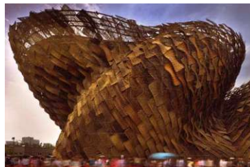
Figure 185: H5 - Expo 2010 Spain Pavilion (Shanghai) hall
