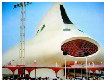
Figure 175: F7 - Expo 1970 Gas Corporate Pavilion (Osaka)
