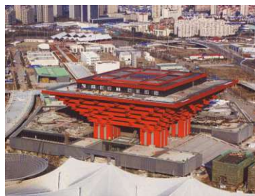
Figure 55: E2 - Expo 2010 China Host Pavilion (Shanghai) Aerial
