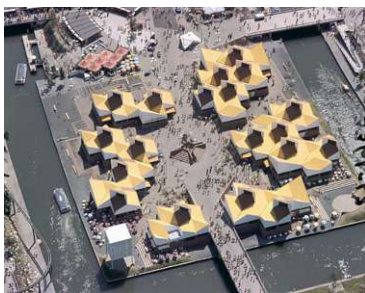
Figure 45: D2 - Expo 1967 Africa Group Pavilion (Montreal) “gaps”
