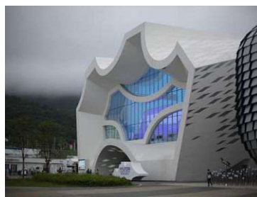
Figure 315: G2 - Expo 2012 Hyundai Corp. Pavilion (Yeosu)
