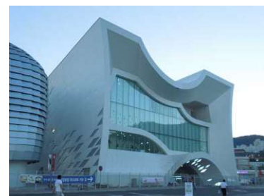
Figure 316: G2 - Expo 2012 Hyundai Corp. Pavilion (Yeosu)
