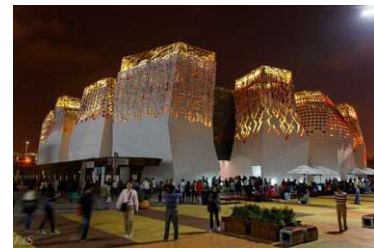
Figure 219: A4 - Expo 2010 Russia Pavilion (Shanghai) Pedestrian View Night
