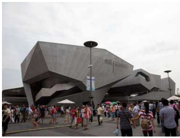
Figure 239: Pedestrian Front View. This is the view most visitors will encounter.
