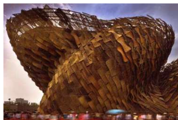
Figure 172: H5 - Expo 2010 Spain Pavilion (Shanghai)
