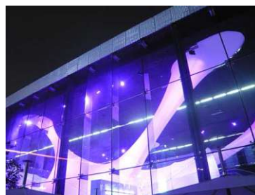
Figure 80: transparency with glass; inside is a textile structure; Expo 2010 Belgium Pavilion (Shanghai)
