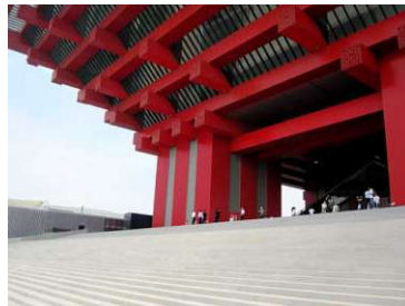
Figure 271: Entrance View 1 E2 - Expo 2010 China Host Pavilion (Shanghai)
