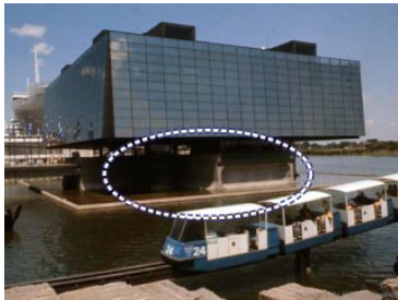
Figure 342: E6 - Expo 1967 Quebec Region Pavilion (Montreal)
