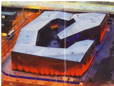
Figure 236: A1 - Expo 2010 Canada Pavilion (Shanghai)
