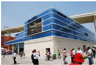
Figure 274: C4 - Expo 2010 Monaco Pavilion (Shanghai)
