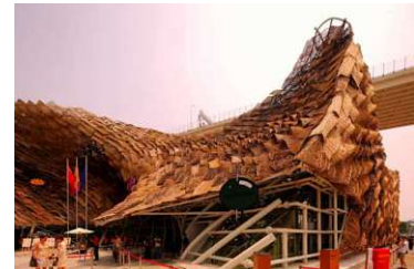
Figure 186: H5 - Expo 2010 Spain Pavilion (Shanghai) court entrance
