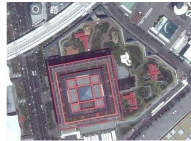
Figure 269: Aerial 2 E2 - Expo 2010 China Host Pavilion (Shanghai)
