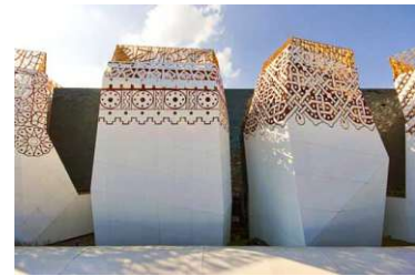
Figure 215: A4 - Expo 2010 Russia Pavilion (Shanghai) Details View
