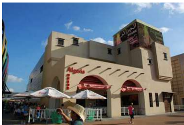
Figure 280: C2 - Expo 2010 Algeria Pavilion (Shanghai)
