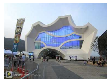
Figure 313: G2 - Expo 2012 Hyundai Corp. Pavilion (Yeosu)
