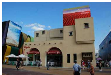
Figure 331: C2 - Expo 2010 Algeria Pavilion (Shanghai)
