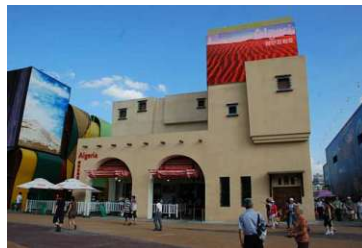
Figure 281: C2 - Expo 2010 Algeria Pavilion (Shanghai)
