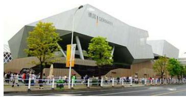
Figure 52: A2 - Expo 2010 Germany Pavilion (Shanghai) Pedestrian Back View
