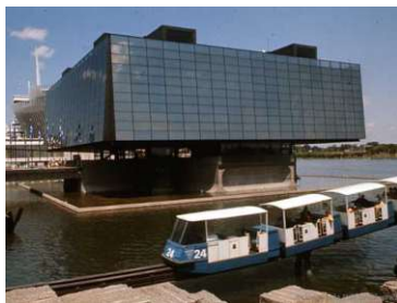
Figure 258: E6 - Expo 1967 Quebec Region Pavilion (Montreal)
