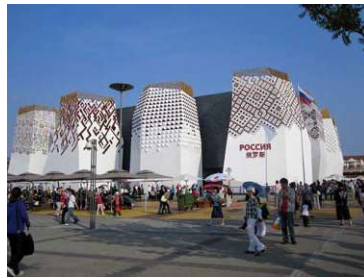
Figure 214: A4 - Expo 2010 Russia Pavilion (Shanghai) Pedestrian View
