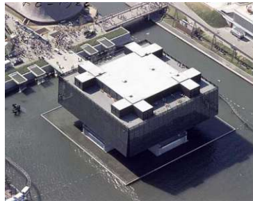
Figure 259: E6 - Expo 1967 Quebec Region Pavilion (Montreal)
