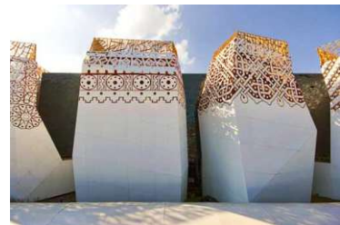
Figure 18: A4 - Expo 2010 Russia Pavilion (Shanghai) Details View
