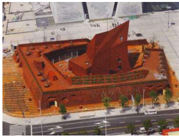
Figure 193: Aerial View B5 - Expo 2010 Luxembourg Pavilion (Shanghai)
