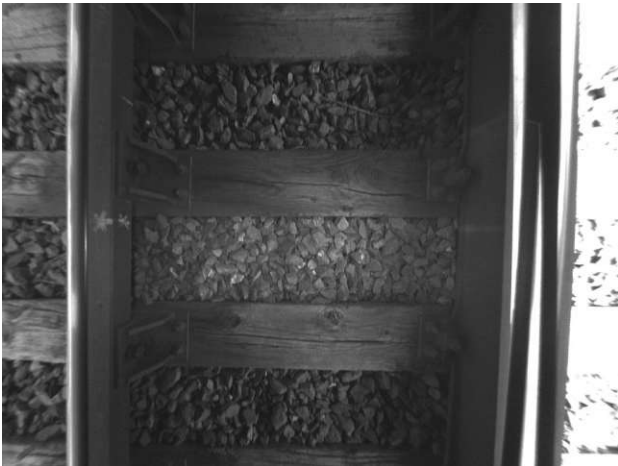
(e) At the center of a switch between two tracks is a so-called switch frog.
