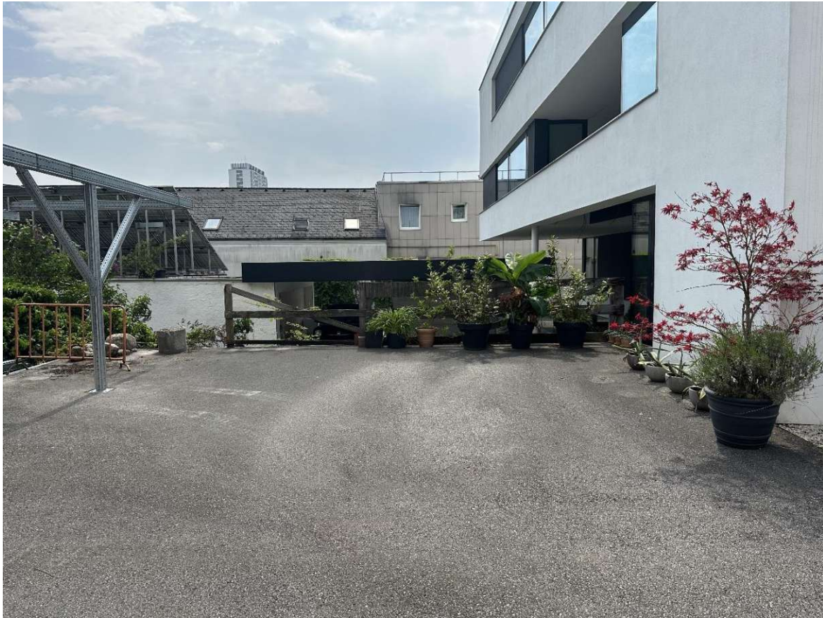
Figure 89: P3 - Space between building and shed. On the left already built parts of the shed are seen.
