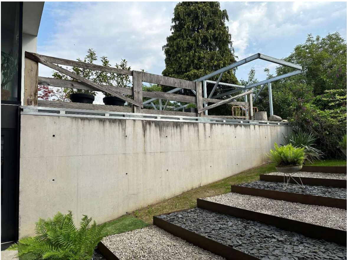
Figure 91: P5 - change in terrain. The picture is taken from basement-level.
