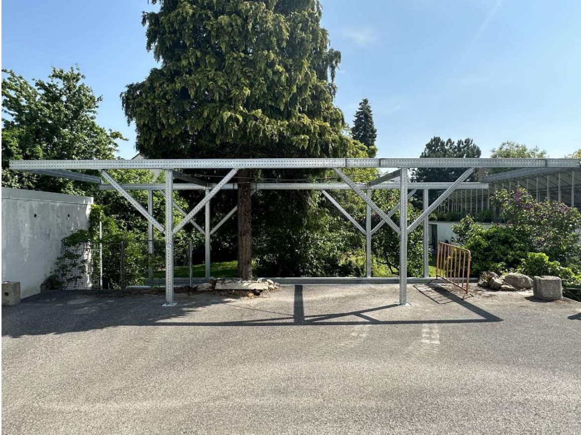
Figure 135: Already built parts of the structure as testing begins
