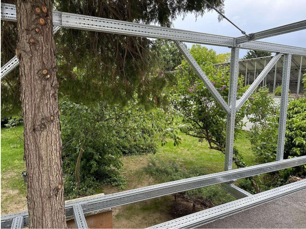
Figure 93: P7 - Sight from driveway down into the garden.
