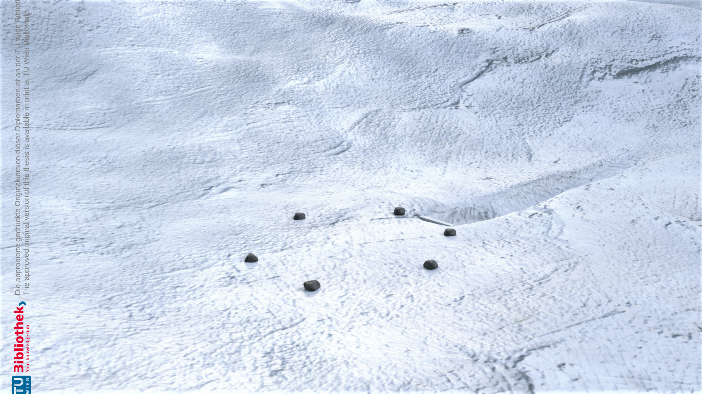
Step 1: excavating the ramp and positioning the footing stones
