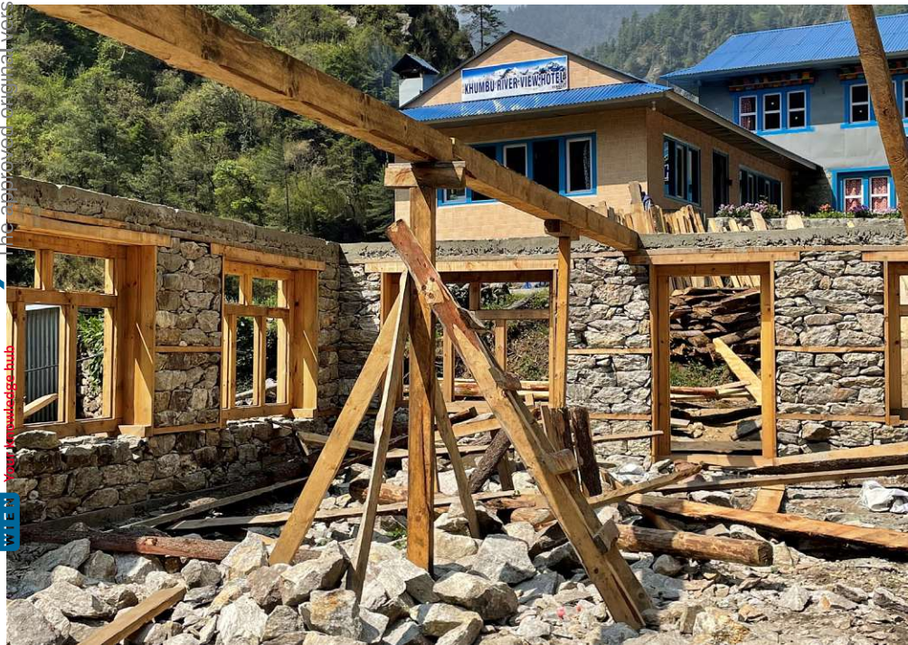
Fig. 17: Rack for building the ceiling
