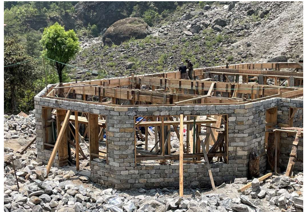
Fig. 16: Construction site near Phakding
