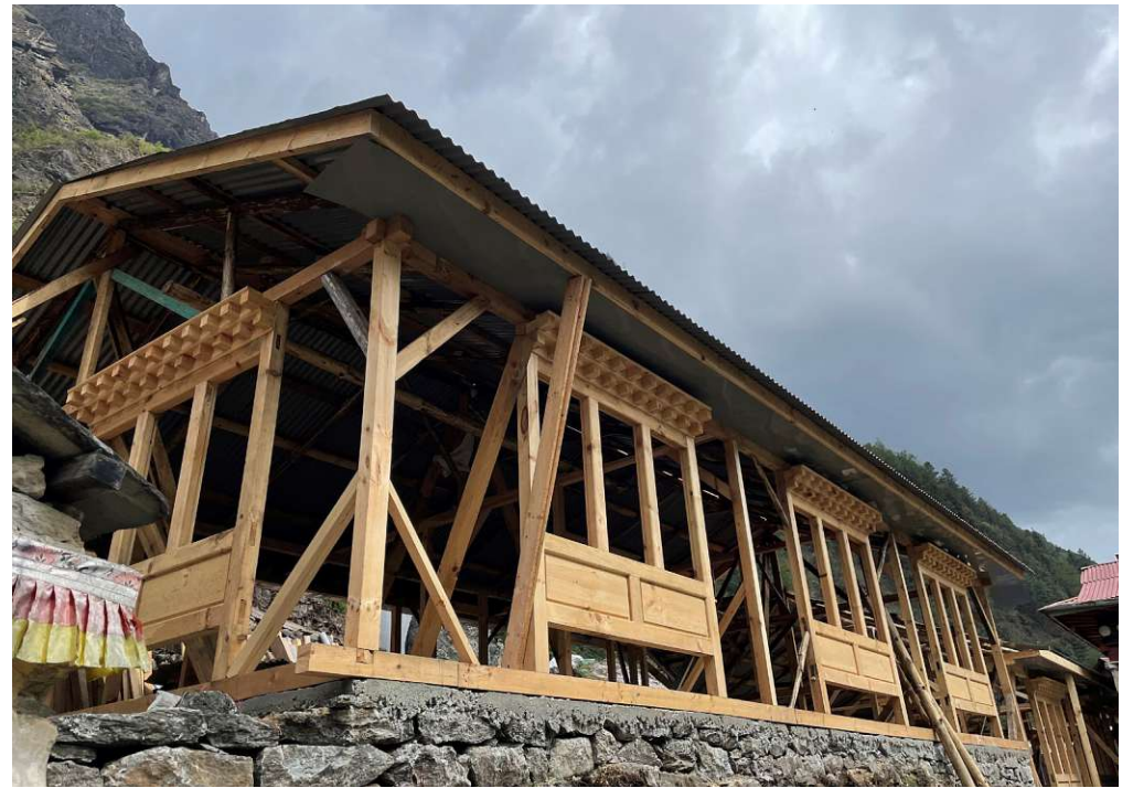
Fig. 12: Construction Site Phakding
