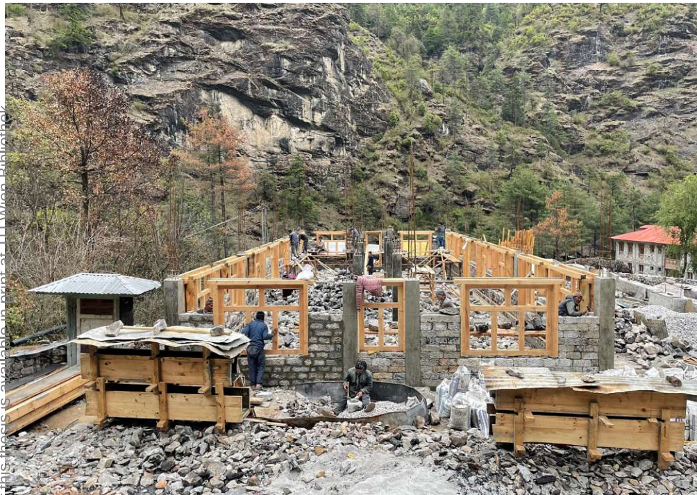
Fig. 15: Construction of a ground floor
