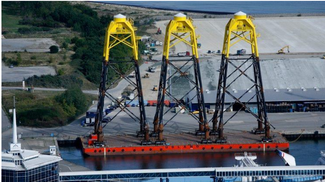
Figure 12 Jacket foundations for offshore wind turbine. Retrieved from (CORPORATIVA n.d.)
