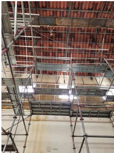
fig.91 inside the church
