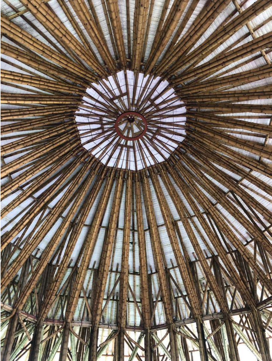
fig.115 roof construction from the inside, Zeri Pavillon
