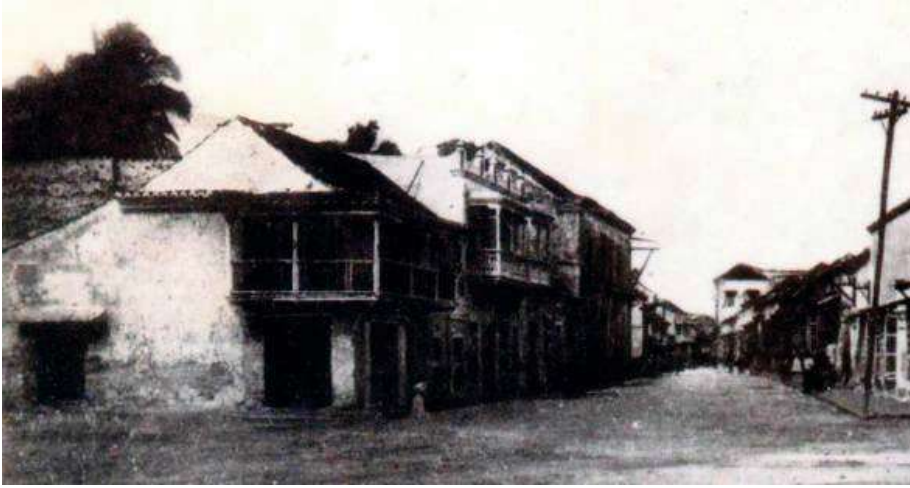
fig.161 first traditional colonial buildings, Bolivar
