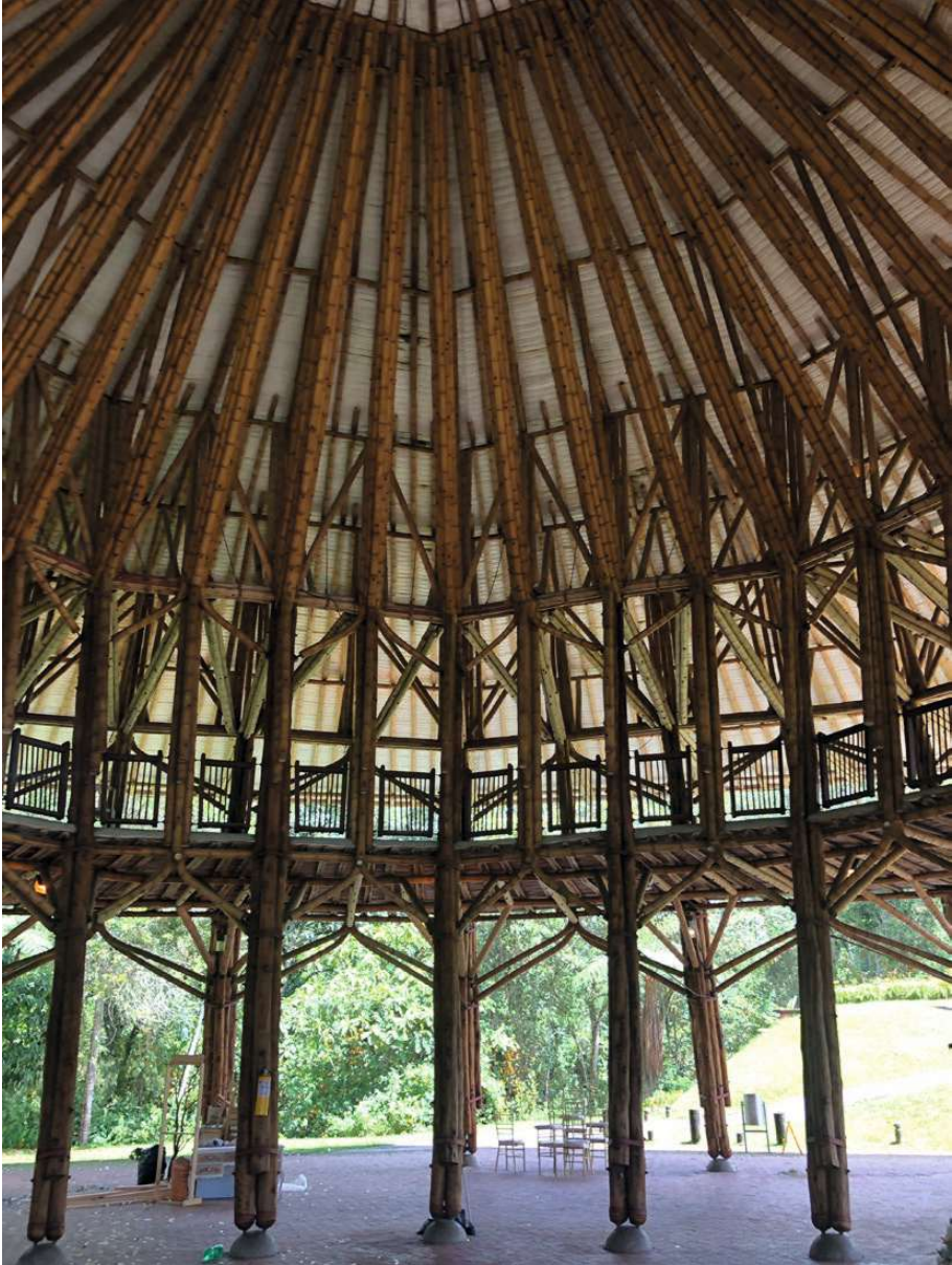
fig.116 guadua and wood structure, Zeri Pavillon
