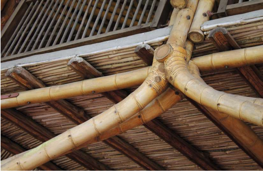
fig.119 and fig.120 connections between the guadua pieces, Zeri Pavillon
