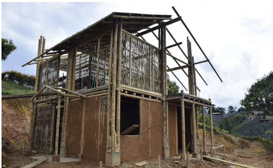
fig.77 the construction with some ground floor walls already covered with clay.
