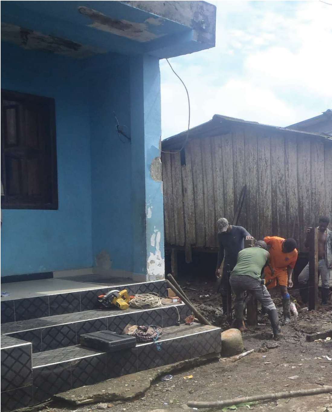
fig.142 building construction, El Valle
