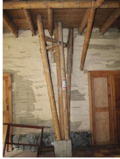
fig.59 concrete base made with guadua framework
