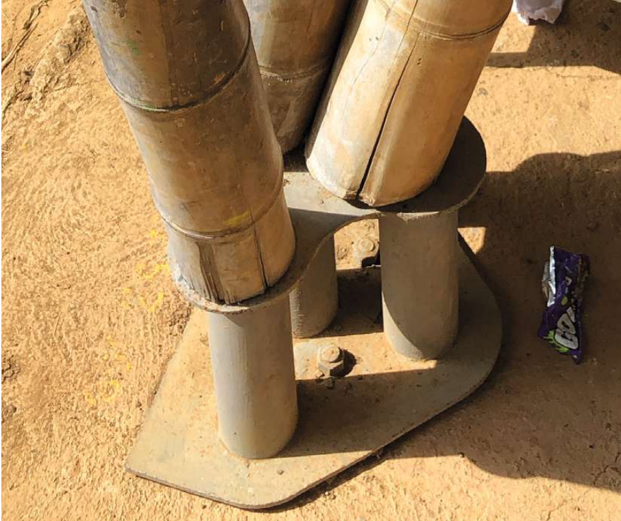
fig.57 base for guadua structure, Montebello
