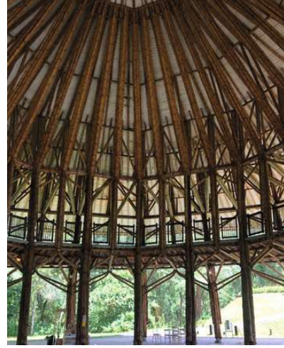
fig.232 guadua structure, Zeri Pavillon
