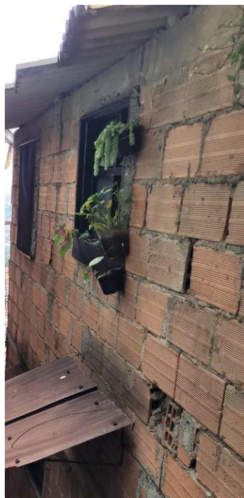
fig.38 ladrillos, self-built invasiones
