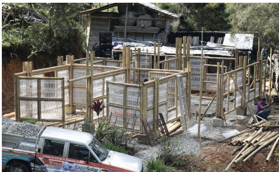
fig.83 most of the frames are built and already filled with plastic bottles
