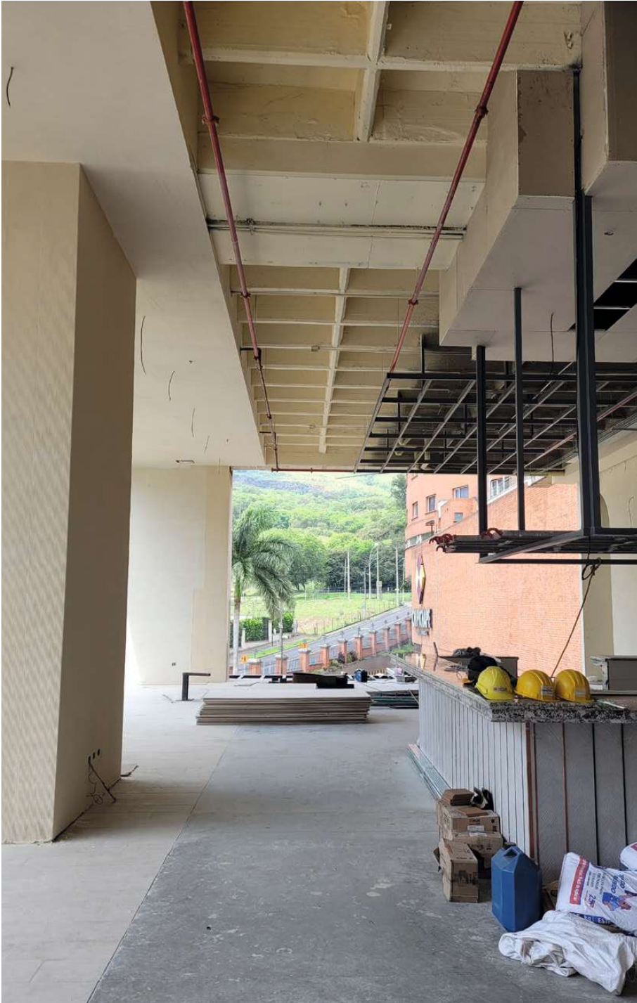
fig.88 inside view of the restaurant under renovation, with the open walls
