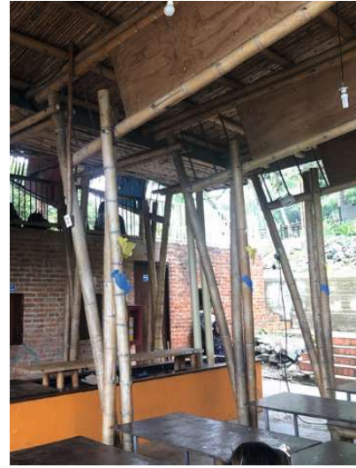
fig.67 the structure holding the roof
