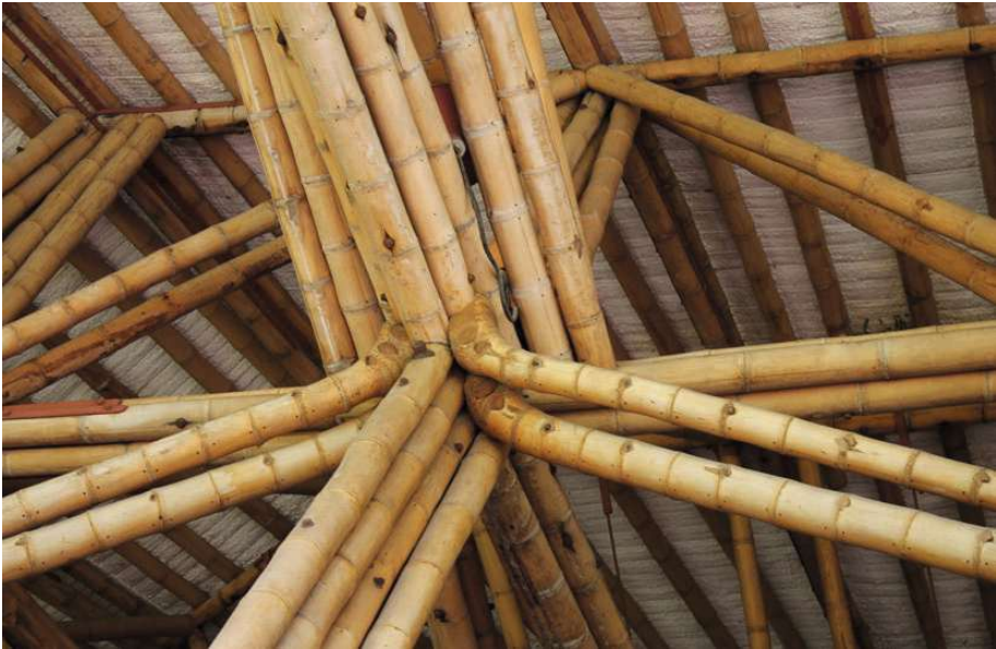
fig.119 and fig.120 connections between the guadua pieces, Zeri Pavillon
