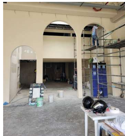
fig.87 inside room of the restaurant
