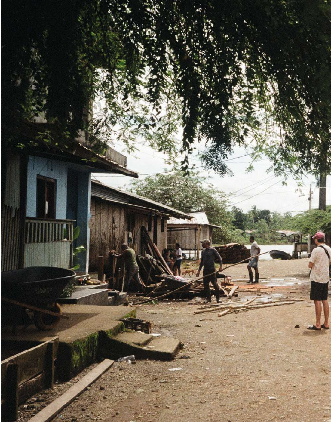
fig.144 building construction, El Valle
