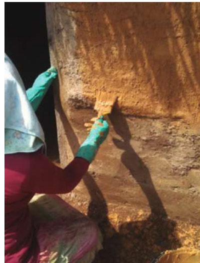
fig.155 refinement layer, bahareque technique
