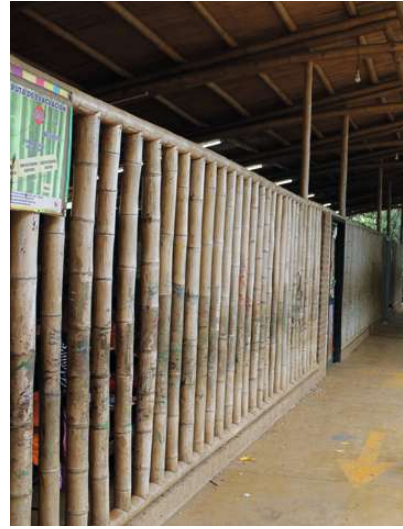
fig.71 dividing walls to the classes
