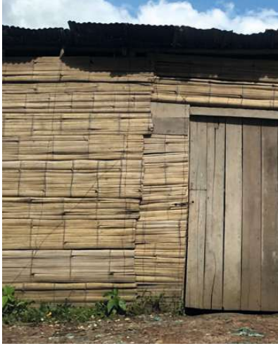
fig.231 guadua esterilla walls, Eje Cafetero
