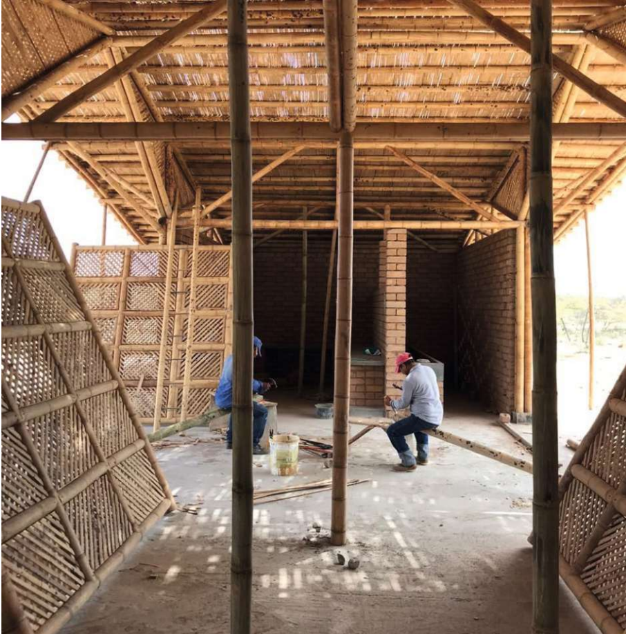
fig.191 carpenters working on the guadua structure, Walirumana
