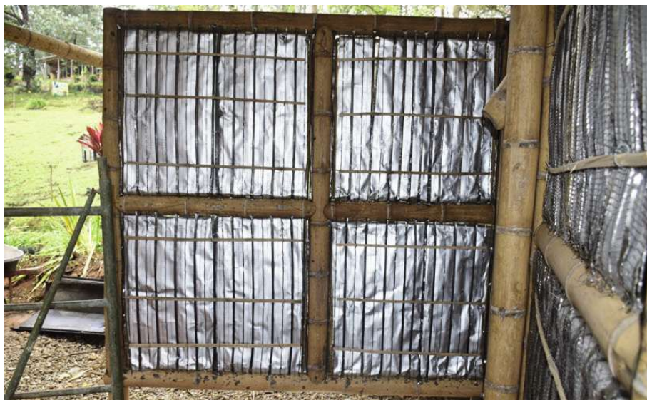
fig.84 The plastic bottles are covered with aluminum and a metallic net.
