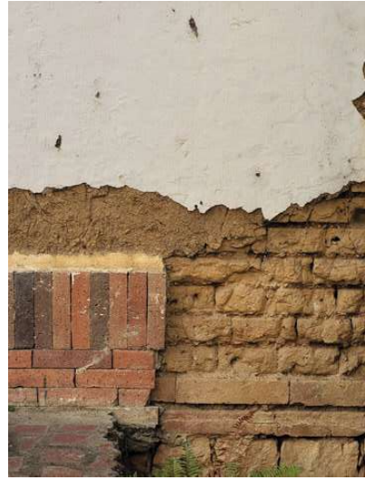
fig.90 constructing materials outside the church
