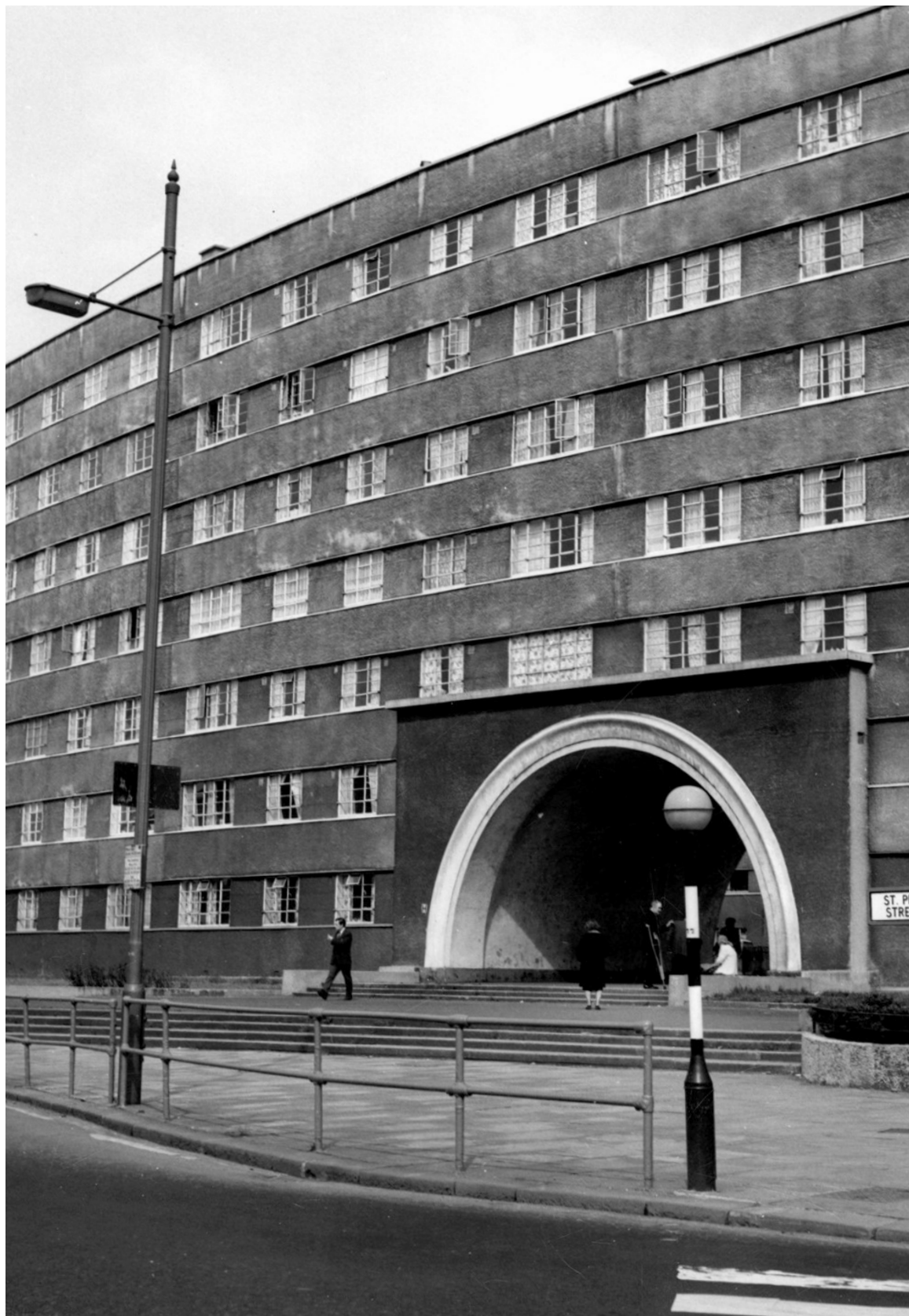
Figure 6.64: Main facade, Quarry Hill Flats
