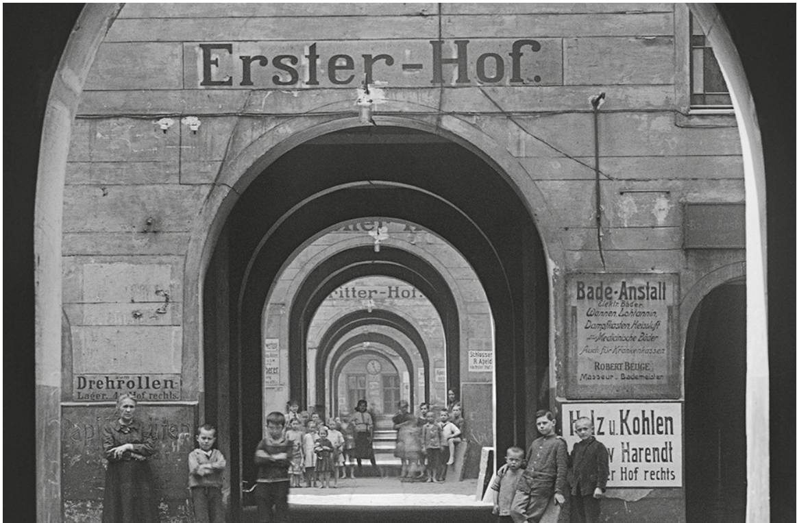
Figure 2.11: Meyers Hof, view through the courtyards
