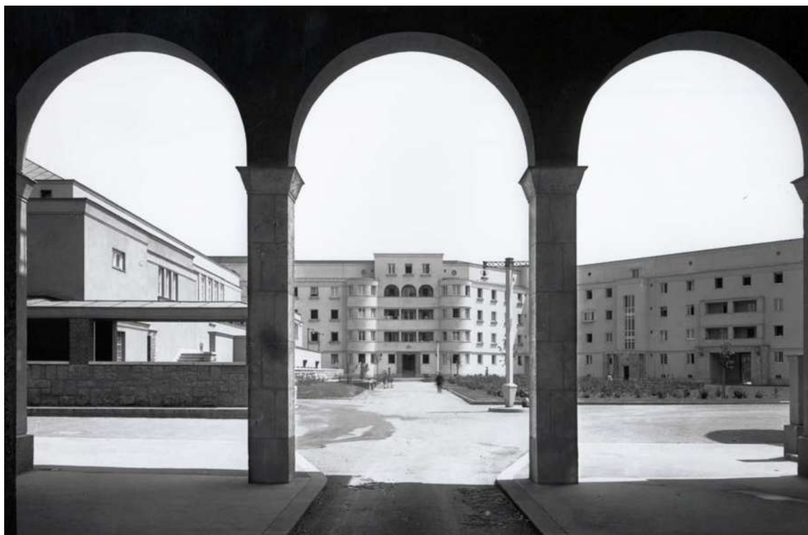
Figure 5.83: Arched passages, Karl-Seitz-Hof
