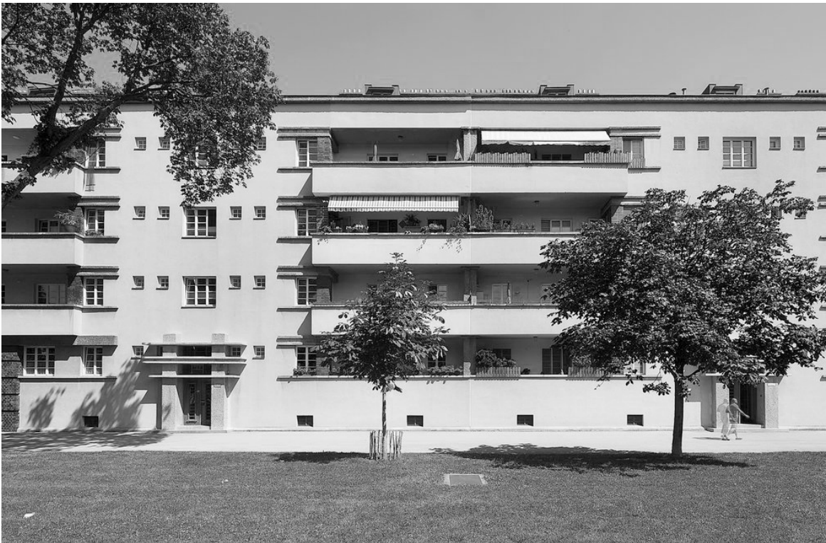
Figure 5.20: Facade of side structures from inner courtyard, Karl-Marx-Hof
