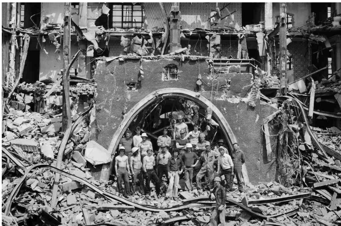
Figure 6.66: Archway after demolition, Quarry Hill Flats
