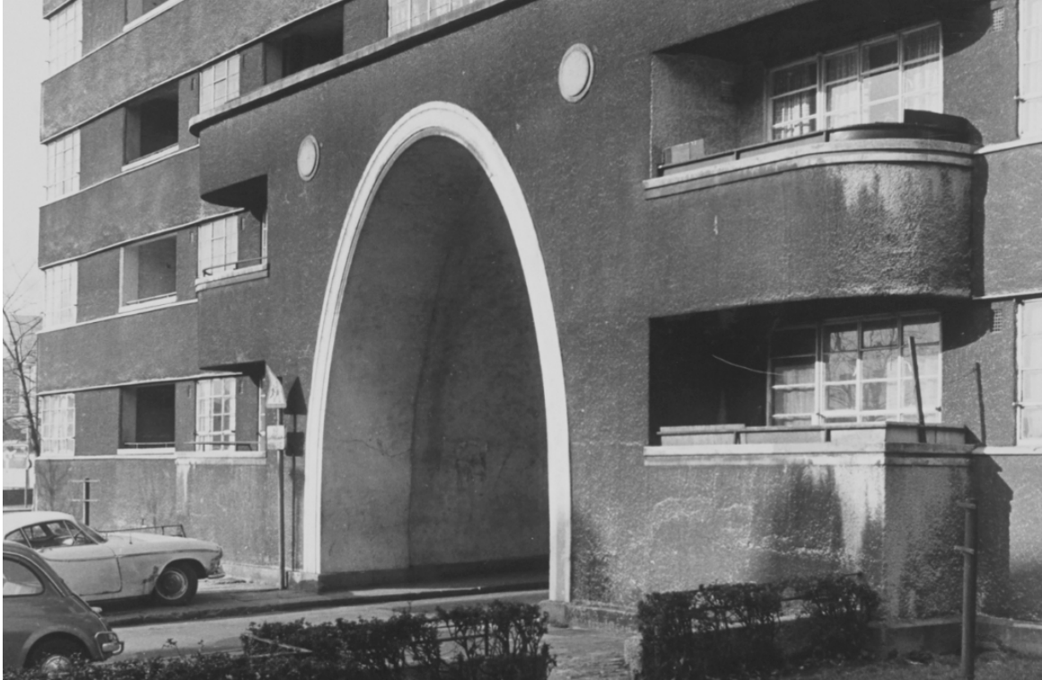
Figure 6.62: Archway, Quarry Hill Flats
