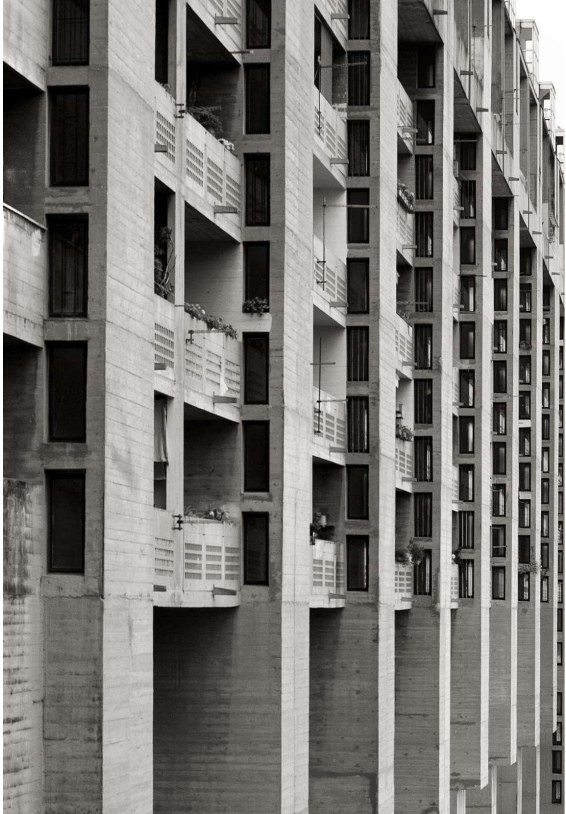
Figure 6.75: Facade, Rozzoli Melara
