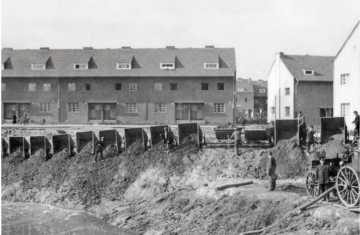
Figure 6.52: Building site, Hufeisensiedlung
