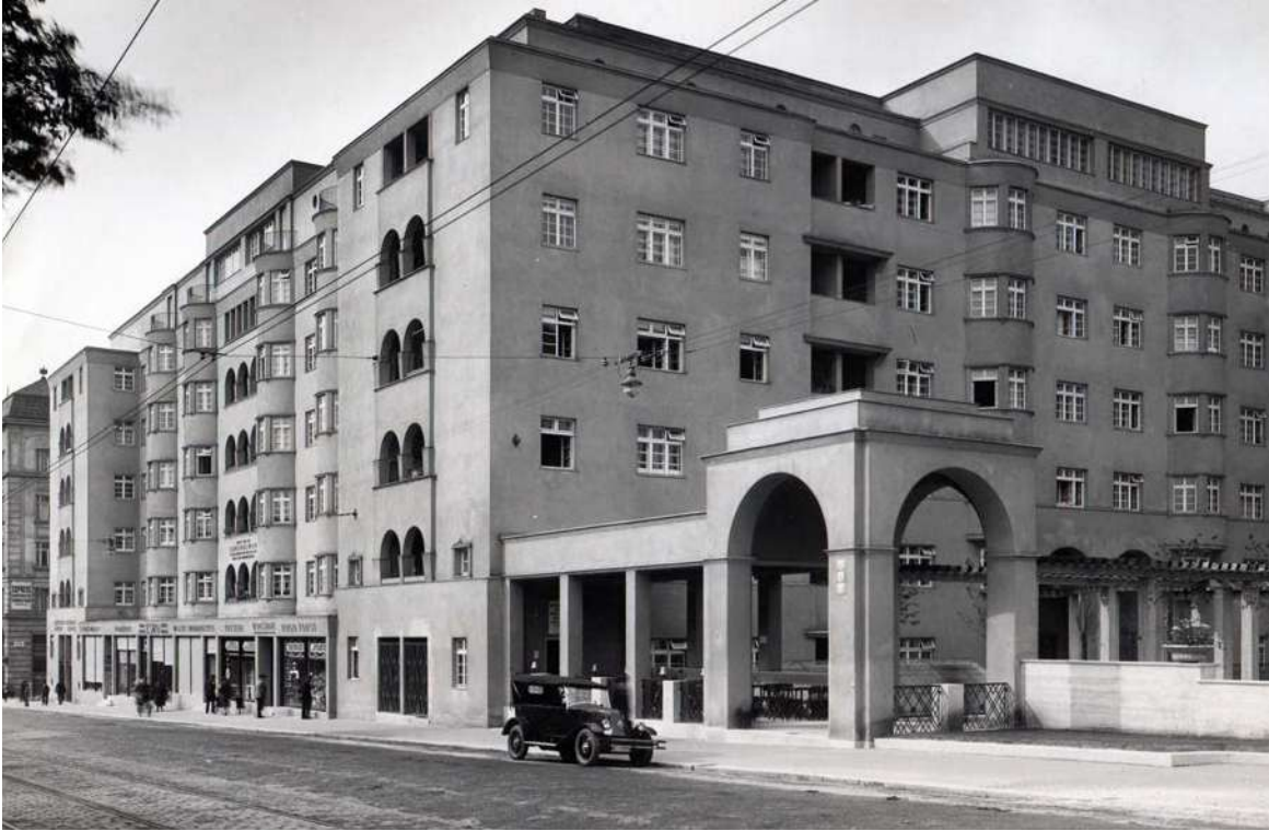
Figure 5.33: Left wing structure on Margaretenstraße , Reumannhof
