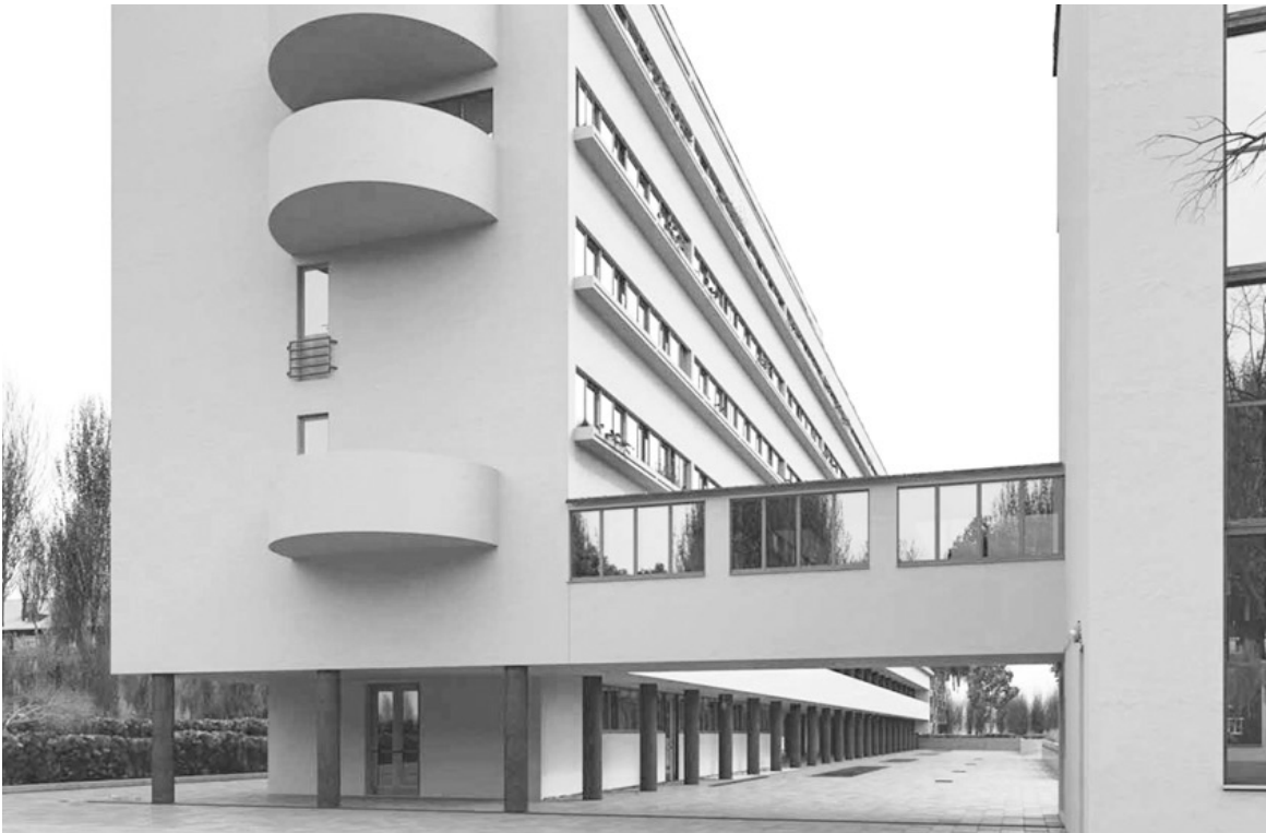
Figure 6.20: Southern facade, Dom Narkomfina
