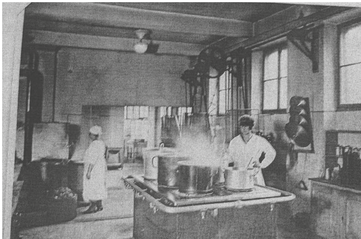
Figure 5.89: Main kitchen, Heimhof
