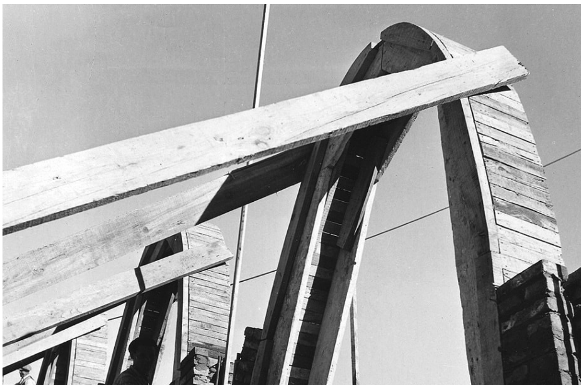
Figure 6.11: Side arches during construction, Climat de France
