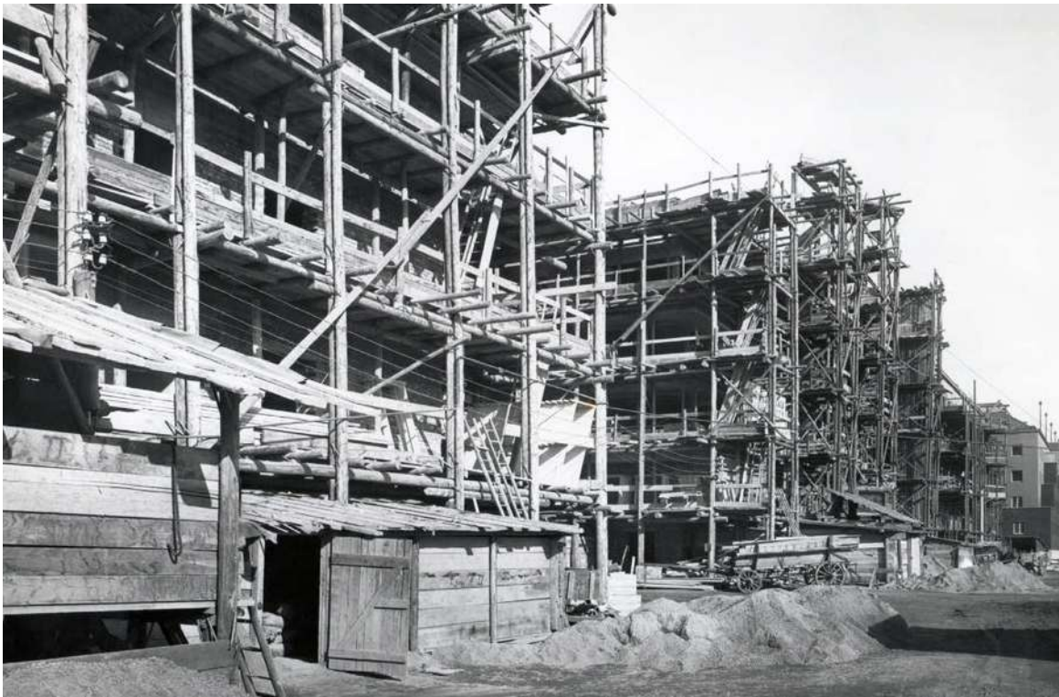
Figure 5.13: East facade during construction, Karl-Marx-Hof
