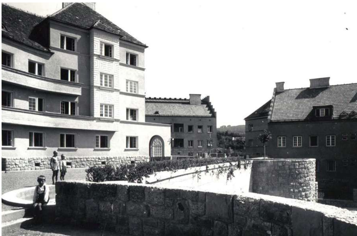
Figure 5.50: Facade Rosenackerstraße, Sandeithof
