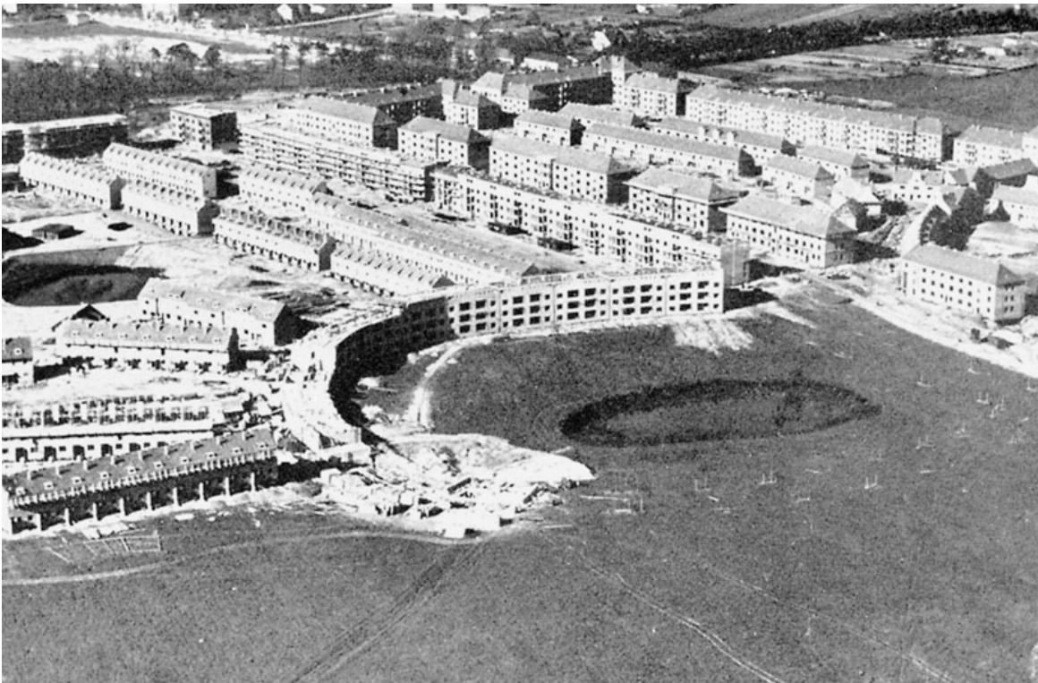
Figure 6.51: Building site, Hufeisensiedlung
