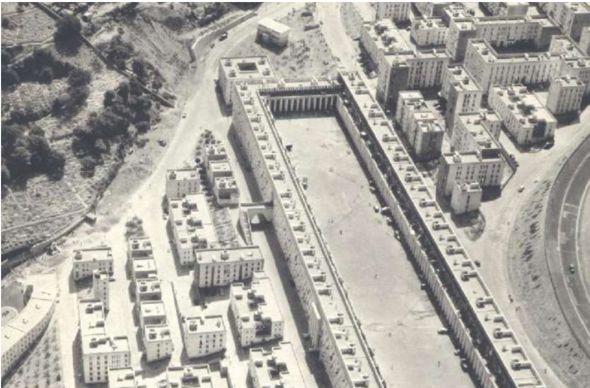
Figure 6.07: Aerial image, Climat de France
