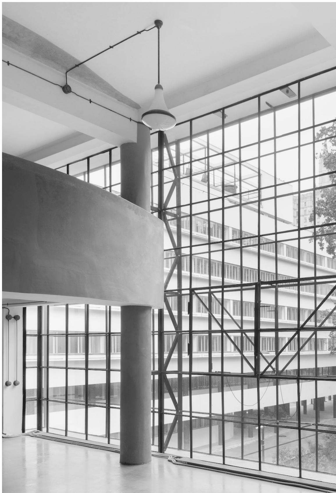
Figure 6.26: Facade detail of attached structure, Dom Narkomfina
