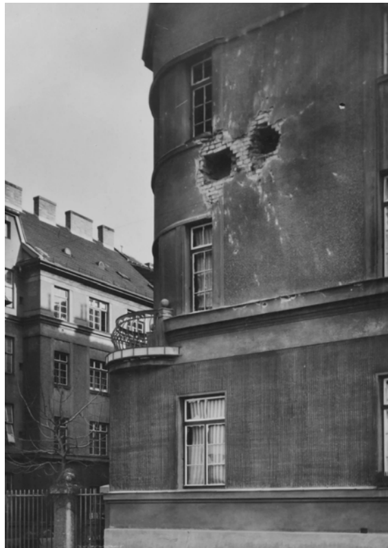
Figure 8.08: Krankenkassenhaus in Simmering, 1934
