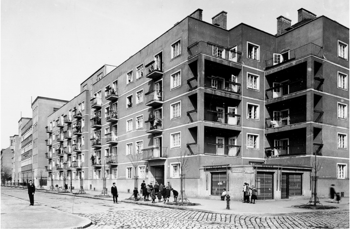
Figure 5.67: Facade along Pasettistraße, Sandleitenhof
