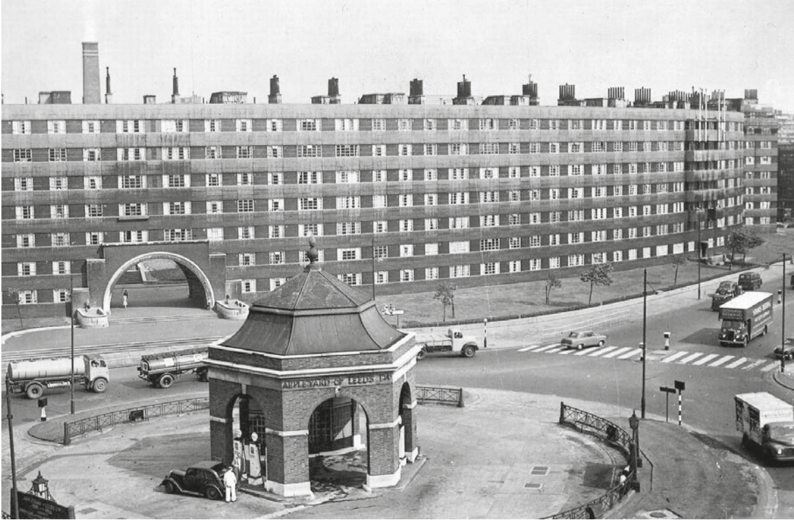
Figure 6.60: Urban placement, Quarry Hill Flats
