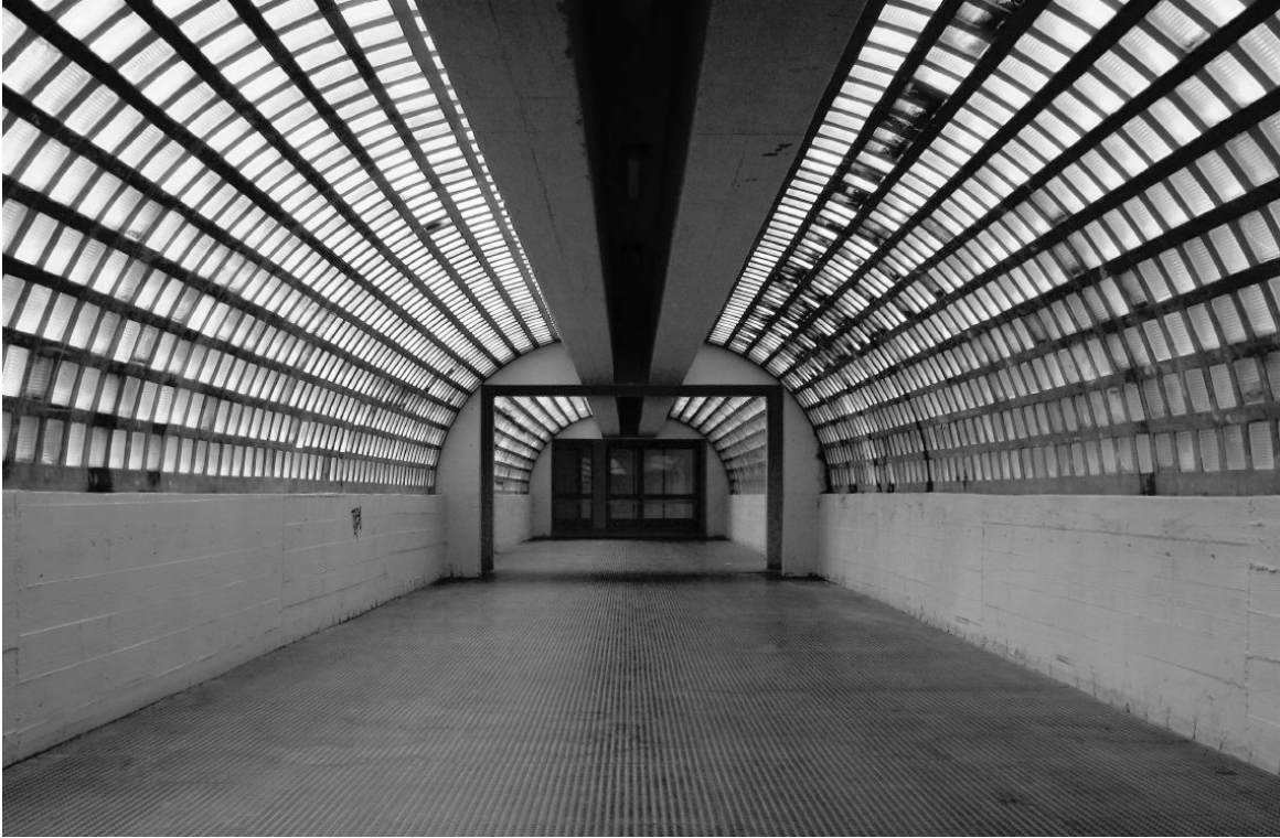
Figure 6.76: Hanging corridors, Rozzol Melara
