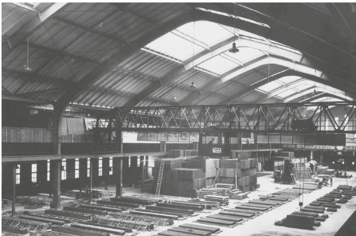
Figure 7.03: Prefabrication of building material
