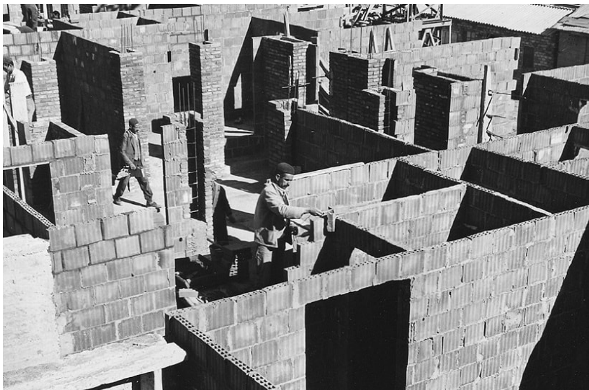
Figure 6.09: Construction site, Climat de France
