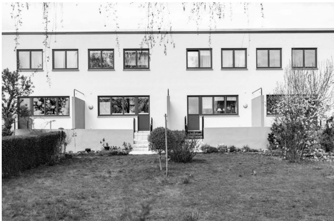
Figure 7.16: Front yard of row house, Siedlung Westhausen
