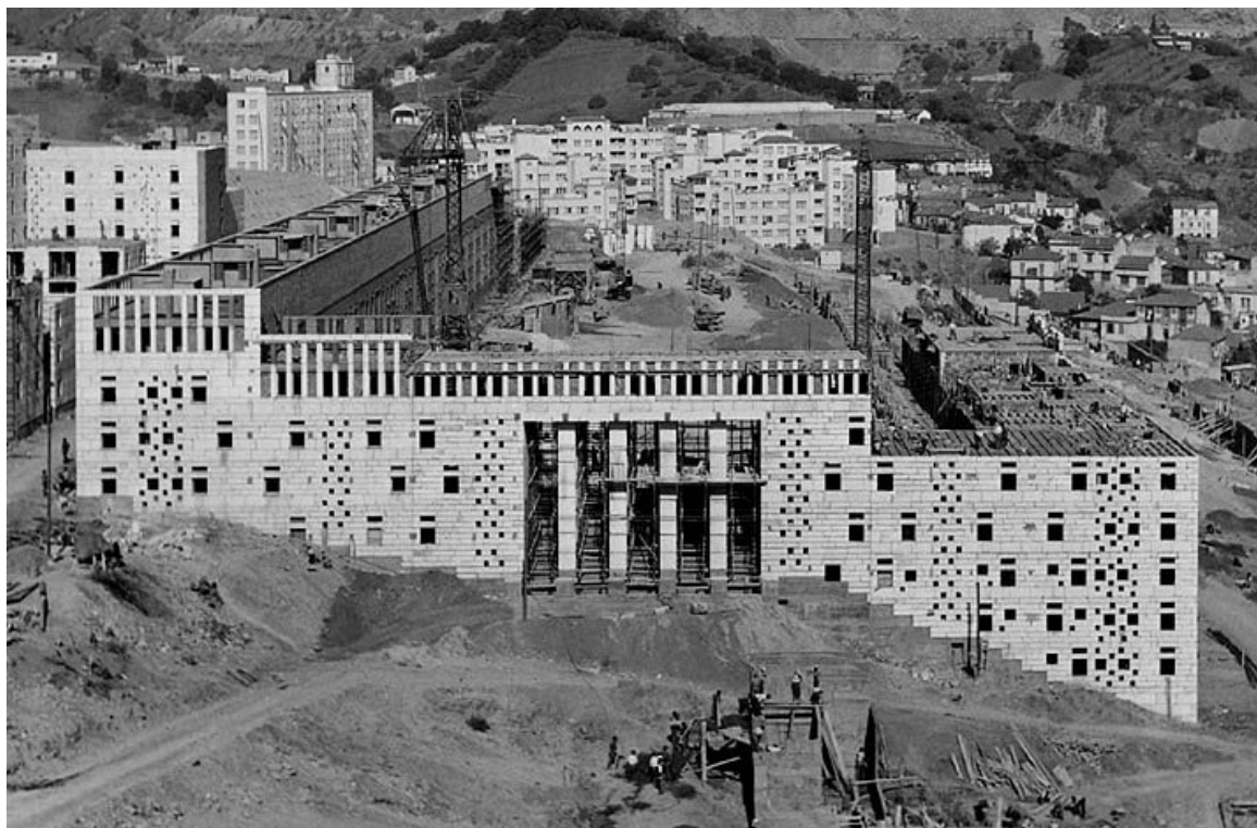
Figure 6.08: During construction, Climat de France
