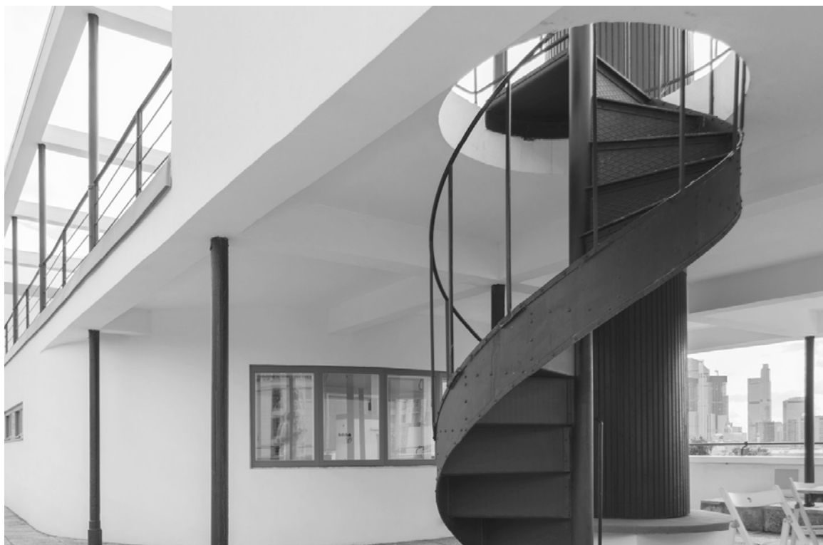
Figure 6.22: Rooftop and communal laundry, Dom Narkomfina
