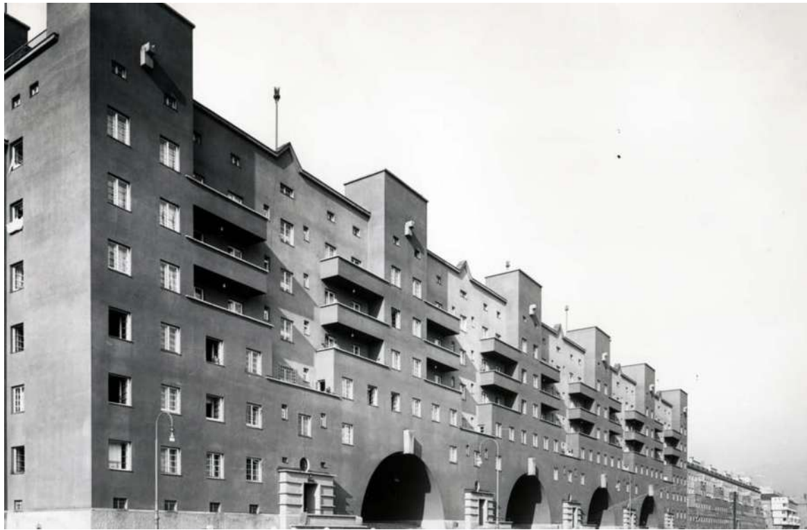
Figure 5.14: East facade after completion, Karl-Marx-Hof
