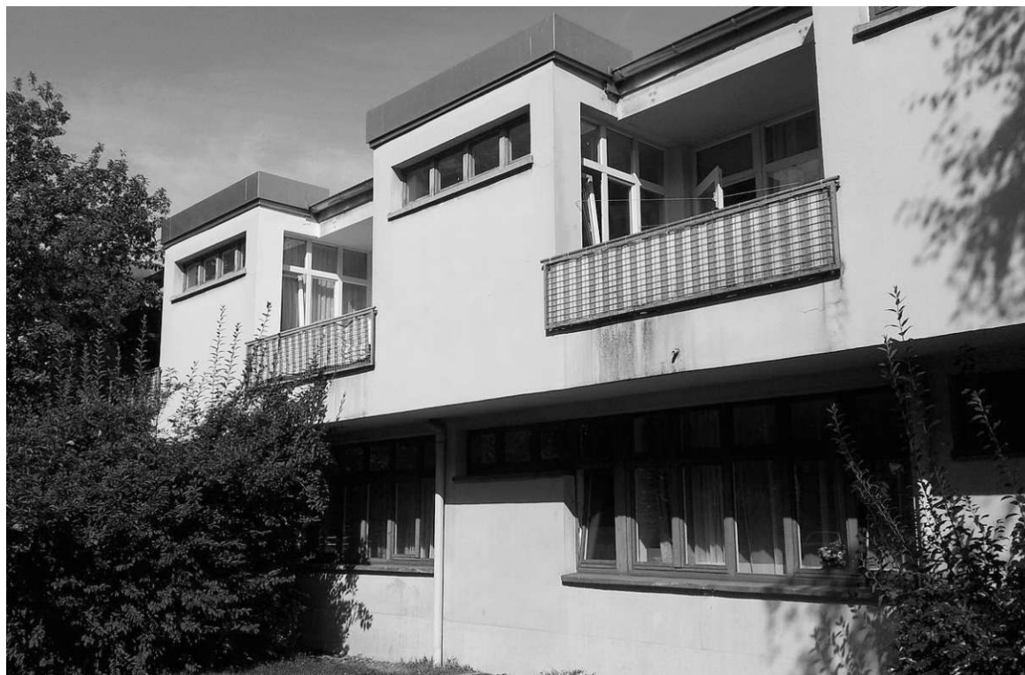
Figure 7.19: Rowhouse, Siedlung Hellerhof
