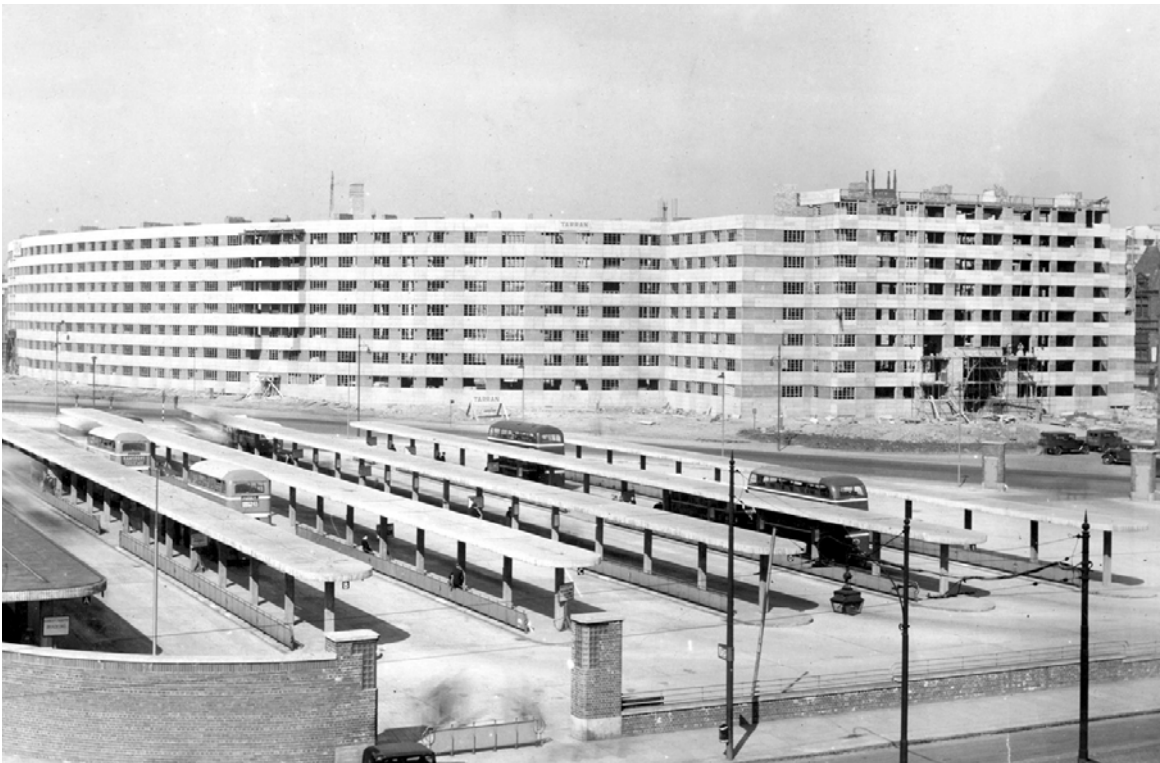
Figure 6.61: During construction, Quarry Hill Flats
