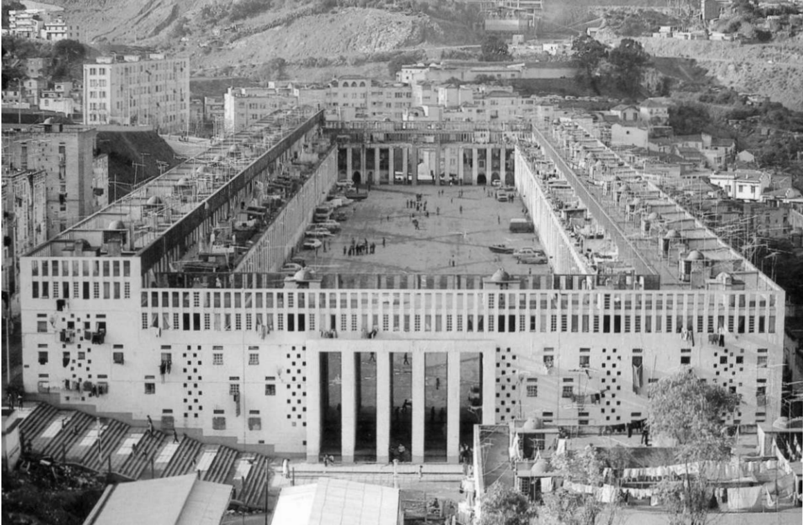
Figure 6.06: After completion, Climat de France
