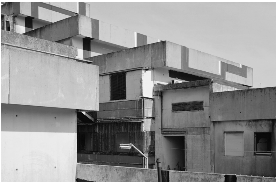
Figure 6.33: Roof terraces, Vele di Scampia
