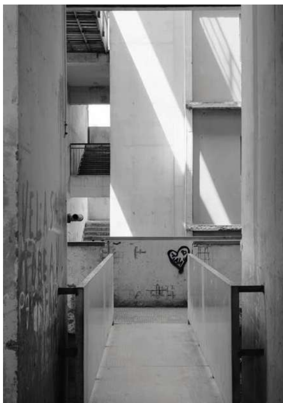
Figure 6.35: View from staircase, Vele di Scampia
