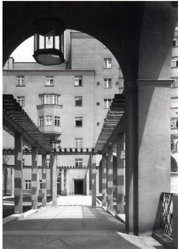
Figure 5.35: Pergolas in cour d'honneur, Reumannhof
