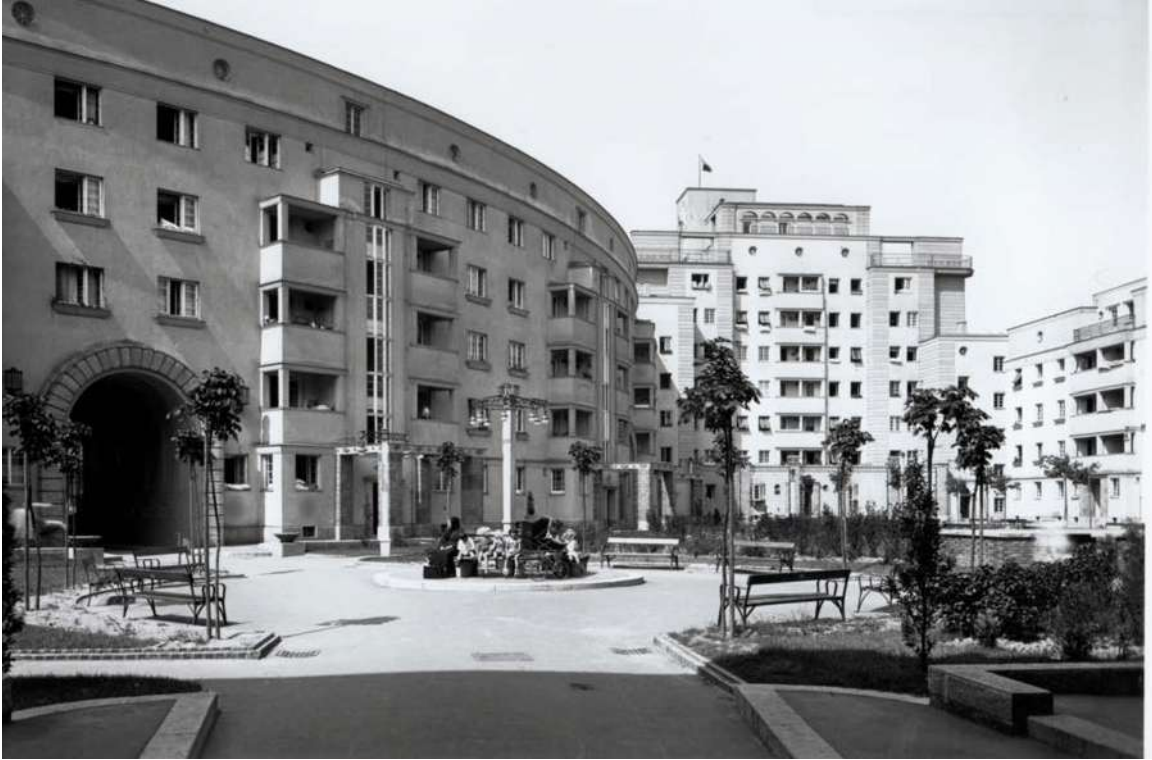
Figure 5.80: Inner courtyard behind cour d'honneur, Karl-Seitz-Hof
