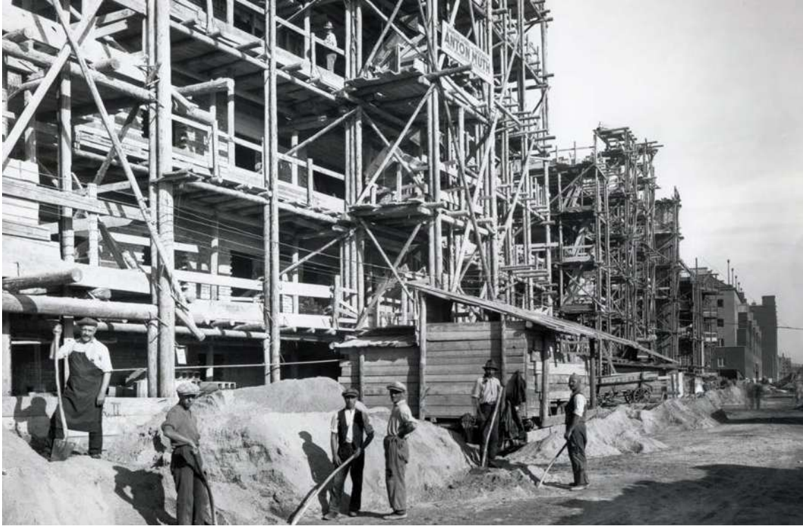
Figure 3.07: Construction of the brick outer wall, Karl-Marx-Hof
