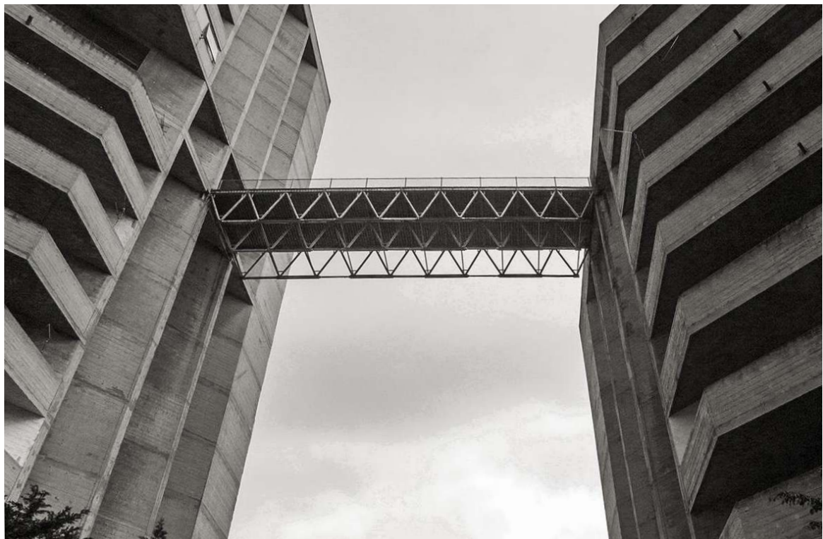
Figure 6.72: Corner connection, Rozzol Melara
