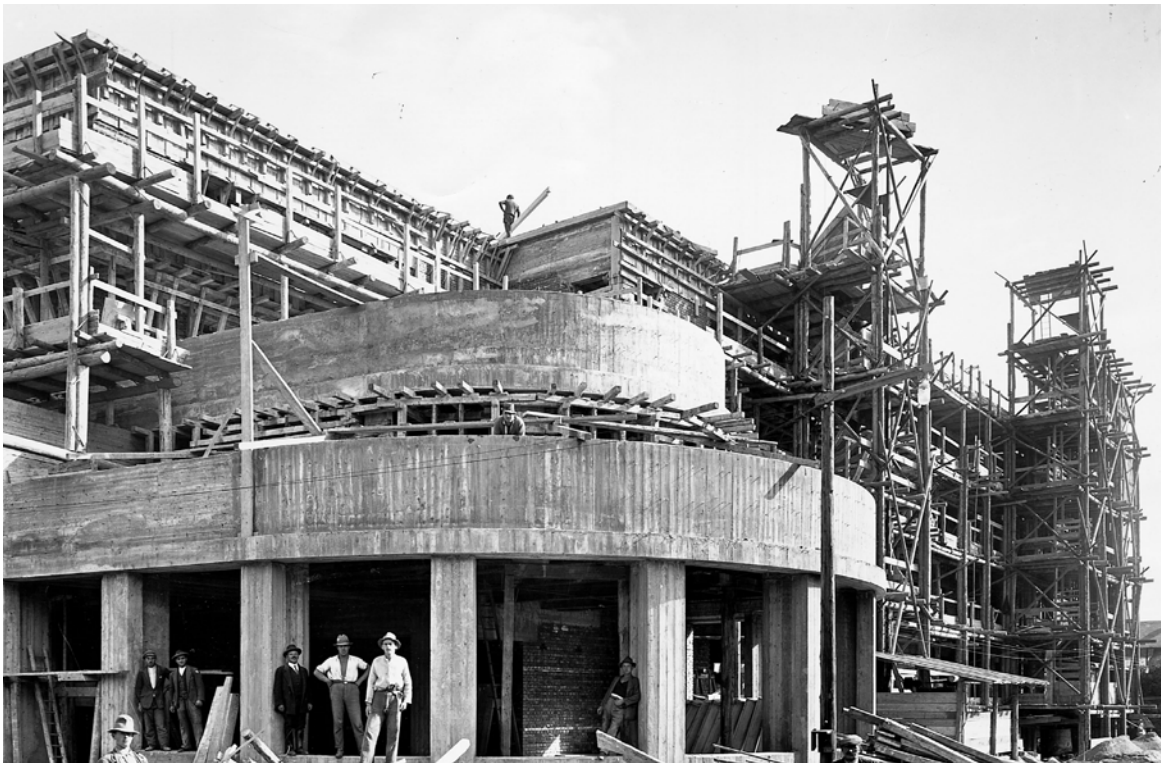
Figure 3.08: Construction of the concrete structure, Interior Design Consulting Center (BEST), Karl-Marx-Hof
