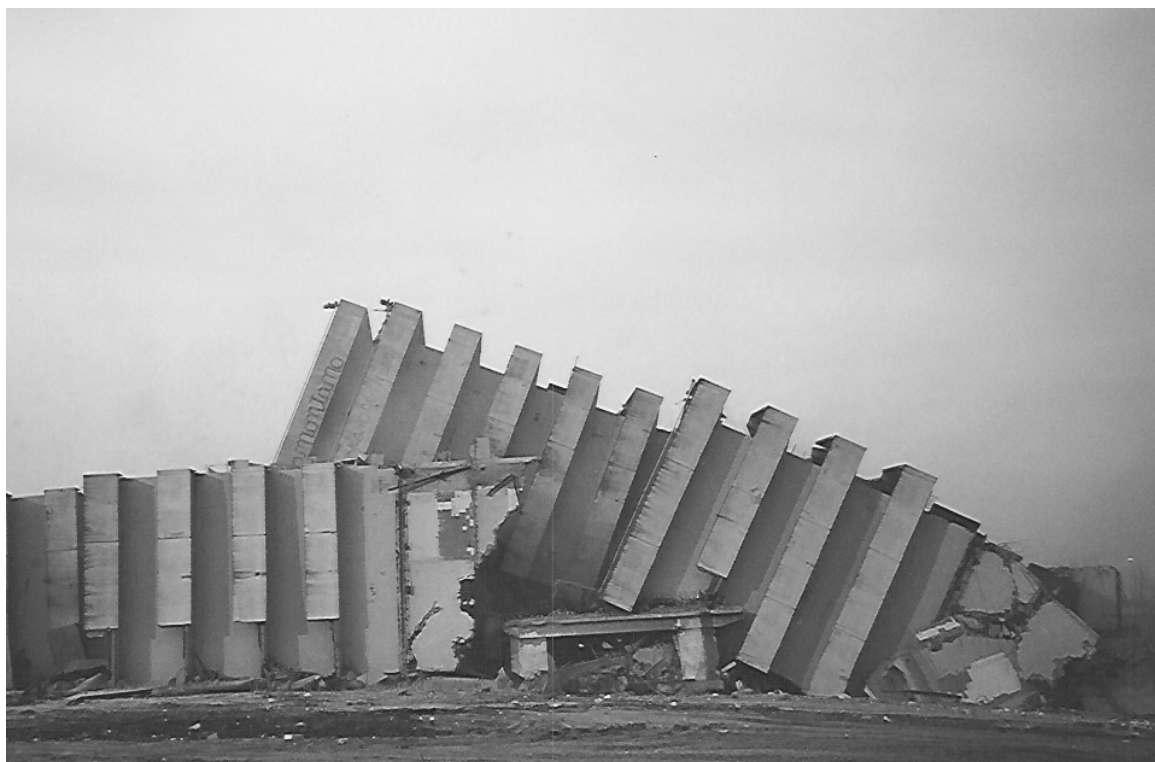
Figure 6.40: After demolition, Vele di Scampia
