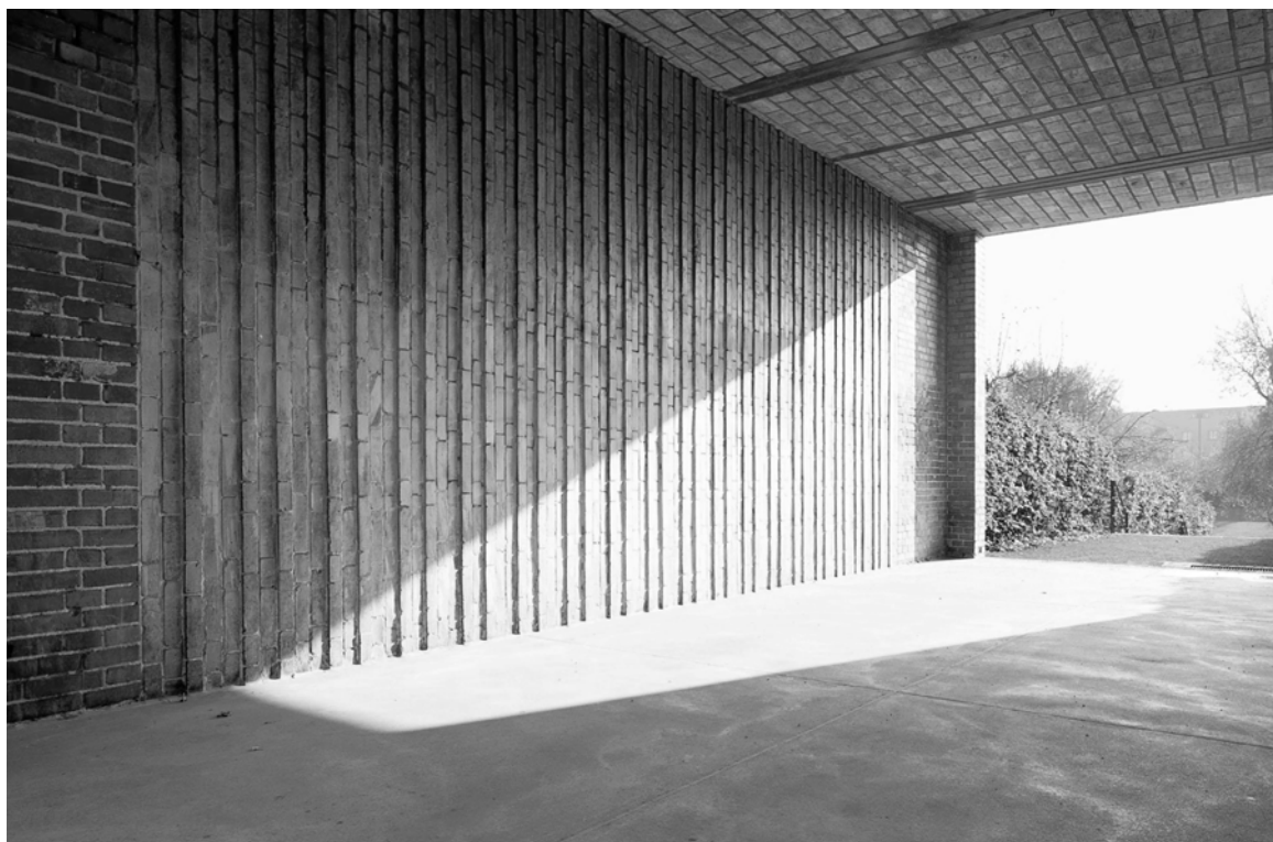
Figure 6.56: Passage through the main structure, Hufeisensiedlung
