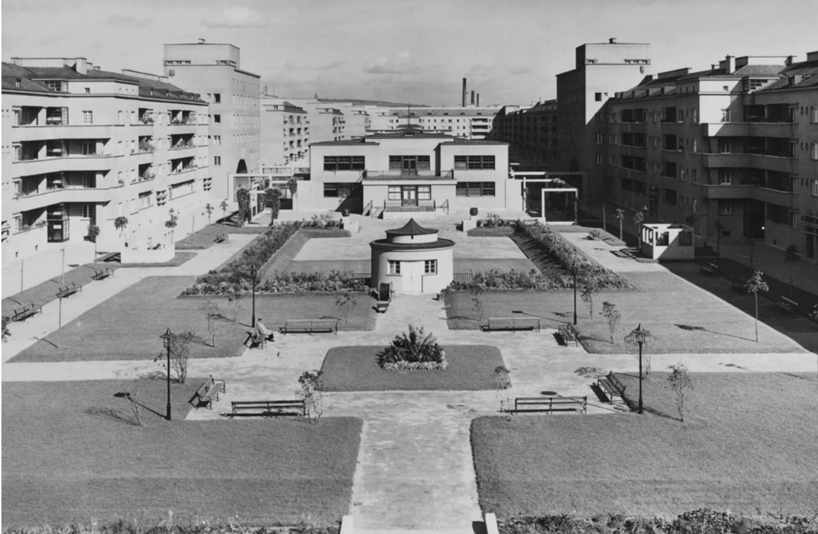
Figure 5.15: Inner courtyard, Karl-Marx-Hof
