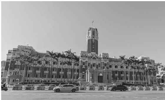
Fig.07 Presidential Office Building (Taiwan Governor's office), 1919
