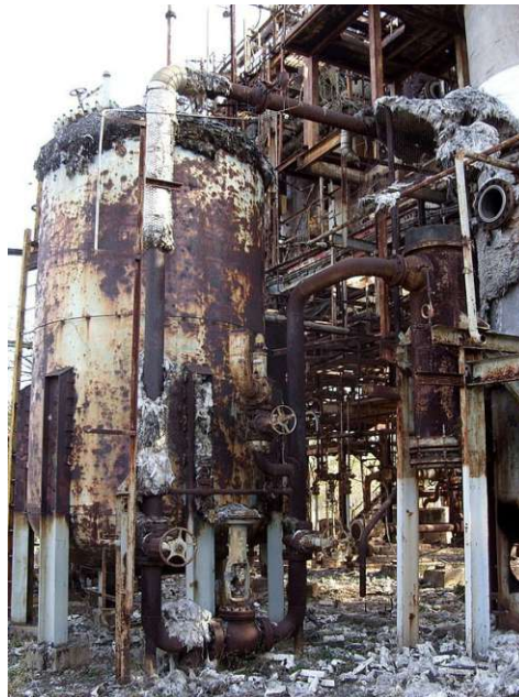
Figure 18: Tank at Bhopal
