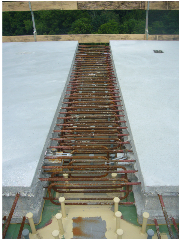
Figure 2. Stitching detail of transverse joint of Bahretal bridge [9]. Photo courtesy of company group Max Bögl/Johann Schlapschy.
