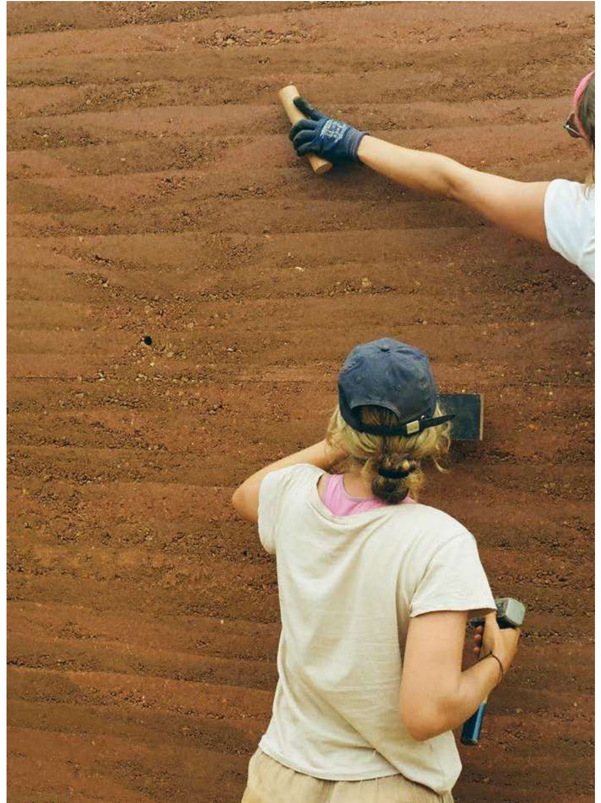
Fig.201: Aftercare of the walls
