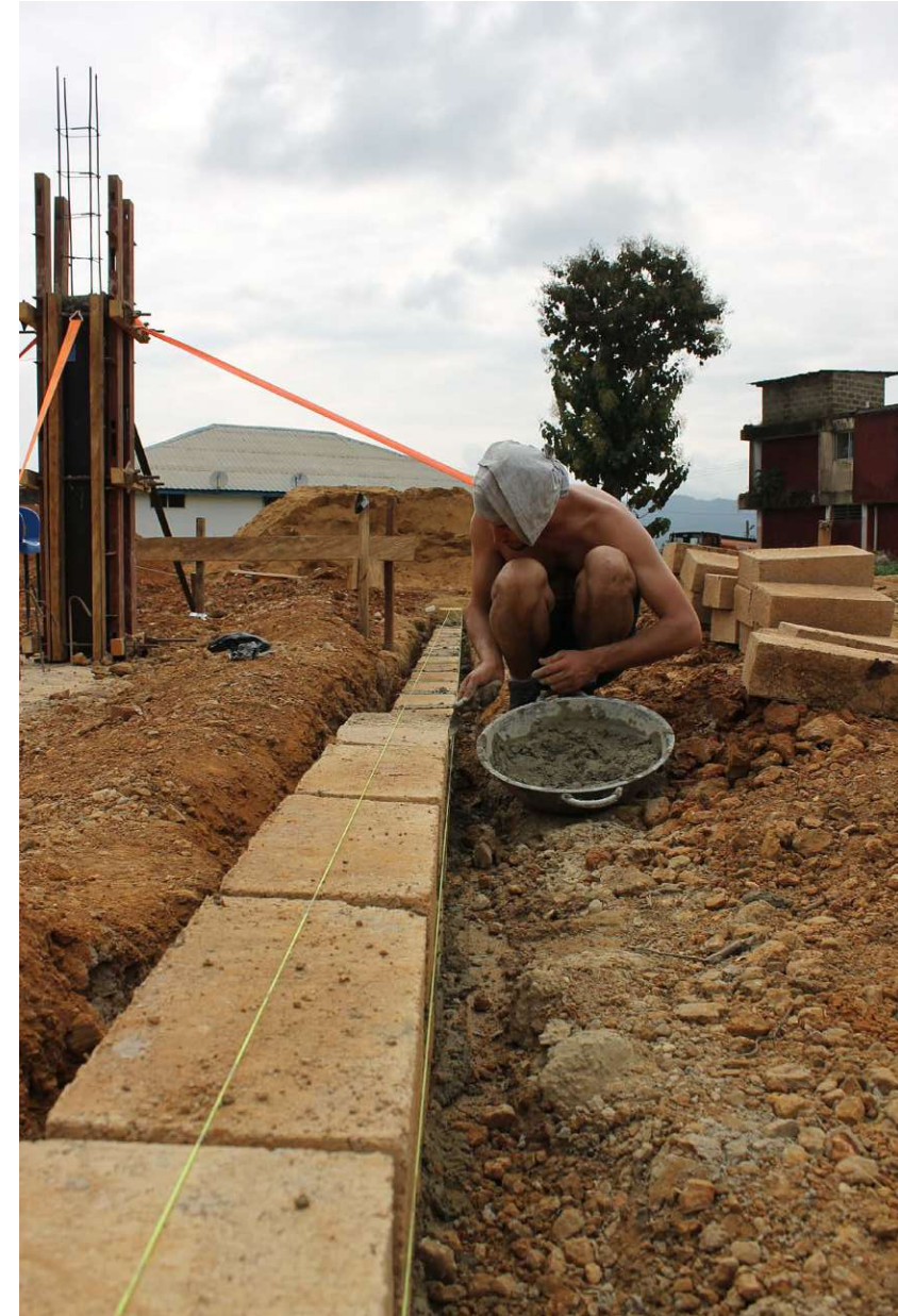
Fig.150: Construction of the perimeter wall with cement blocks | Week 5
