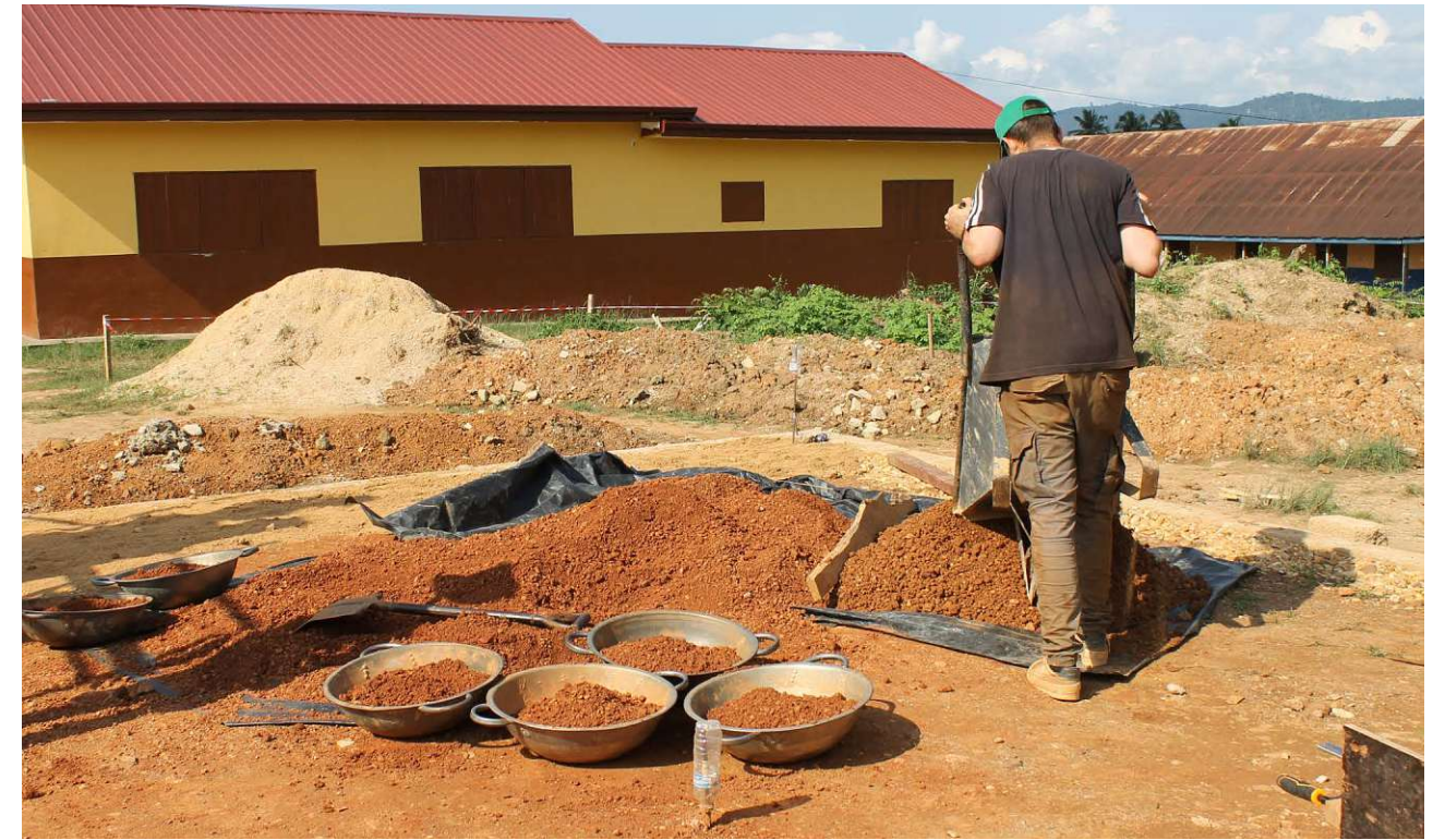
Fig.185: Earth storage outside | week 3 -6
