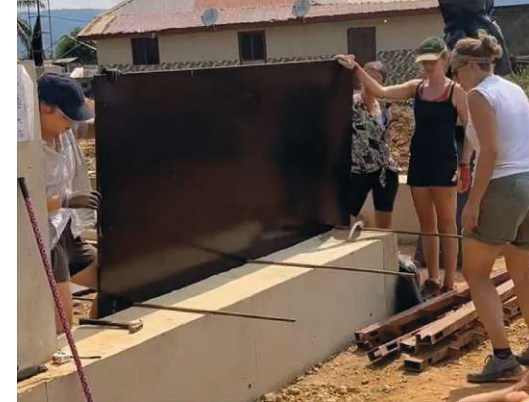
Fig.187: First, the formwork was positioned on the plinth
