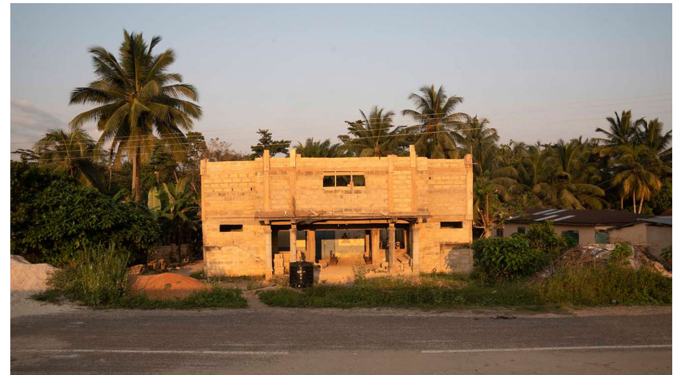
Fig.43: Nsutam construction methods IUnfinished cement block house
