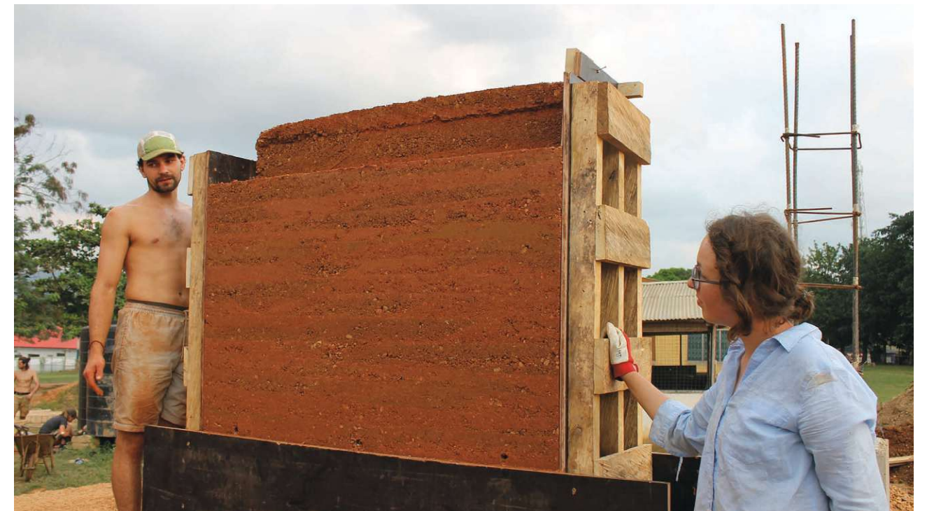
Fig.197: Wooden spacer holder for the ring beam
