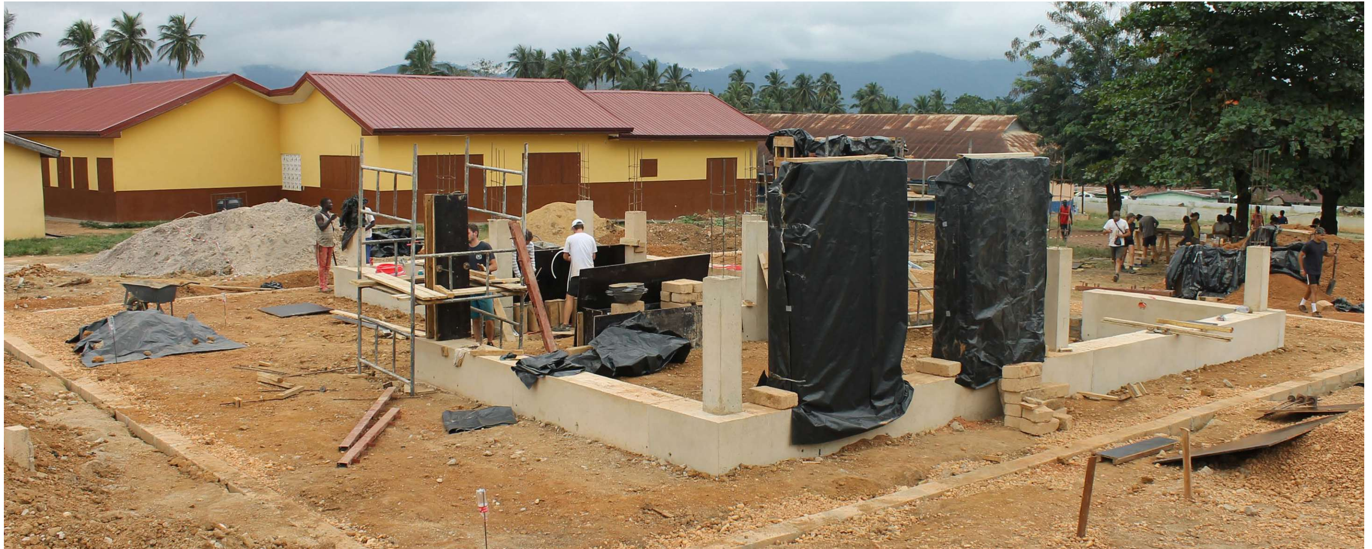
Fig.207: Project status at week 6
