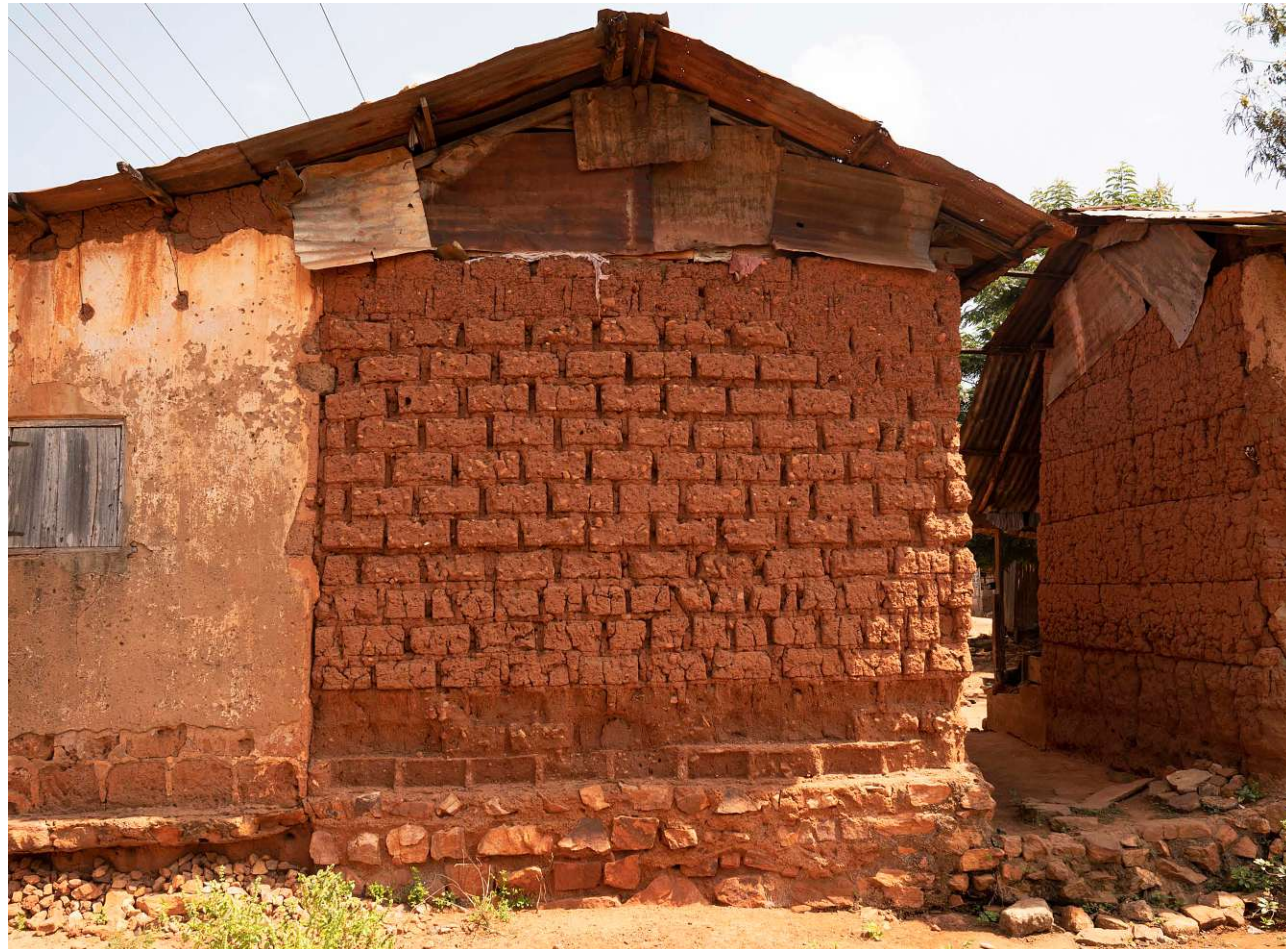
Fig.61: Earth brick house with a quarry stone plinth | Eastern Region
