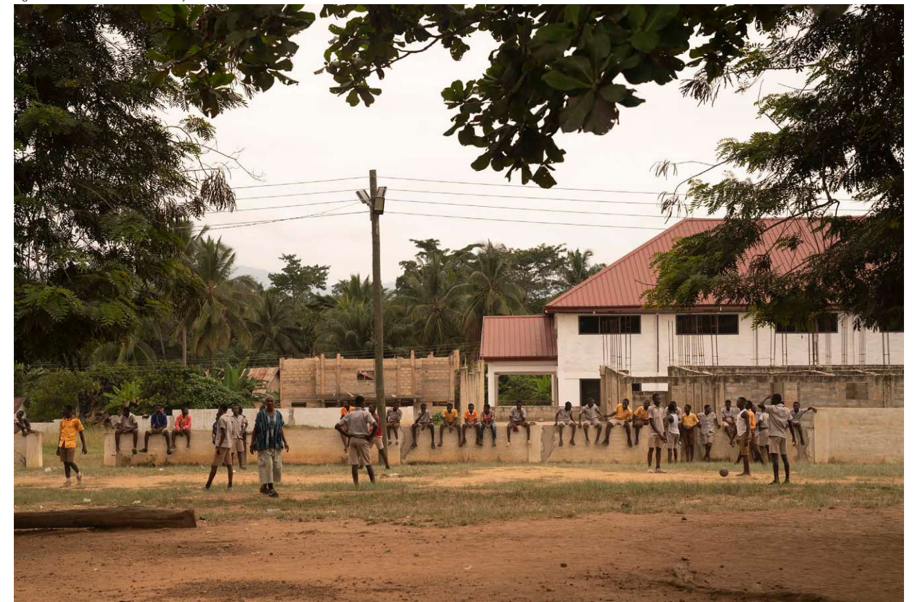
Fig.135: Construction site I July 2022
