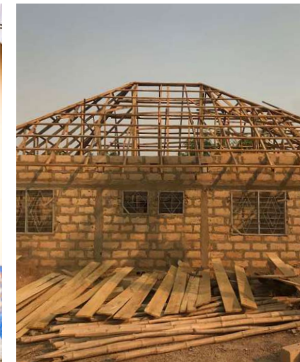
Fig.50: Cement block house with wooden roof frame
