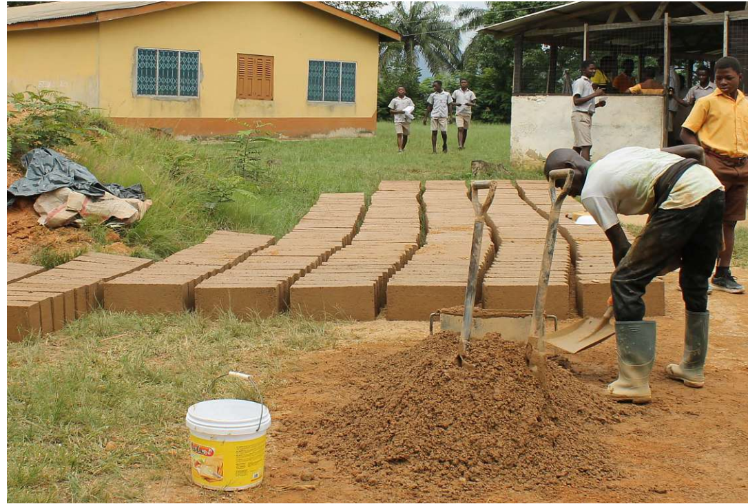
Fig.44: Production of Cement blocks | Sand, cement and water get mixed.
