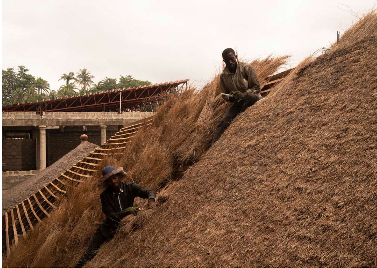
Fig.67: Construction of a straw roof | Eastern Region
