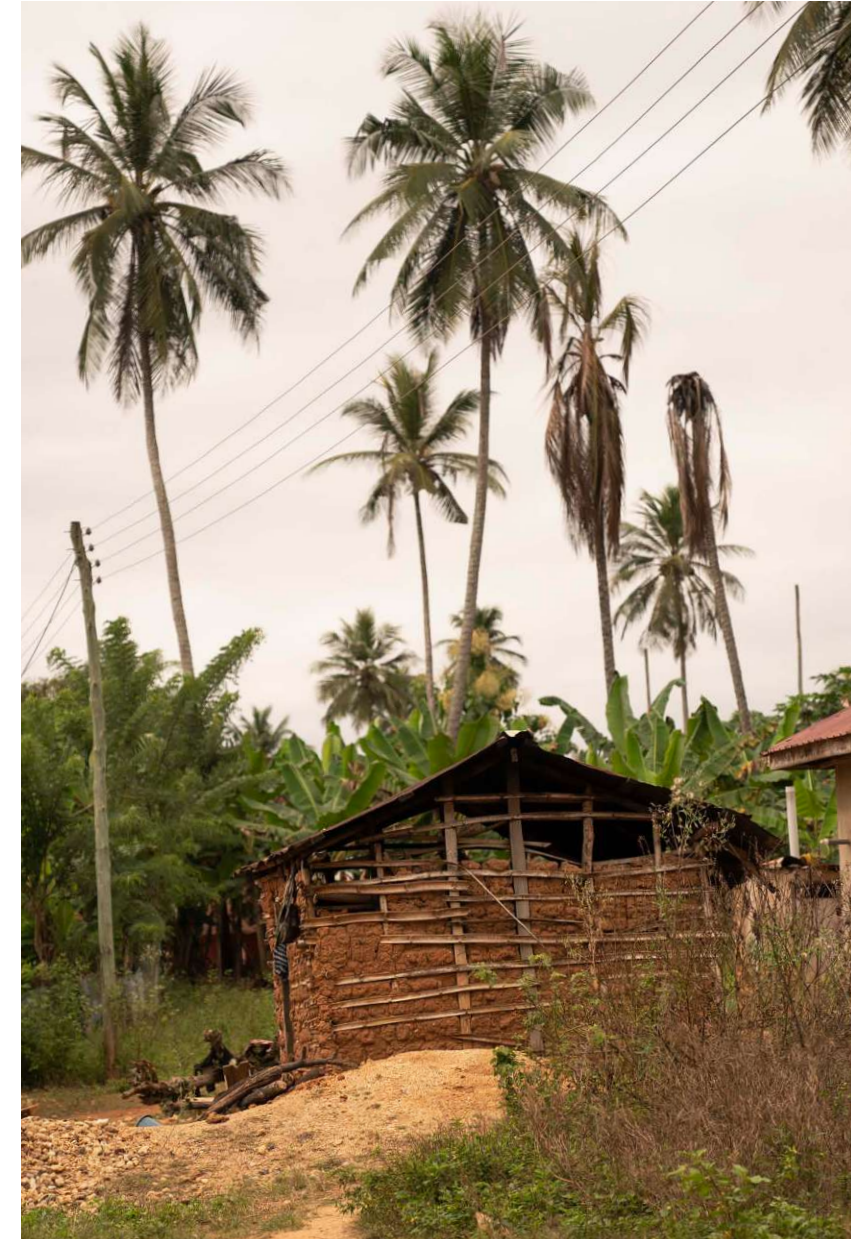
Fig.66: Wattle and daub house with a skeleton structure of bamboo and wood | Nsutam
