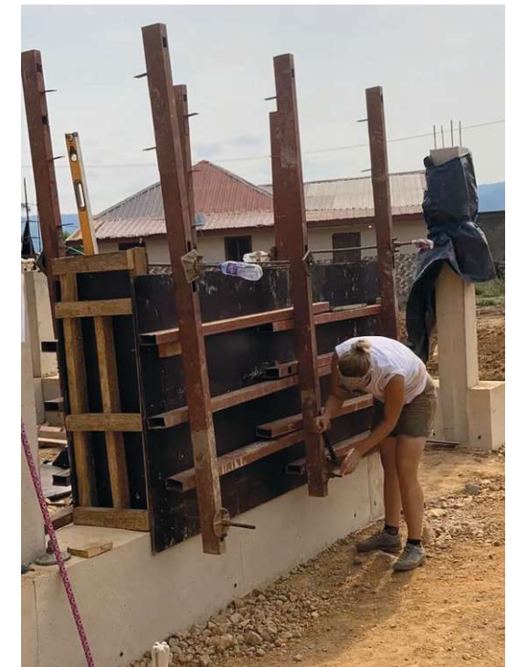
Fig.190: When everything was set up, the tie rods were tightened
