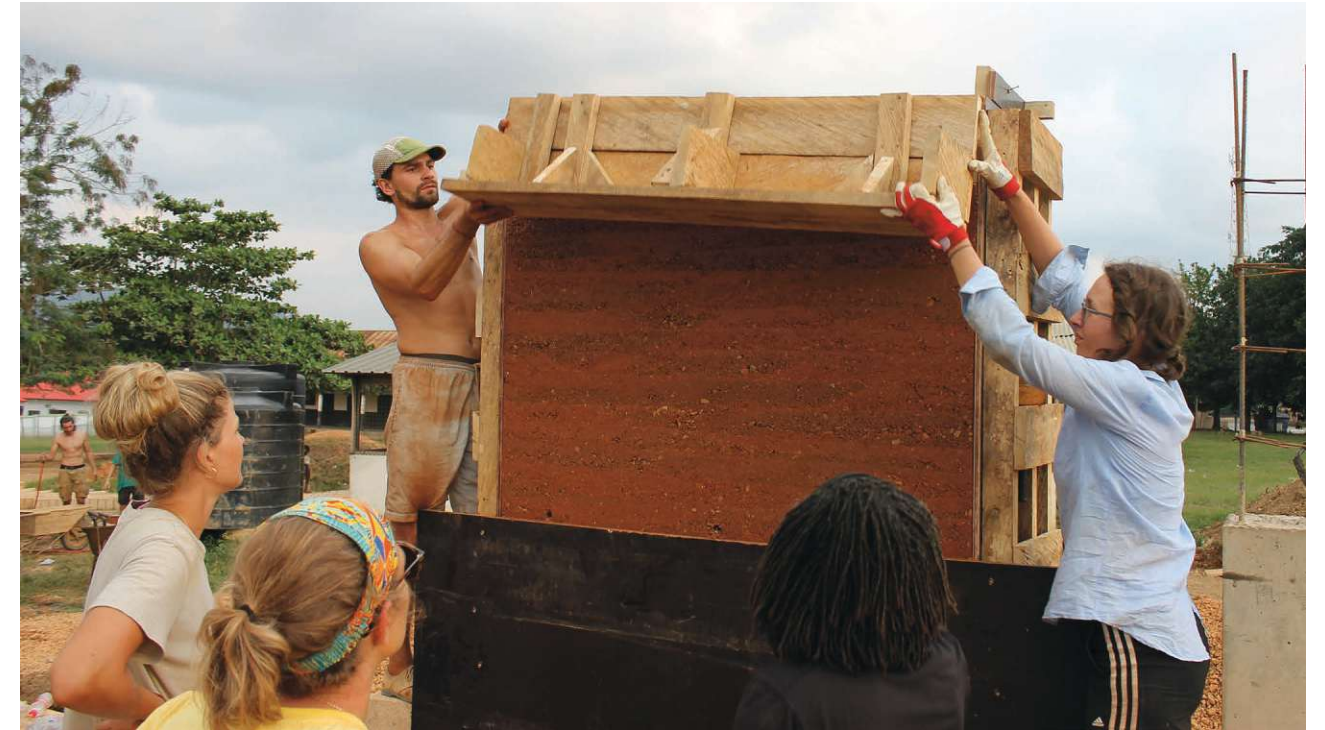
Fig.196: Wooden spacer holder for the ring beam
