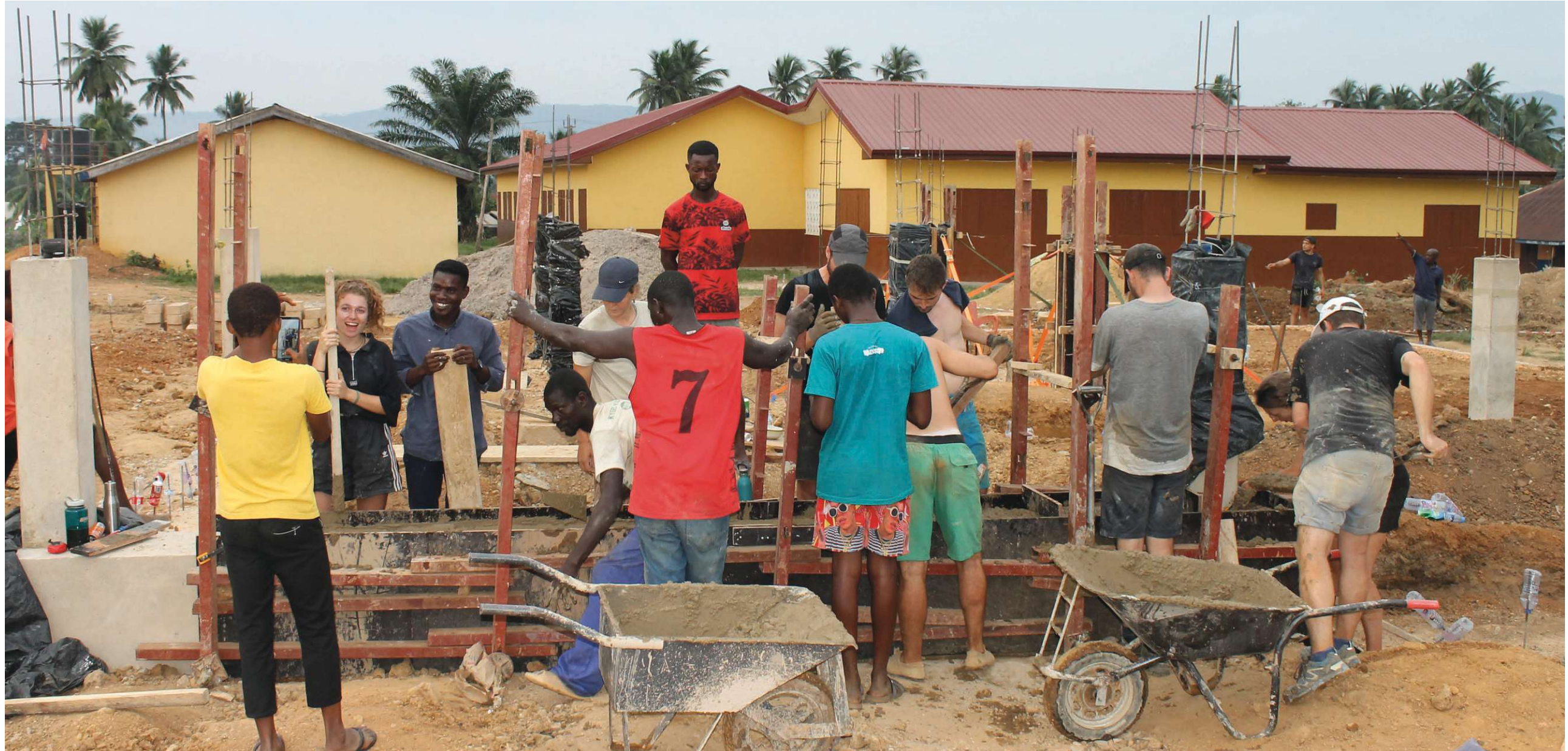
Fig.148: Concreting the plinth | Week 4
