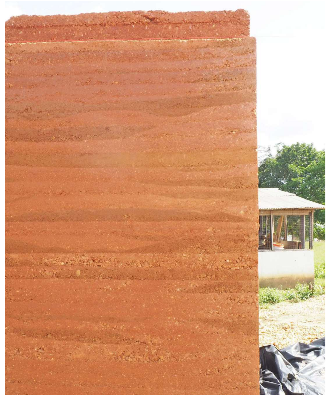
Fig.205: First completed rammed earth wall | Week 5
