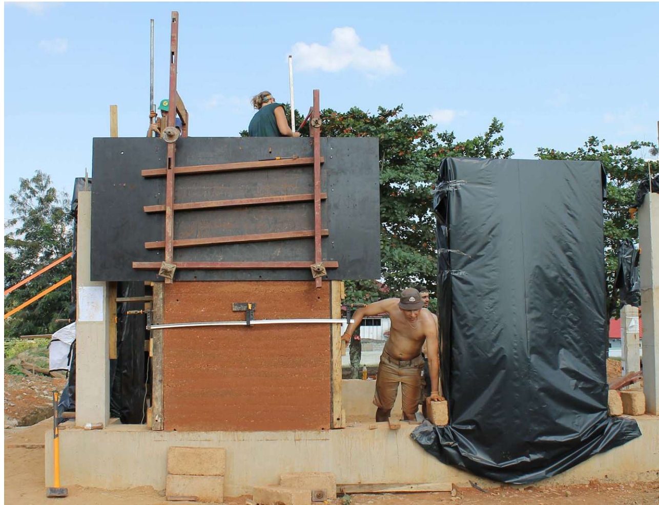
Fig.198: Shifting the formwork | Formwork was pulled upwards
