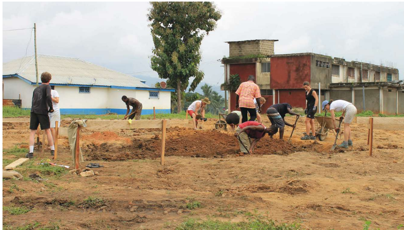
Fig.144: Foundation digging | Week 1
