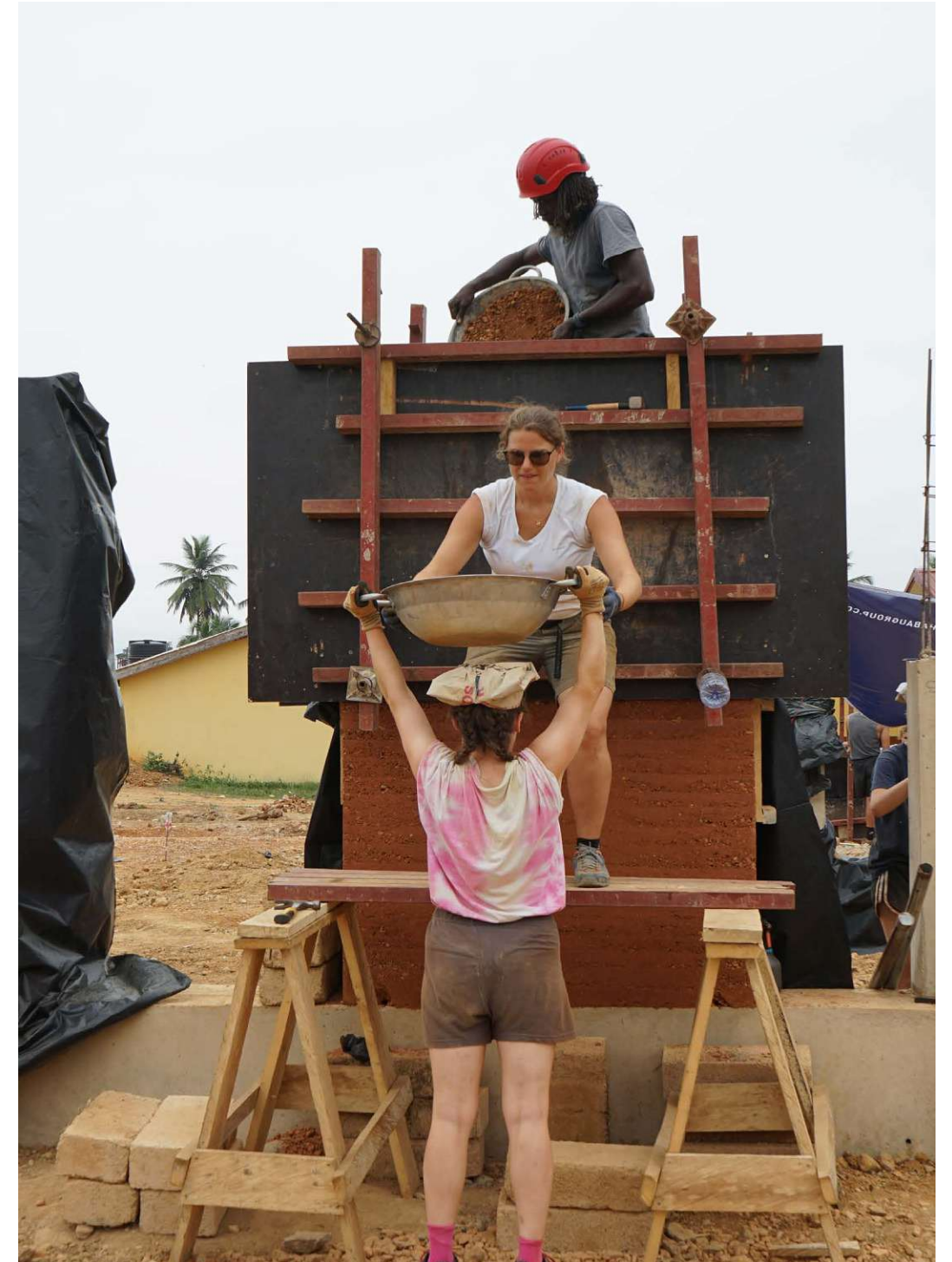
Fig.191:Filling in the Earth
