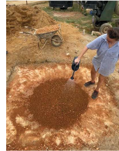
Fig.180: Fine gravel were dumped onto the mixing area
