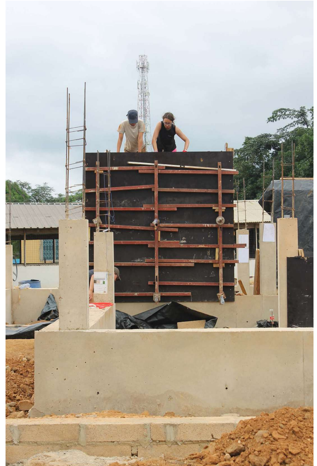
Fig.199: Shifting the formwork | Second formwork was installed
