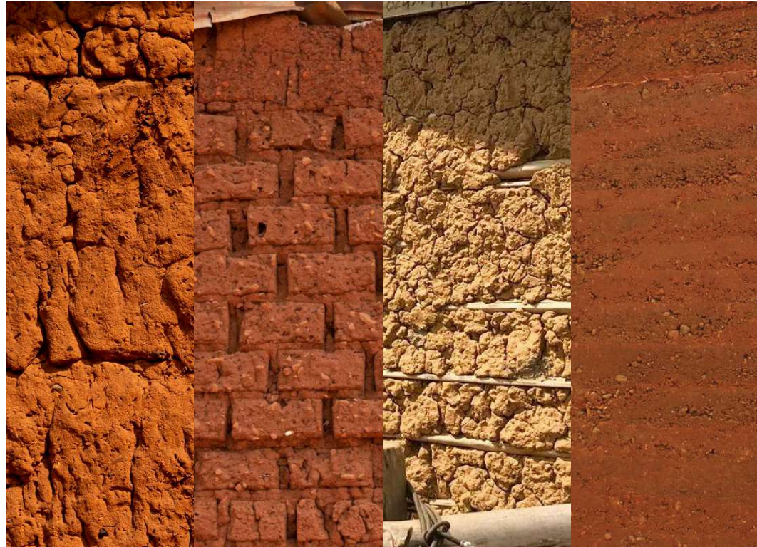
Fig.52 :Overview of the different earth techniques
