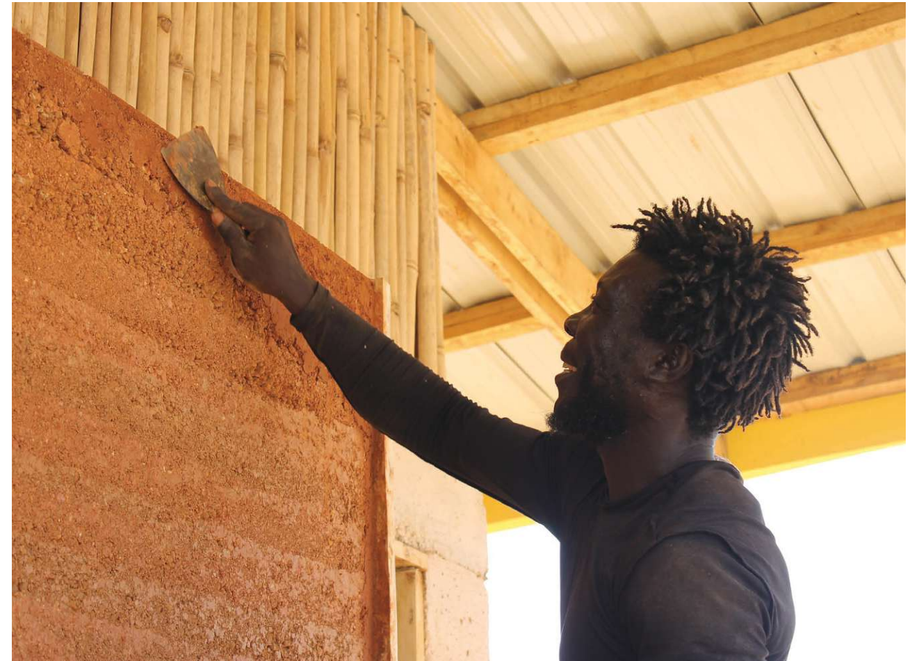
Fig.203: Aftercare of the walls
