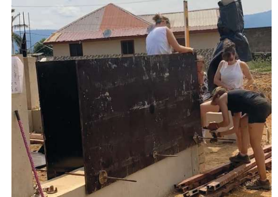
Fig.188: Then the two sideboard were added
