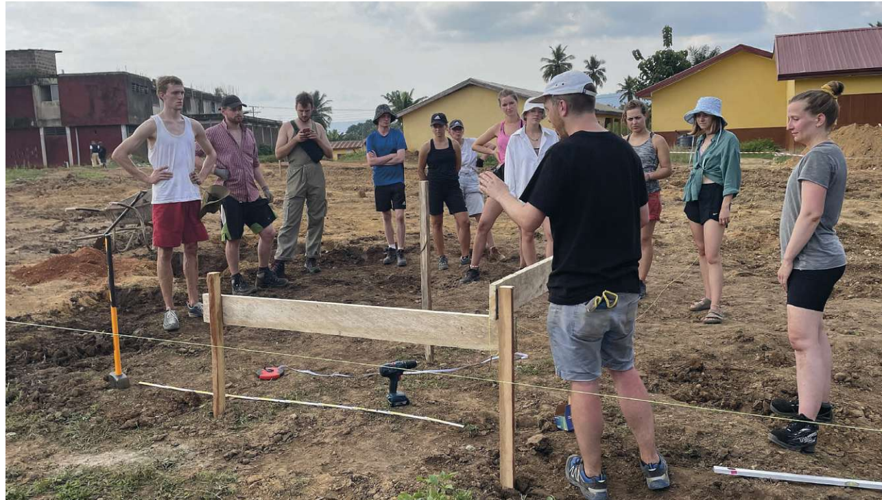
Fig.143: Setting up of the batter board | Week 1
