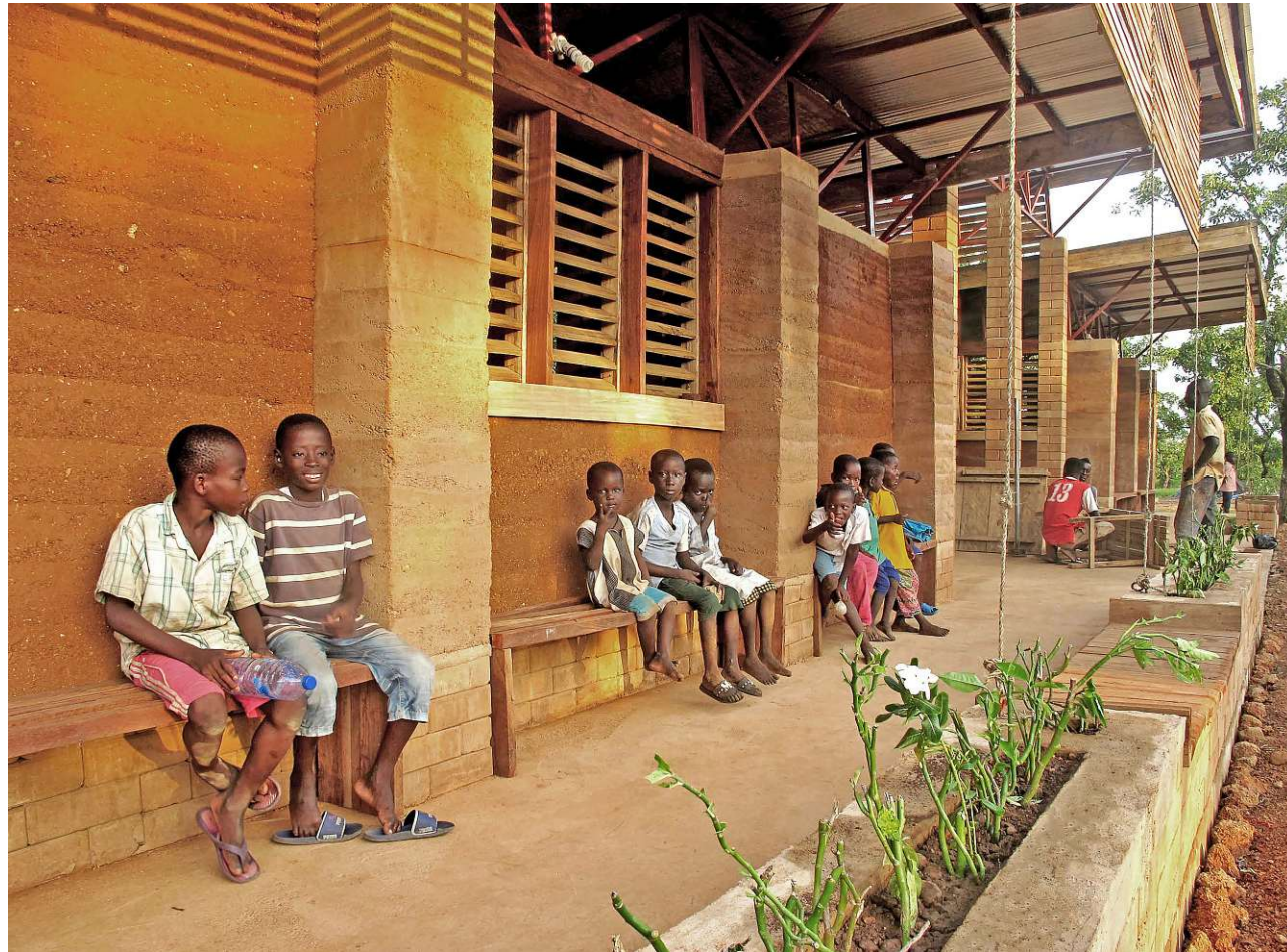
Pilot Project ArchiFair: „mudCAFETERIA“ Built area: 200 m 2 Construction period: 16 Weeks Building costs: 20.000 Euro Financed: Sponsors and Donations
