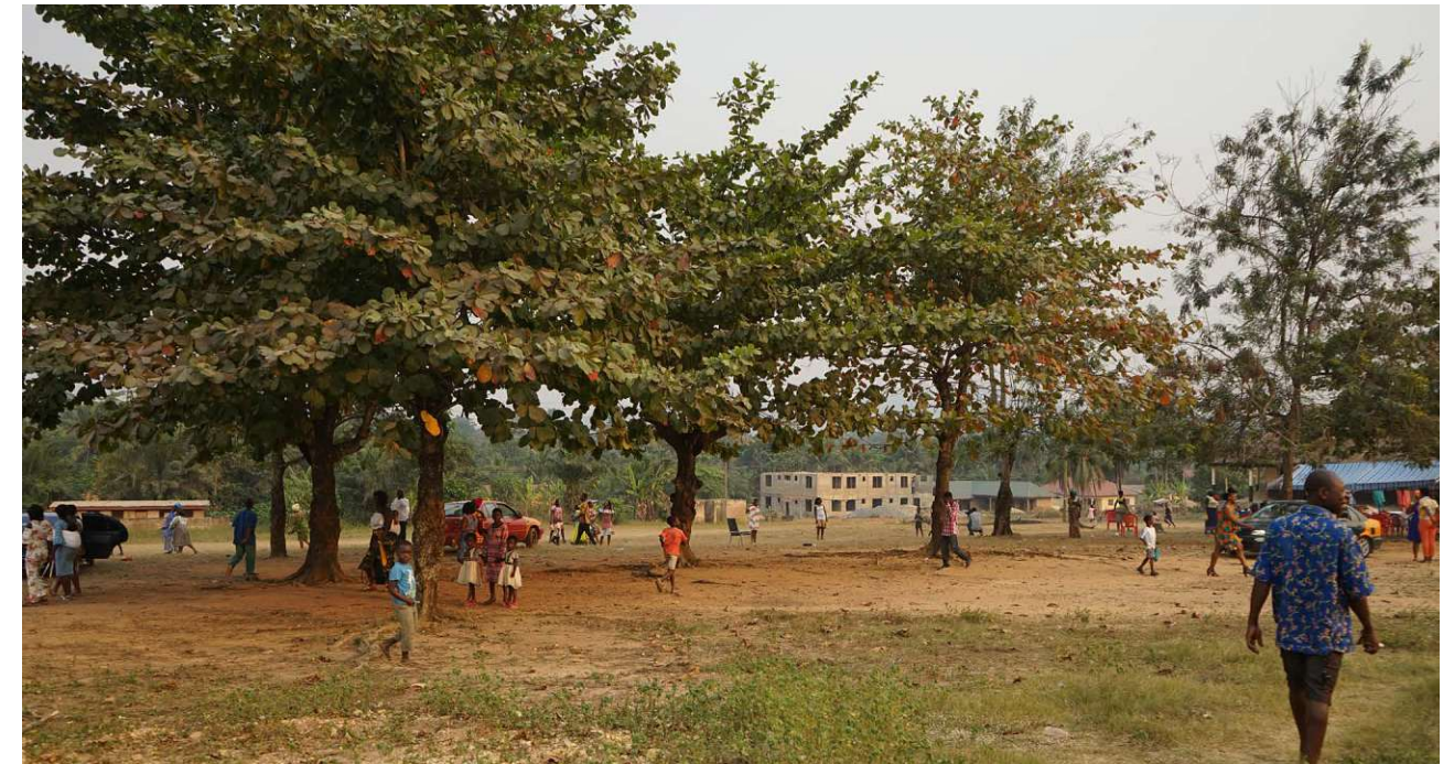
Fig.134: Construction site I February 2020
