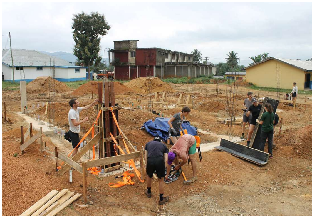
Fig.146: Setting up the formwork for the reinforced concrete columns | Week 4
