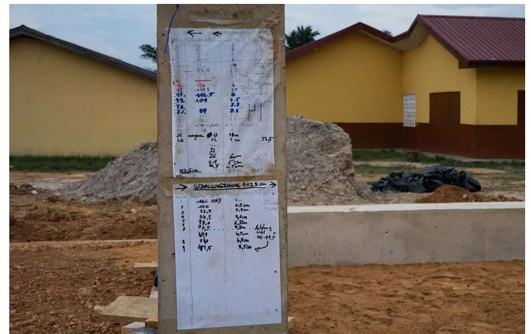
Fig.193: Ramming protocol
