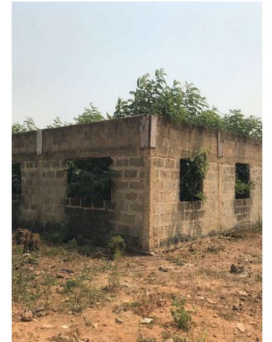
Fig.77: Unfinished structure of the community centre
