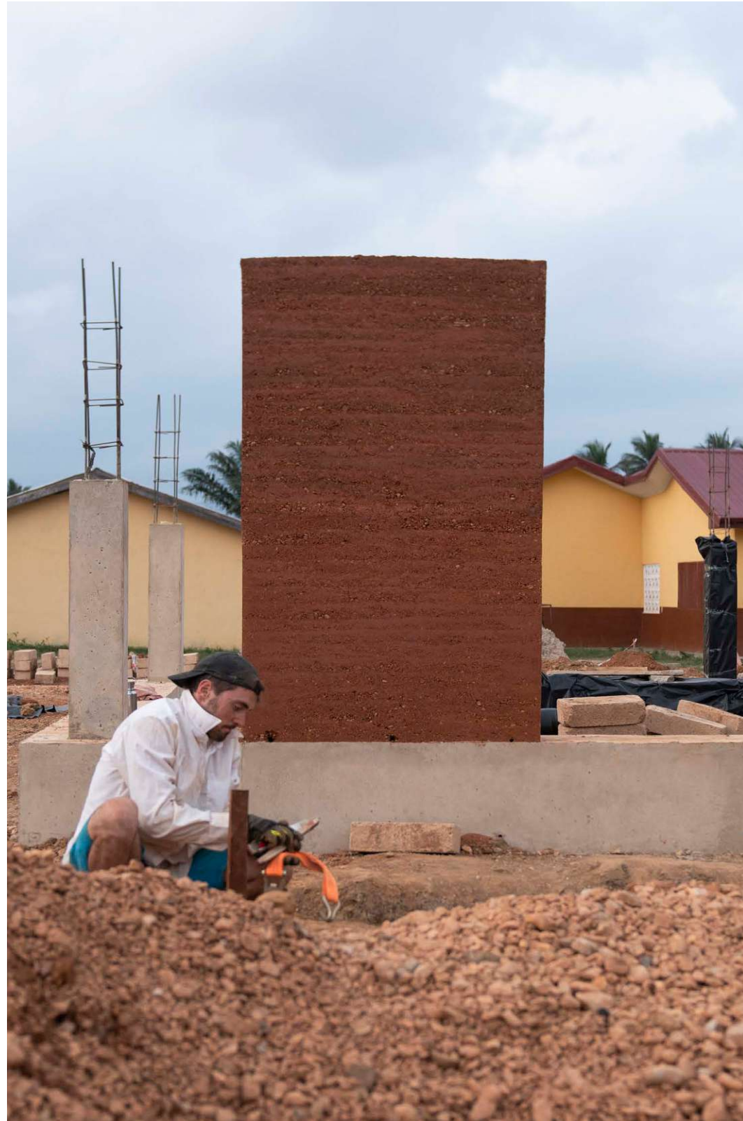
Fig.204: First completed rammed earth wall | Week 5
