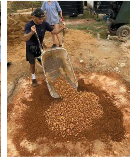
Fig.181: Then the larger stones were added
