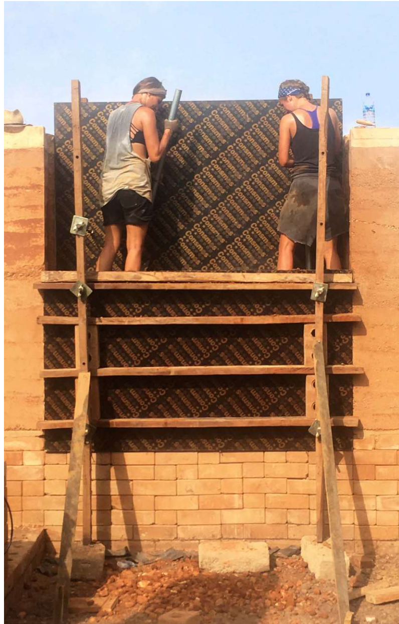
Fig.70: Wooden rammed earth formwork | North Ghana
