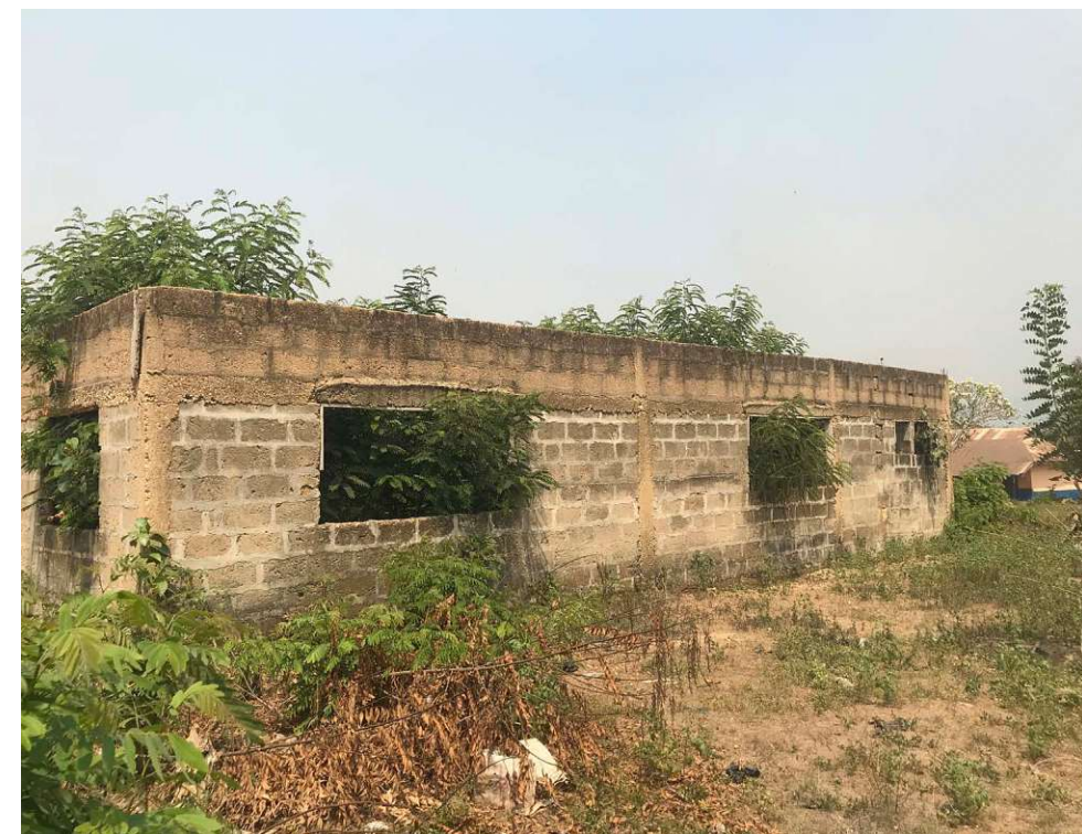
Fig.88: Unfinished structure of the community center
