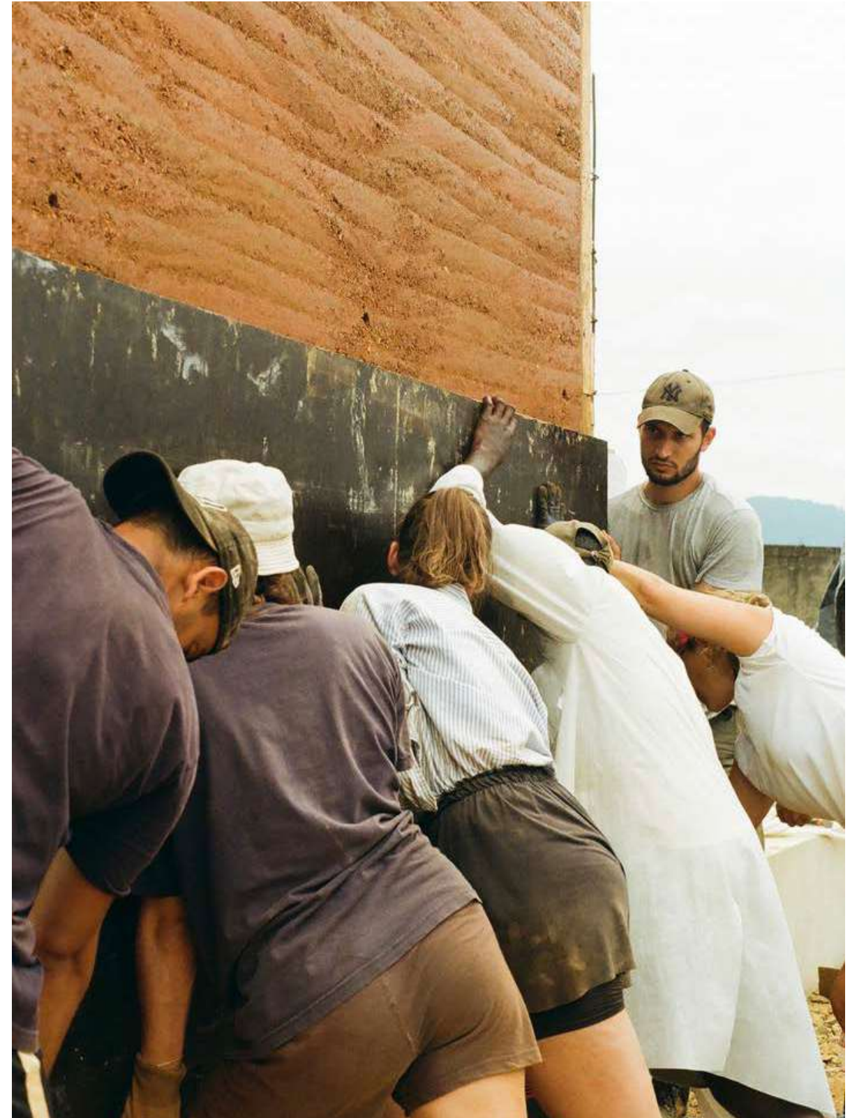
Fig.200: Removing the formwork
