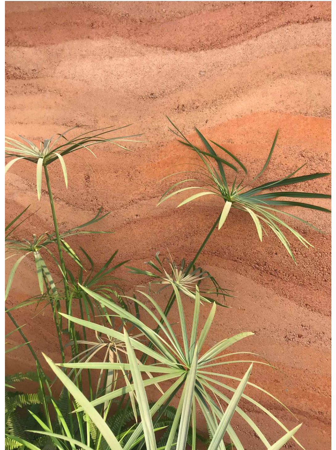
Fig.26: Rammed earth wall from Hive Earth Studio | Accra 2020
