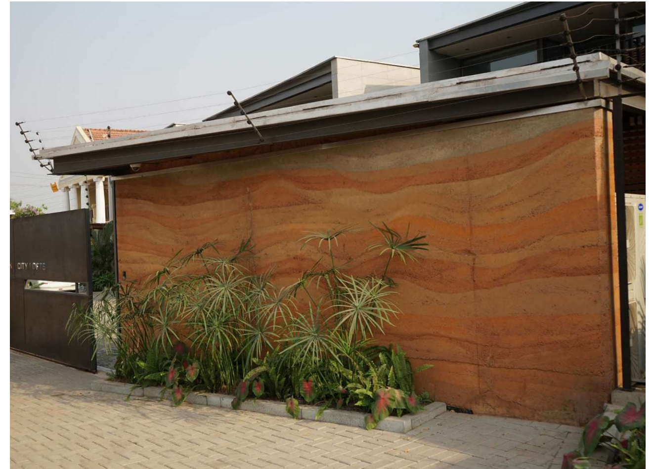
Fig.69: Rammed earth wall | Accra
