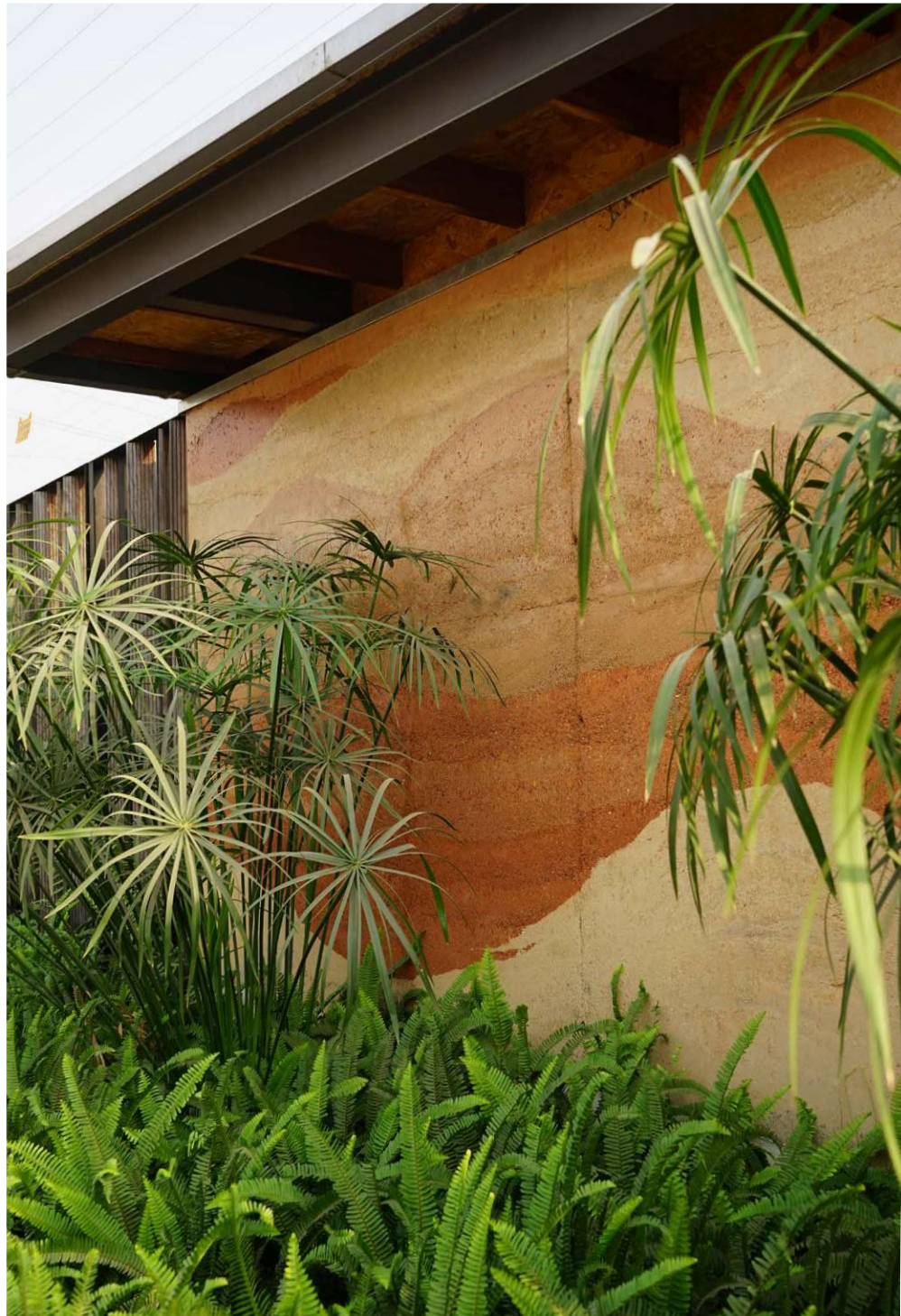
Fig.25: Rammed earth wall from Hive Earth Studio in their signature technique „waves“ | Accra 2020
