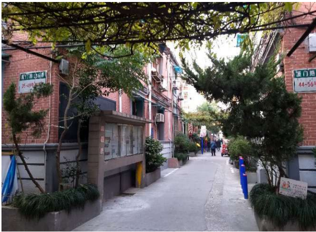
Main alley in West Guizhou Lilong
