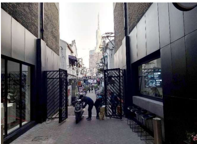
View north along Yanqingli's main alley
