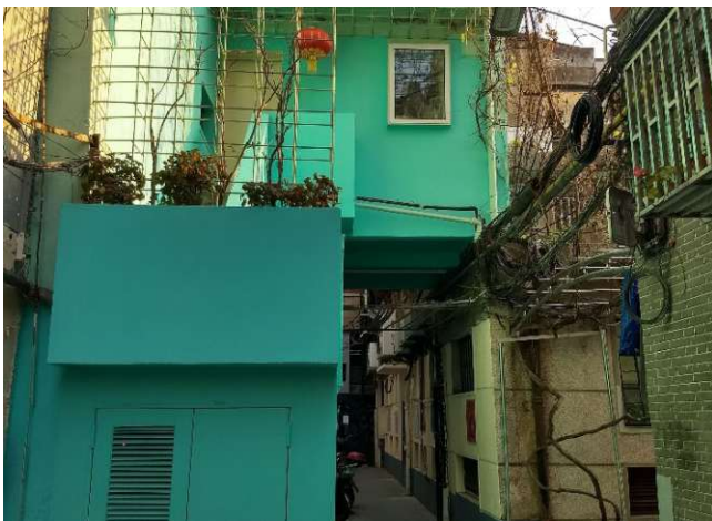
Public Reading Room at West Guizhou Lilong [3]
