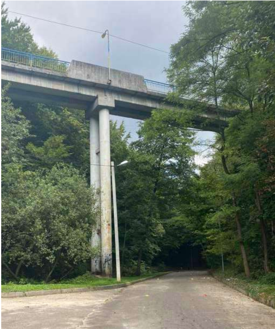
Fig. 152 Pedestrian bridge in Pohulianka Forest Park
