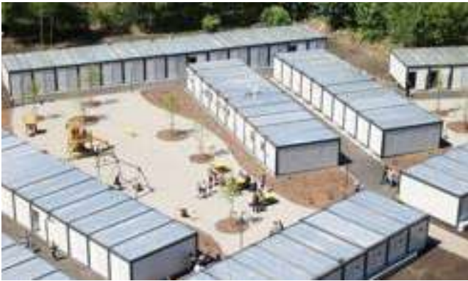
Fig. 85 Playground in modular settlement in Lviv
