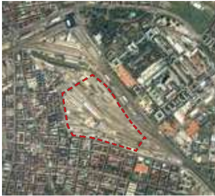
Fig. 31 Former railway depot
