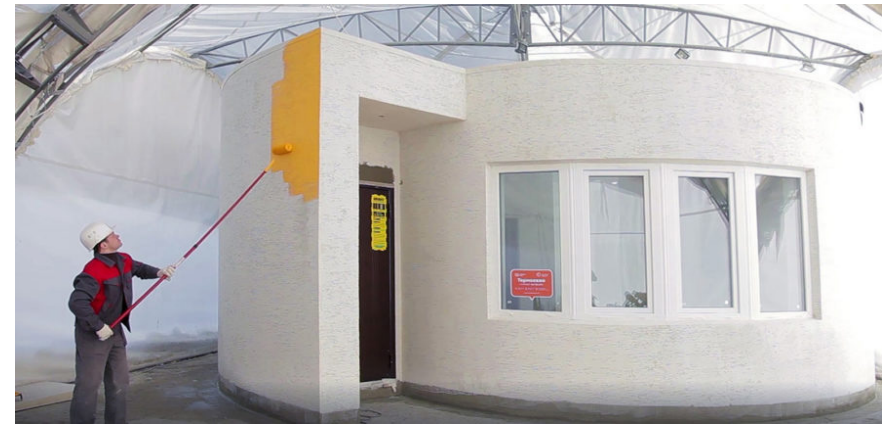
Fig.4.29. Plaster finishing
