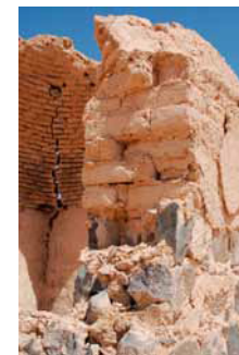
Fig.2.38. Mud wall built on stone foundation, Mecca and Dipasquale, 2009
