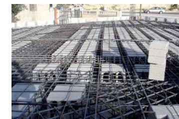
Fig.2.41. Concrete hollow block, Helmedag, 2012
