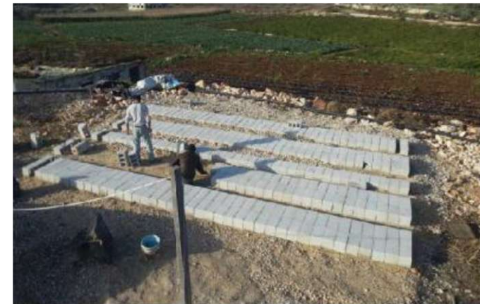
Fig.4.14. Assembling earth ducts, Najjar, 2017
