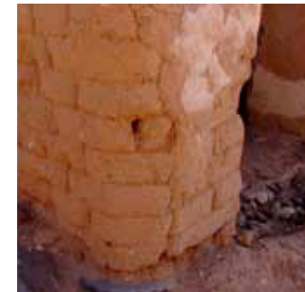
Fig.2.37. Mud wall built on the ground, Mecca and Dipasquale, 2009
