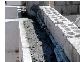
Fig.2.41. Concrete hollow block, Helmedag, 2012
