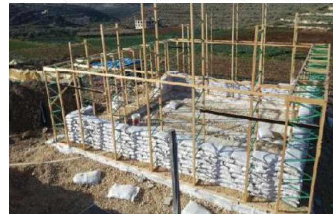
Fig.4.15. Sand bag stacking and assembling Eco-beams, Najjar, 2017
