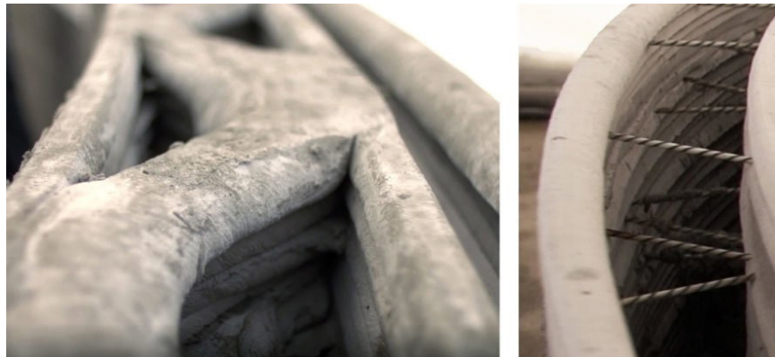
Fig.4.28. 3D printed wall and the added fiberglass
