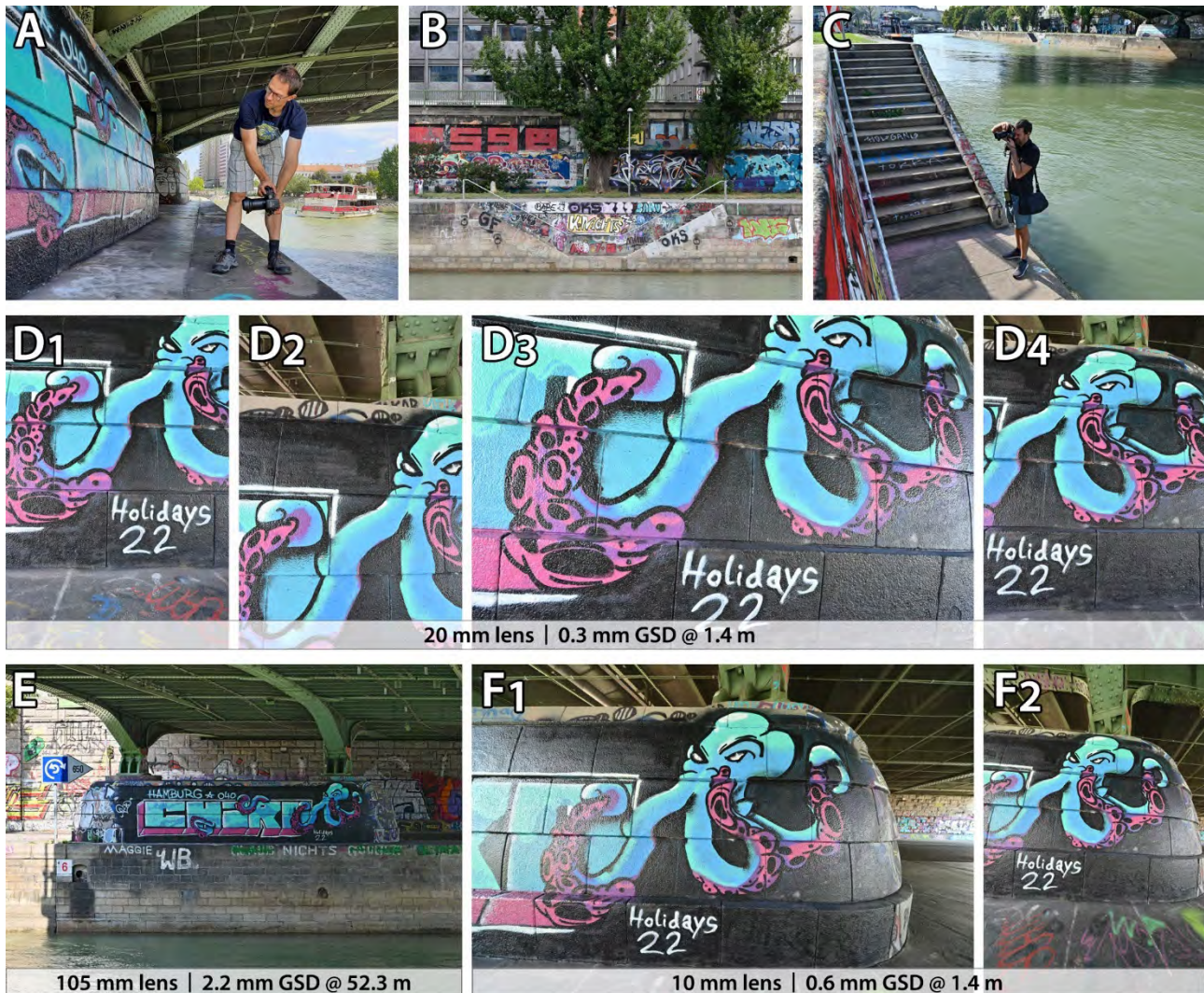
Figure 13. Three surfaces that are difficult to photograph appropriately. A) water-facing parts of some bridge pillars with only 1.5 m of manoeuvring space until the embankment edge; B) embankment surfaces just above the waterline and (together with C) narrow staircases embedded in these embankments. The current solution is photographing cases A and C with a 20 mm lens. Insets D1 to D4 show some results of the bridge pillar in A. Note that the camera is usually held vertically in a low position (like A and resulting in D1) and then lifted to yield D2. The considerable image overlap is necessary for SfM purposes. A horizontal or landscape camera rotation (D3) would necessitate at least three images to incorporate some parts of the unchanged surroundings (like the floor or the green metal parts of the bridge pillars). A photo covering a small portion of the ground and metal bridge parts (like D4) is uncommon; one needs to hold the camera above the water, thus creating an unstable and dangerous acquisition position. The lower row presents two possible solutions to this problem. Acquiring a photo with a longer focal length lens (E) takes away the risk and will always yield a lot of surrounding elements, which are necessary for the incremental SfM algorithm (see Wild et al. in this volume). Still, this solution delivers a GSD about twice the threshold set by INDIGO. In addition, one also must cross the channel to photograph. Using an extreme wide-angle lens avoids this time cost. F1 and F2 show that a 10 mm lens can capture the element of interest plus surrounding structures with both a horizontal (F1) and vertical (F2) camera rotation (for reference, compare F1 with D3 and F2 with D4). With this solution, the photographer needs fewer photos or can move slightly closer to the pillar element, making acquisition safer. Although the GSD is twice that of the 20 mm lens, it is still far below the 1 mm threshold.
