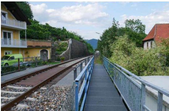
Narrow walkway to reach Schwallenbach station. Will need to be modified to comply with barrier free accessibility.
