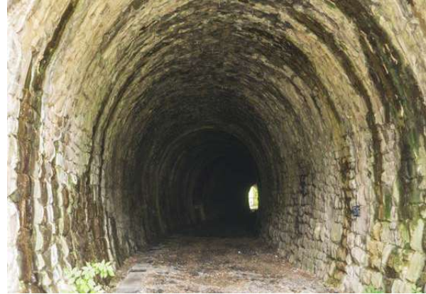
KM 48.9: West portal of the Schallmarbacher tunnel. Note S curve in the middle of the tunnel. No visible deterioration or drainage issues.
