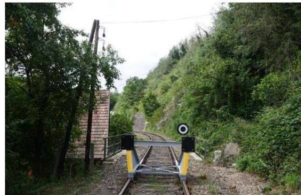
End of operable track on the eastern end of the Donauuferbahn
