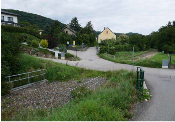
KM 47.8: Small concrete box culvert. Appears in good-very good shape.
