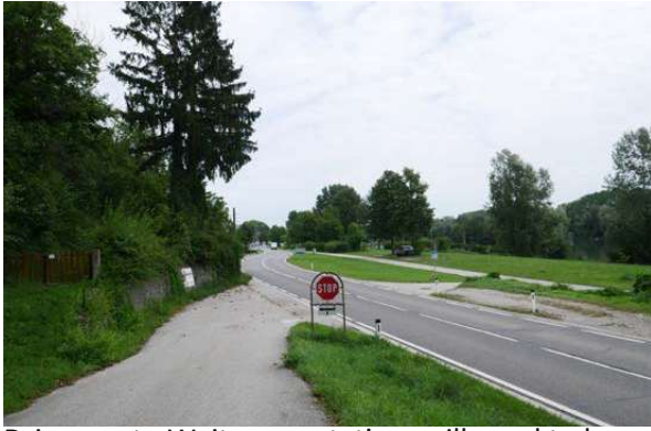
Driveway to Weitenegg station, will need to be modified for bus access
