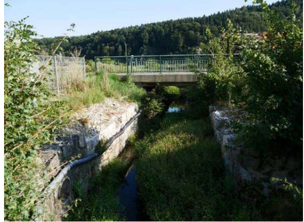
KM 58.2: Small metal span removed.
