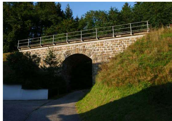
KM 65.2: Bridge at Hirschenau-Nöchling
