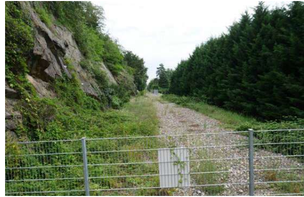
Right of way Lehen-Ebersdorf looking east.
