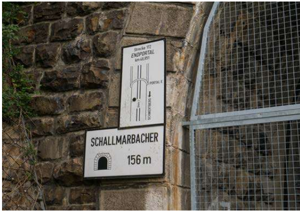
KM 48.9: West portal of the Schallmarbacher tunnel. Note S curve in the middle of the tunnel. No visible deterioration or drainage issues.
