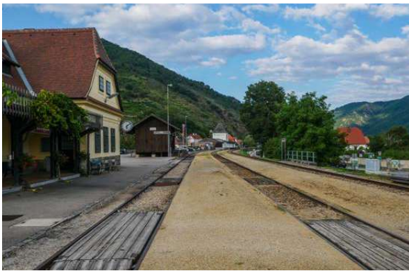
Track layout at Spitz. Provision of barrier free platforms will require innovative solution. Modification of track layout undesirable.
