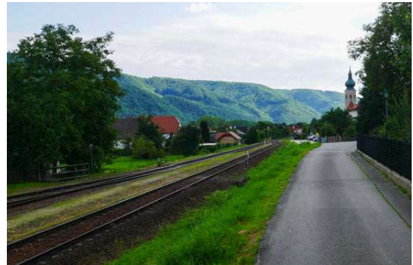
Looking west from Aggsbach station. Track closest to the station is the shortest and could be potentially removed
