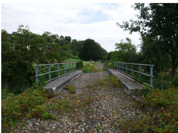
KM 47.2: Small arch culvert, in good condition with concrete deck.
