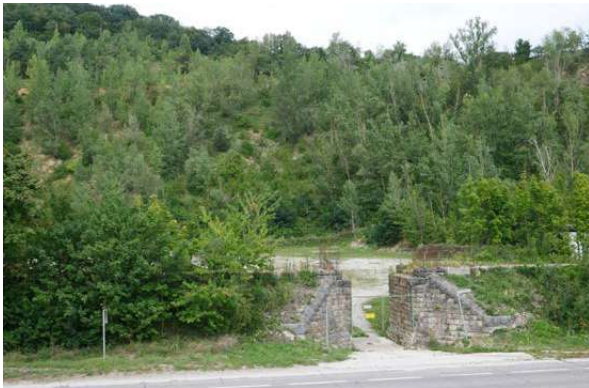
KM 41.3: Removed bridges at entrance to quarry.
