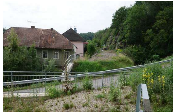
Lehen-Ebersdorf looking west, right of way broken to regrade road.
