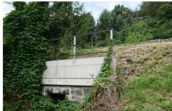
KM 39: Renovated stone box culvert
