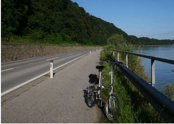
Track alignment along road elevated on a stone embankment
