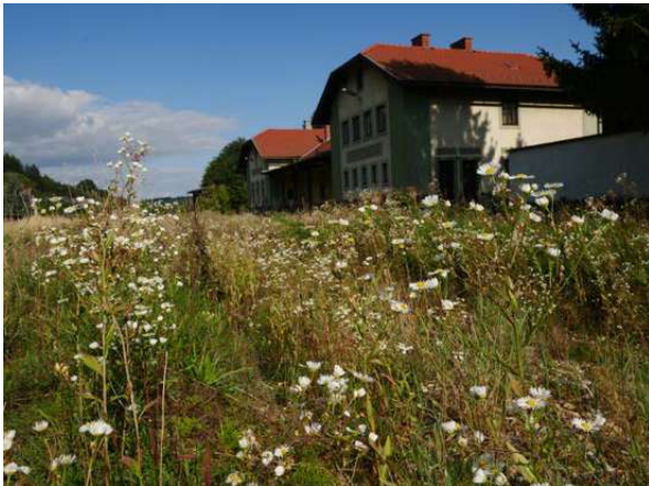
Station in Persenbeug with abandoned former rack area.
