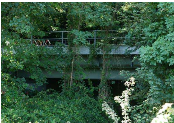
KM 57.3: Newly renewed bridge over stream
