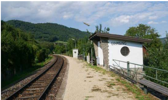
Grimsing station shelter
