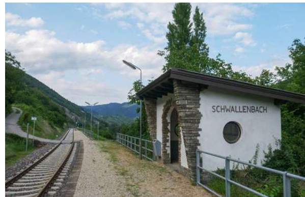
Station shelter at Schwallebach.
