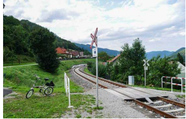
Access to station via level crossing
