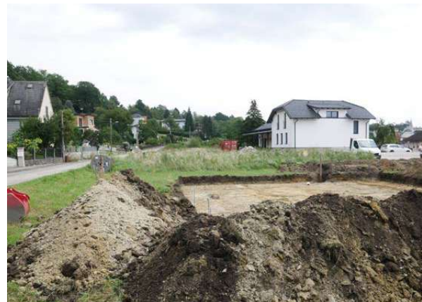
43.9: Foundations for structure being poured in former track area.
