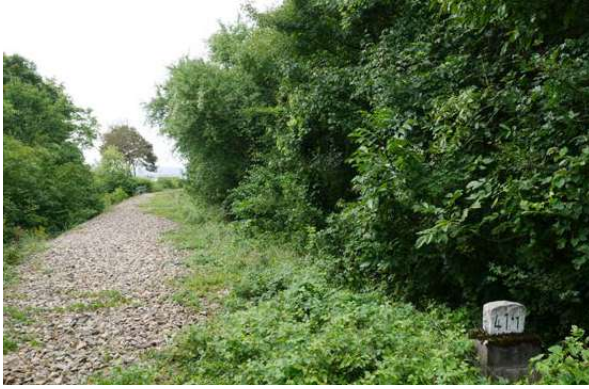
KM 41.1: Right of way condition
