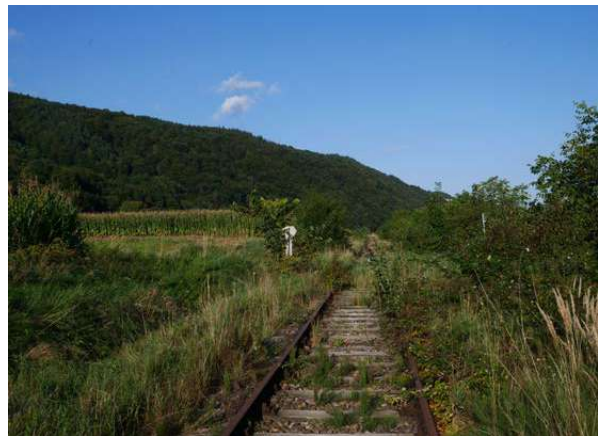
KM 58.8: view looking east, track shows no sign of recent use
