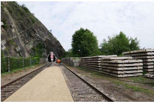
Track materials salvaged from the middle segment stacked for reuse.
