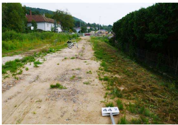
KM 44.2: Right of way with fallen kilometer post
