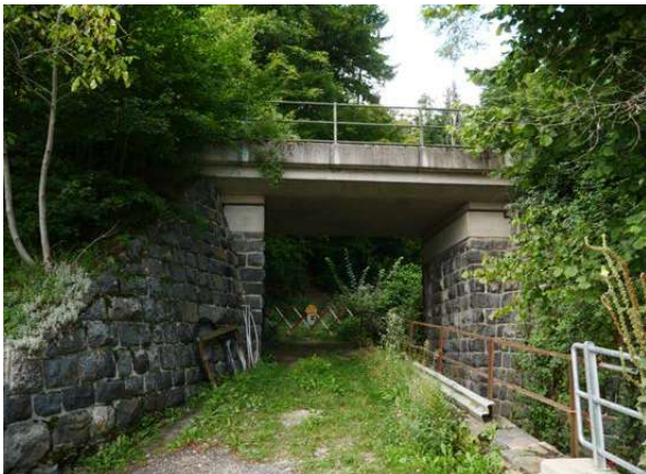
KM 51.5: Completely rebuilt concrete deck bridge in very good condition
