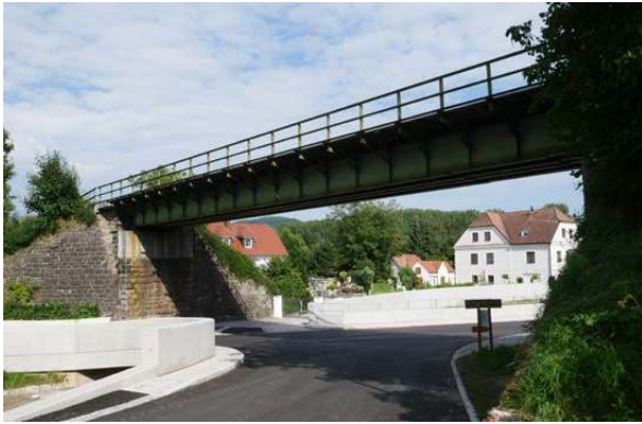
No station, location considered for transfer node between the railway and Melk.
