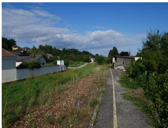
Western exit of station
