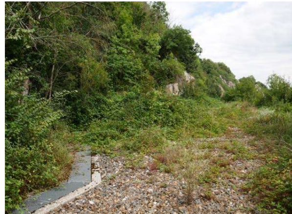
KM 49.5: Relatively new drainage improvements along right of way.
