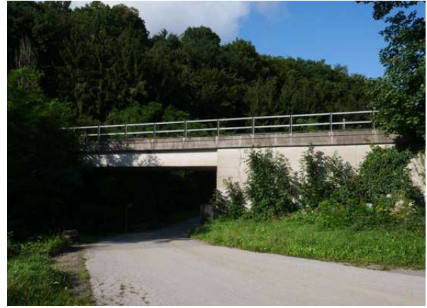
KM 56.3: New concrete bridge in very good condition
