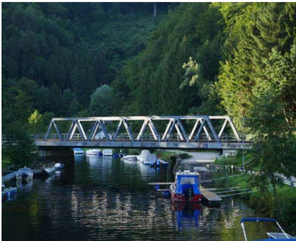
KM 61.1: Newly constructed bridge over the Ysper river. Track is however in bad condition.
