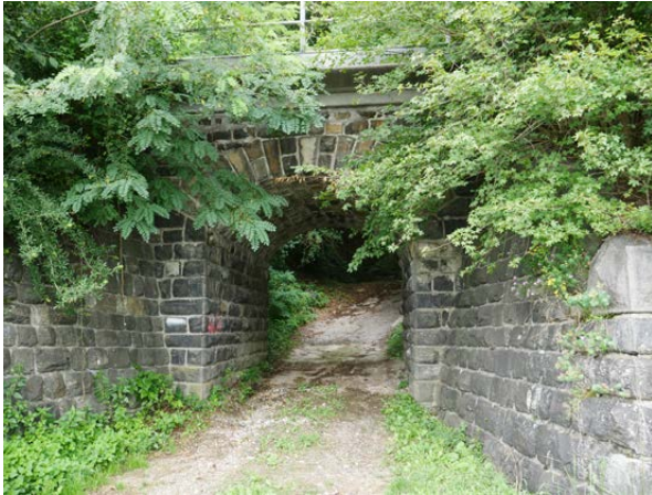
KM 46.4: Arched road underpass. Bridge is in good shape with new concrete deck
