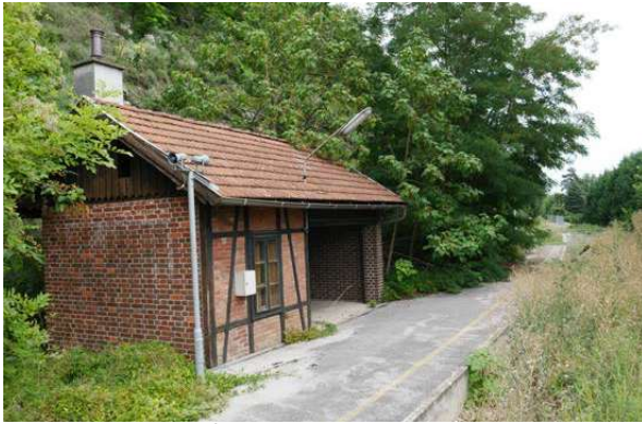
Lehen-Ebersdorf station shelter
