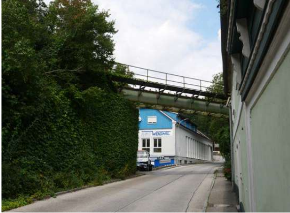
KM 49.2: Bridge over the Steinbachstrasse. Metal deck structure. Bridge appears in poor to fair shape with significant rusting.
