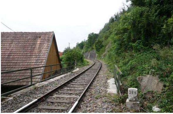
KM 38.6: Small box culvert past the buffers.
