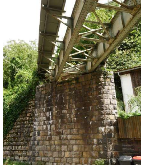
KM 49.2: Bridge over the Steinbachstrasse. Metal deck structure. Bridge appears in poor to fair shape with significant rusting.
