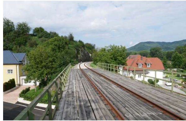
Track level view of bridge at Schallemersdorf.
