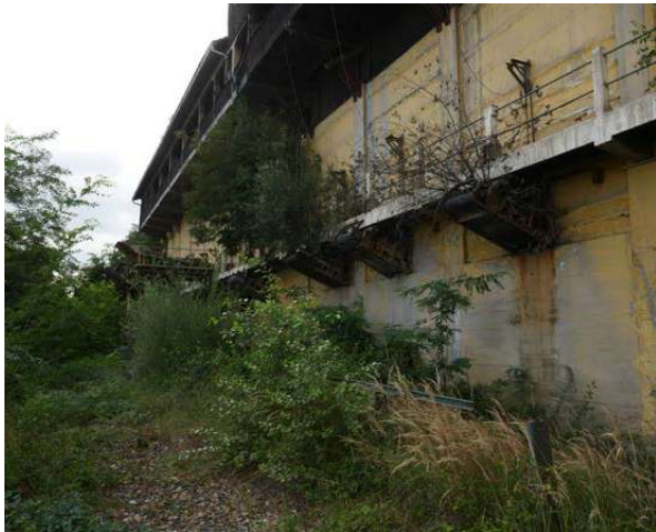
Old loading silos, track area heavily overgrown.
