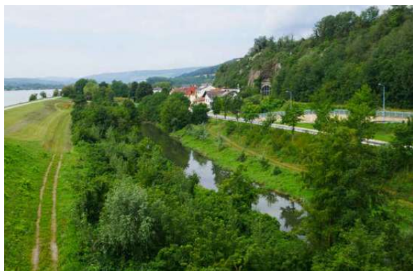
KM 43.1: Eastern portal of Klein-Pöchlerner Tunnel viewed from Danube road bridge
