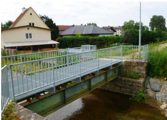
KM 44.1: Bridge over small channel. Bridge is being repurposed for pedestrians.
