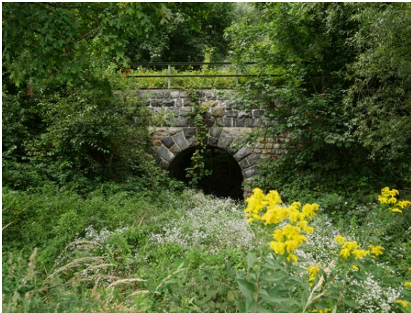
KM 51.1: Small stone arch bridge, appears in good but unrenovated condition.
