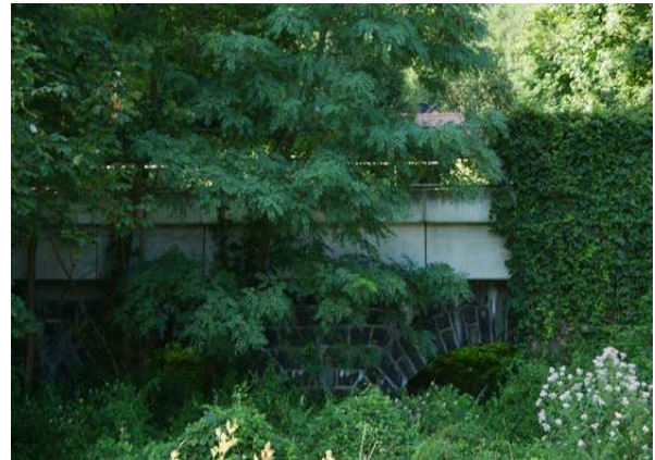
KM 57.3: Newly renewed bridge over stream
