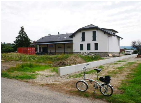
43.9: Klein-Pöchlarn station building, construction of wall across former track area.
