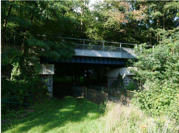
KM 56.9: New metal deck bridge over a stream
