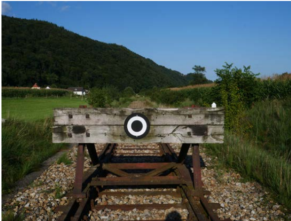
KM 58.7: Buffer post at the end of the intact trackage
