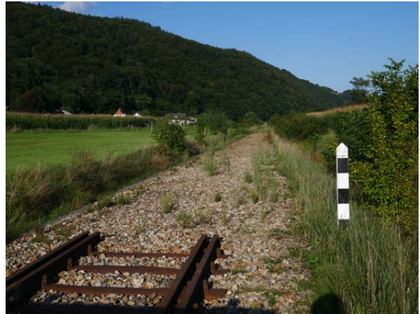
Station building in use as cafe. Valuable space directly adjacent to the platform is wasted on parking on parking for non rail users.
