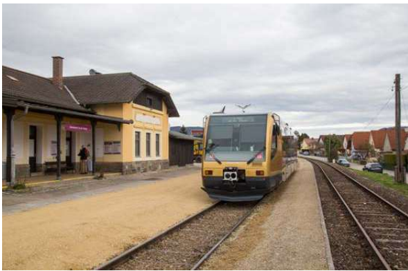
Train at end station of Emmersdorf. Outside track has already been removed enabling future barrier free access.
