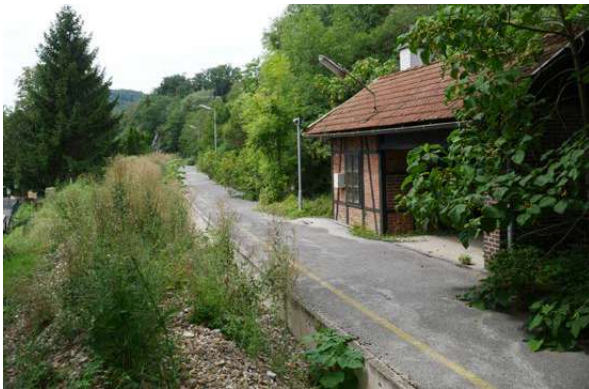
KM 40.106 Lehen - Ebersdorf halt. 2010 vs 2021. Track materials have been removed and ballast piled in center of old alignment. 2010 image Wikipedia CC
