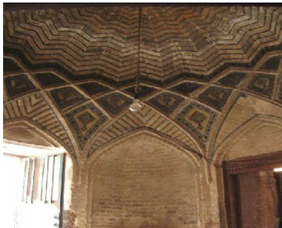
Figure 3-20 Execution of details on the ceiling of the entrance vestibule
