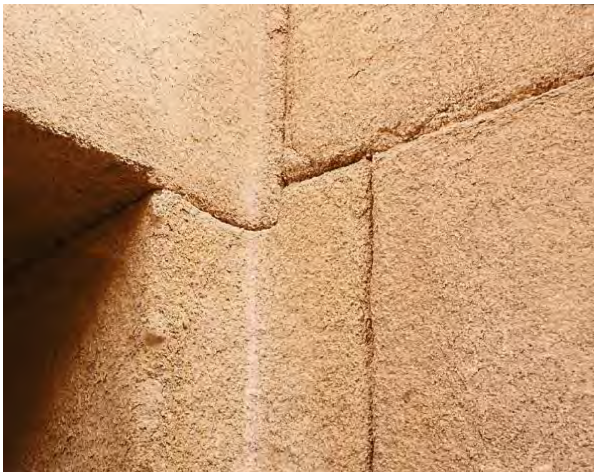
Figure 171 Close up of corner at Temple of Osirion, Egypt
