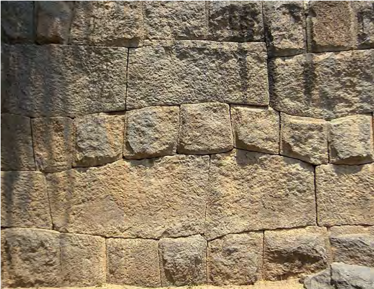
Figure 28 Wall close up, another location in the same complex, Warangal, India
