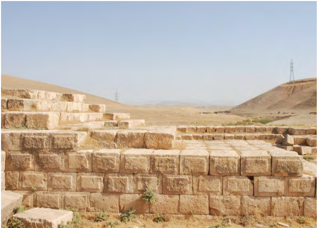
Figure 5 Jerwan Aqueduct, Iraq
