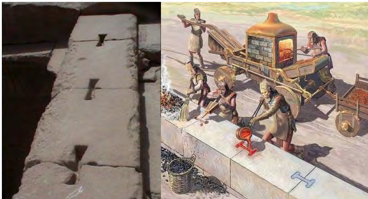
Figure 169 Metal clamps in ashlar (left) and how they are possibly made (right)
