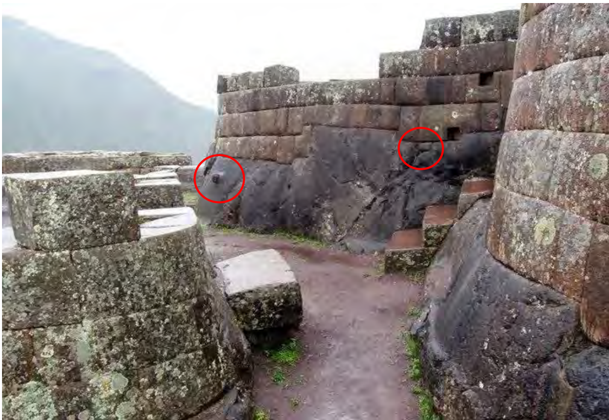
Figure 158 Another perspective displaying the nub and the filler block on the bedrock in Pisac, Peru
