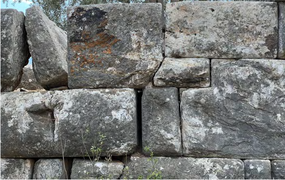
Figure 80 Close up of the filler block in Euromos, Turkey
