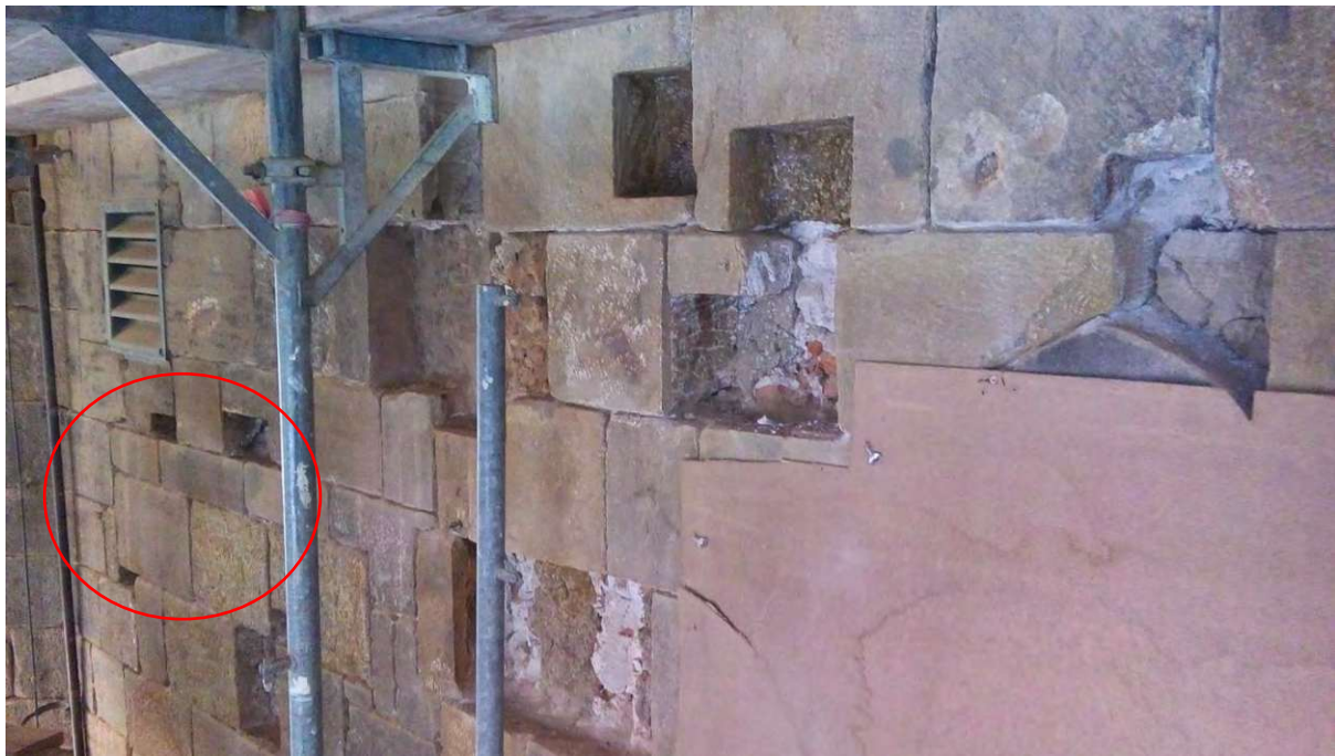
Figure 84 Dutchman repair ( Vierung )
