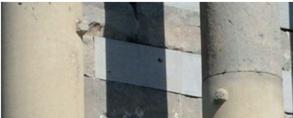
Figure 42 Red marked area zoomed in, displaying nubs on column segments, in Temple of Garni, Armenia
