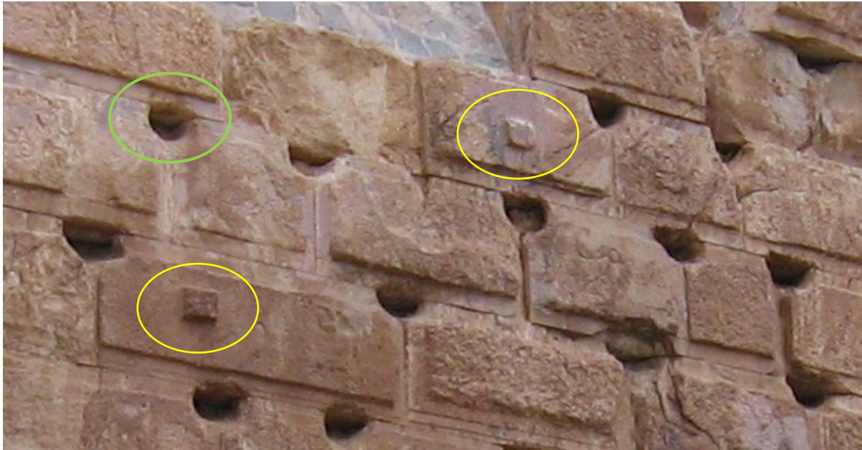
Figure 24 Red marked area zoomed in, displaying, nubs (marked in yellow) and joint/corner holes (marked in green) in Pasargadae, Iran
