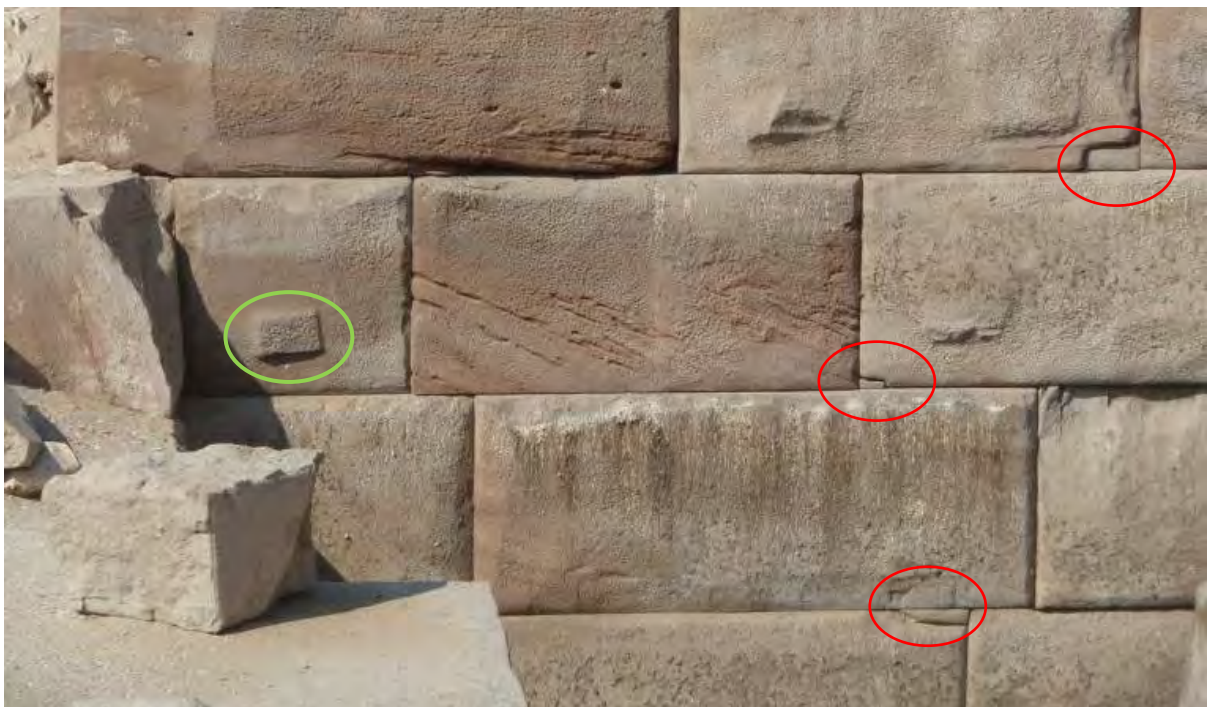
Figure 76 Another perspective of the same wall, displaying filler blocks along with a nub (marked in green) in Temple of Osirion, Egypt
