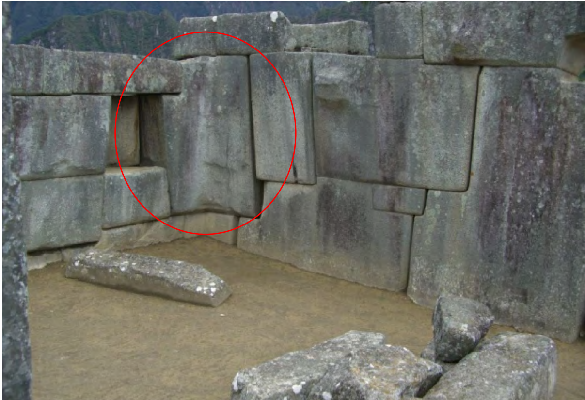
Figure 173 Rounded corner at Machu Picchu, Peru
