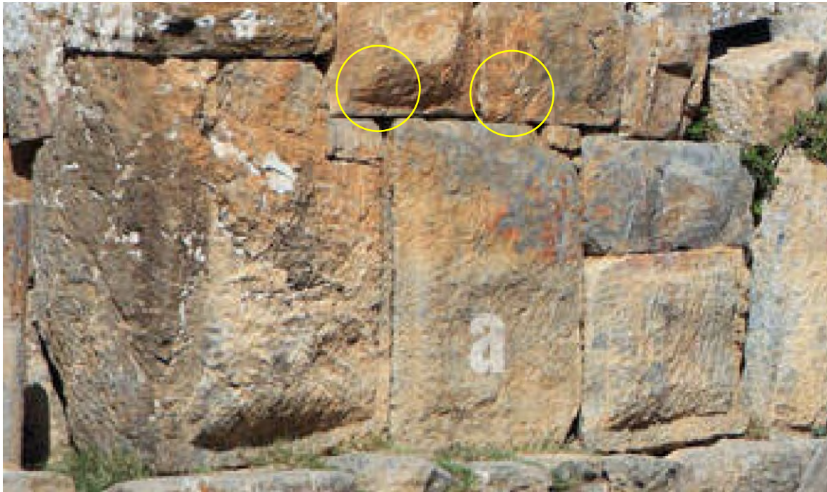
Figure 11 Yellow marked area zoomed in, displaying filler blocks, in Djemila (Cuicul), Algeria
