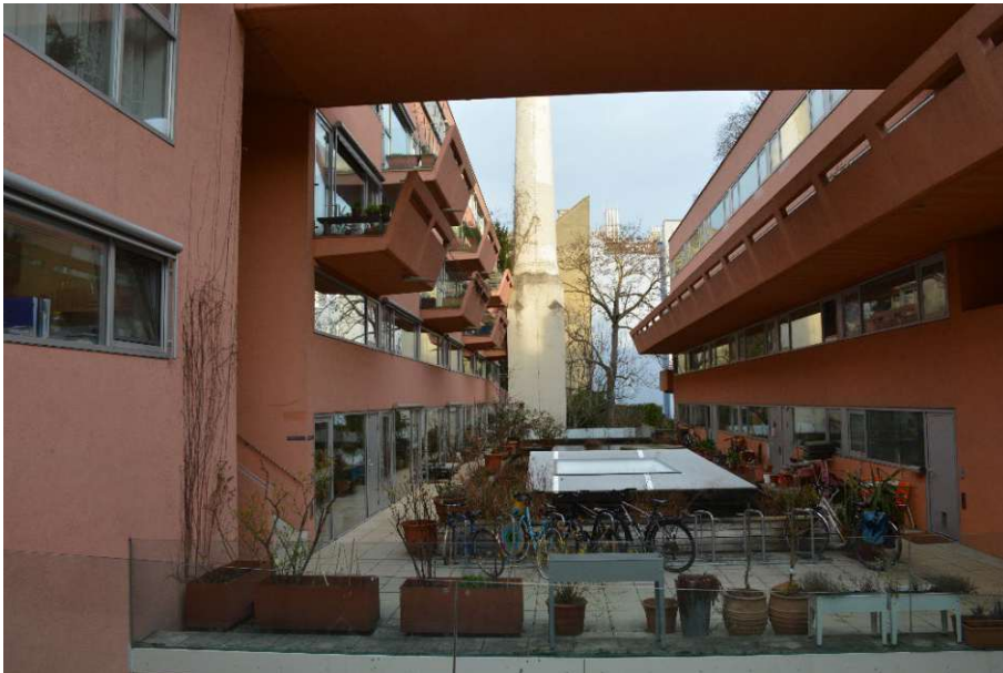
Fig. 54: Semi-private space above the bathhouse, Sargfabrik (own photograph, 2023)
