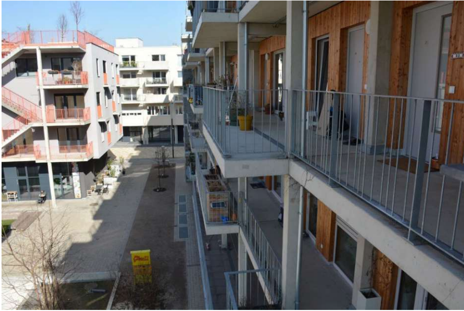
Fig. 38: Northwestern building side of Gleis 21 (own photograph, 2023)
