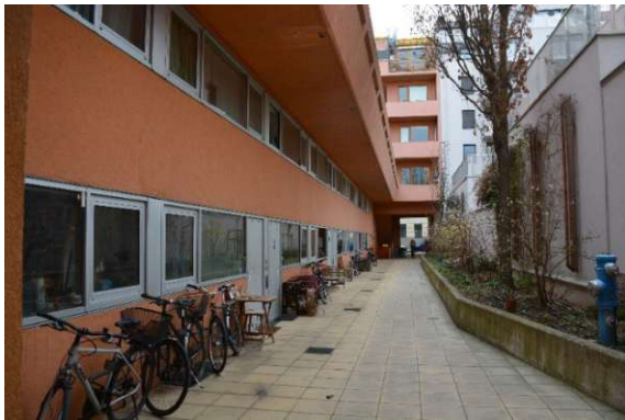
Fig. 57: Semi-public path, Sargfabrik (own photograph, 2023)
