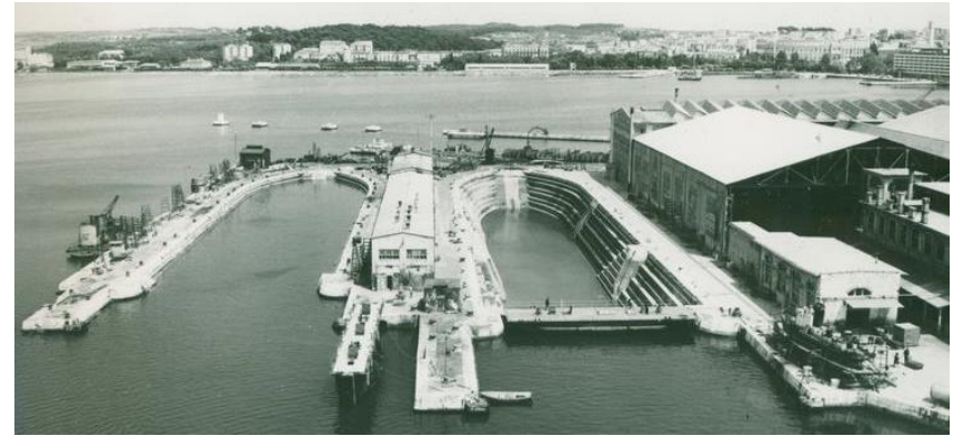
Figure 25 | Water regulated ship docks on the side of the island
