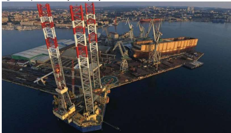
Figure 34 | Aerial view of a sea platform construction
