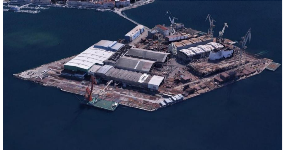
Figure 71 | South-East aerial view of Uljanik island
