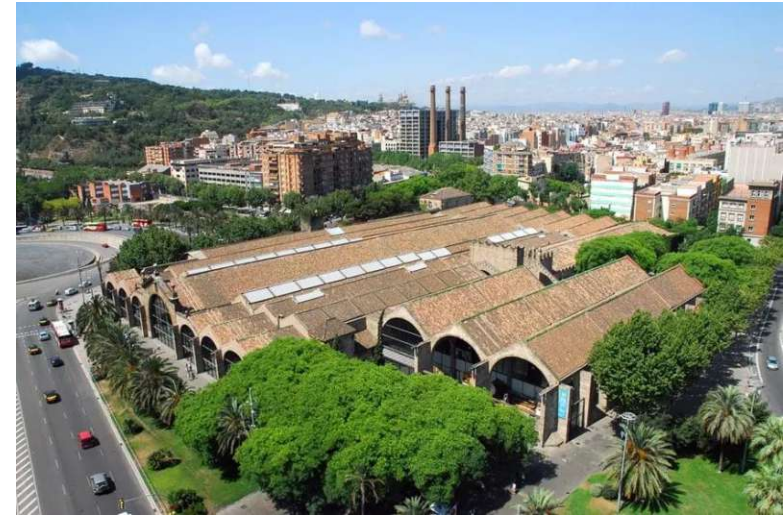
Figure 57 | Arial view of refurbished hangars
