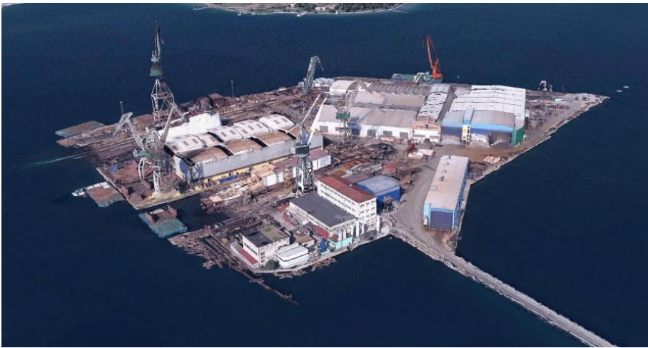
Figure 70 | North-West aerial view of Uljanik island
