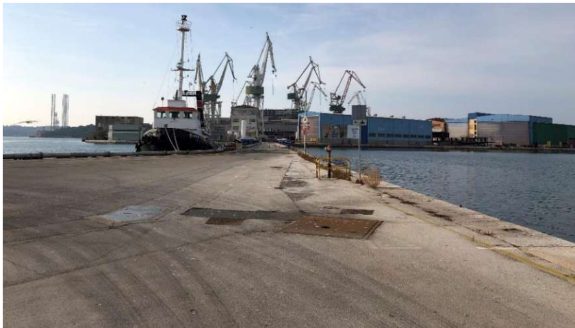
Figure 66 | Approach to the island bridge
