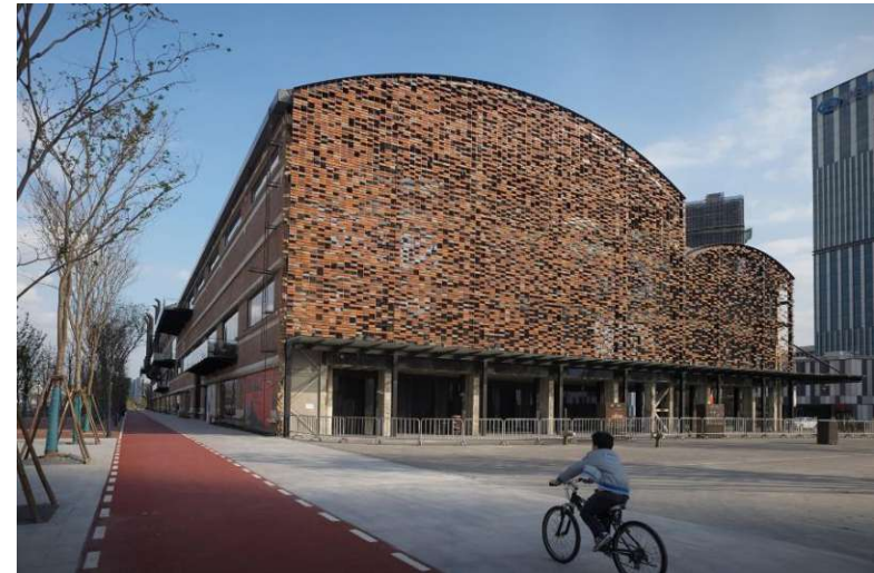
Figure 59 | New brickwork façade; West side of the building
