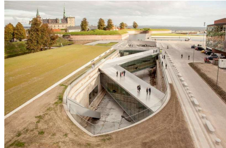
Figure 61 | Repurposed drydock with new walkways and interior space
