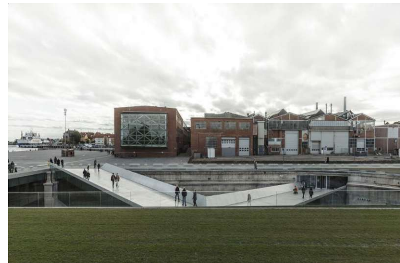
Figure 62 | West side view of repurposed drydock
