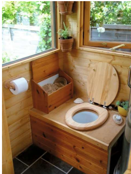
fig.26- an example of composting toilet
