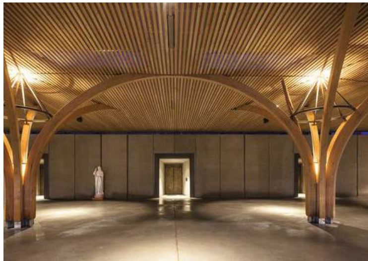
fig.48- supporting tree-like columns
