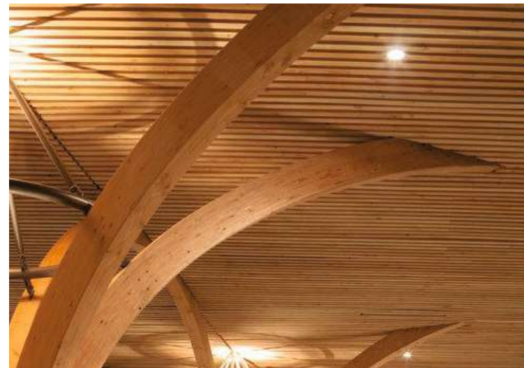
fig.49- branches of tree-like columns
