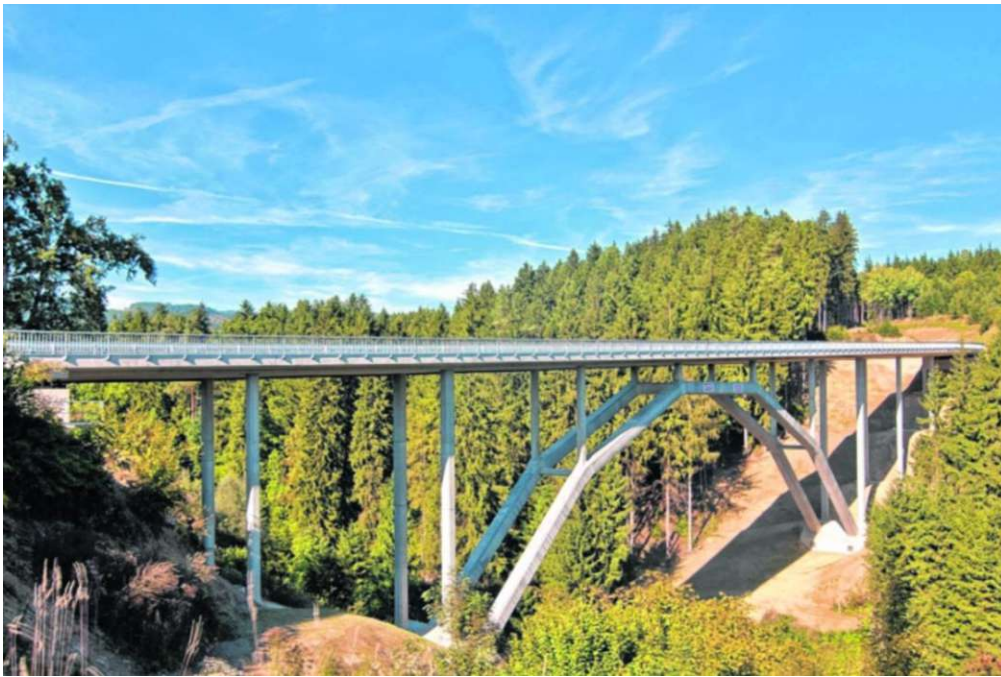
Figure 2.1: Wild Bridge in Völkermarkt, Austria built of UHPC concrete [6]
