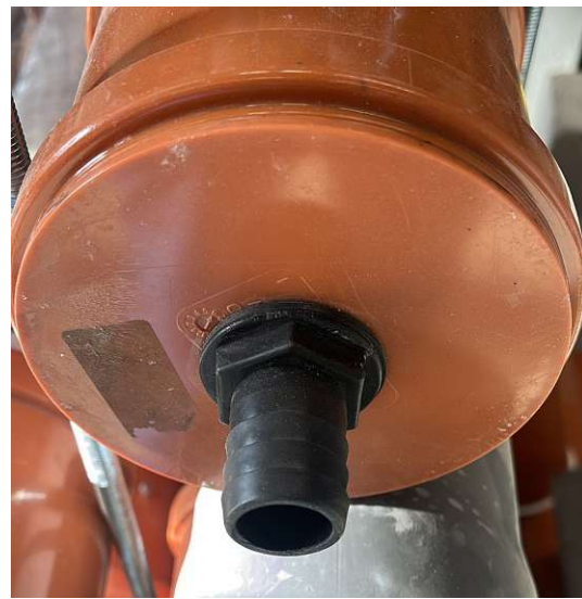
(b) Hose connection adapter
