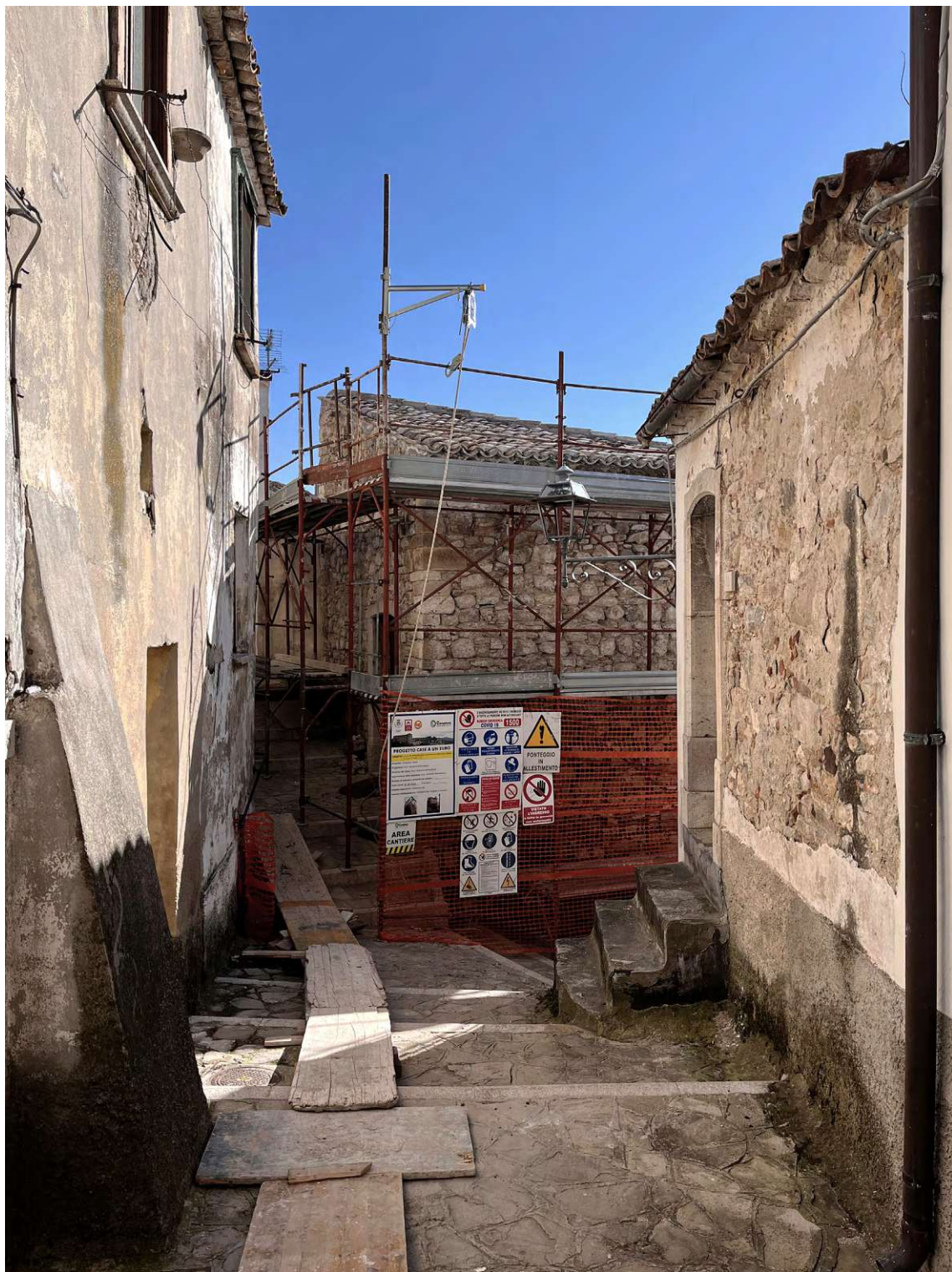
Fig.83 Construction site of €1 House project
