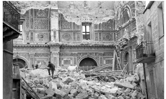
Fig.112 Traces of the severe earthquake
