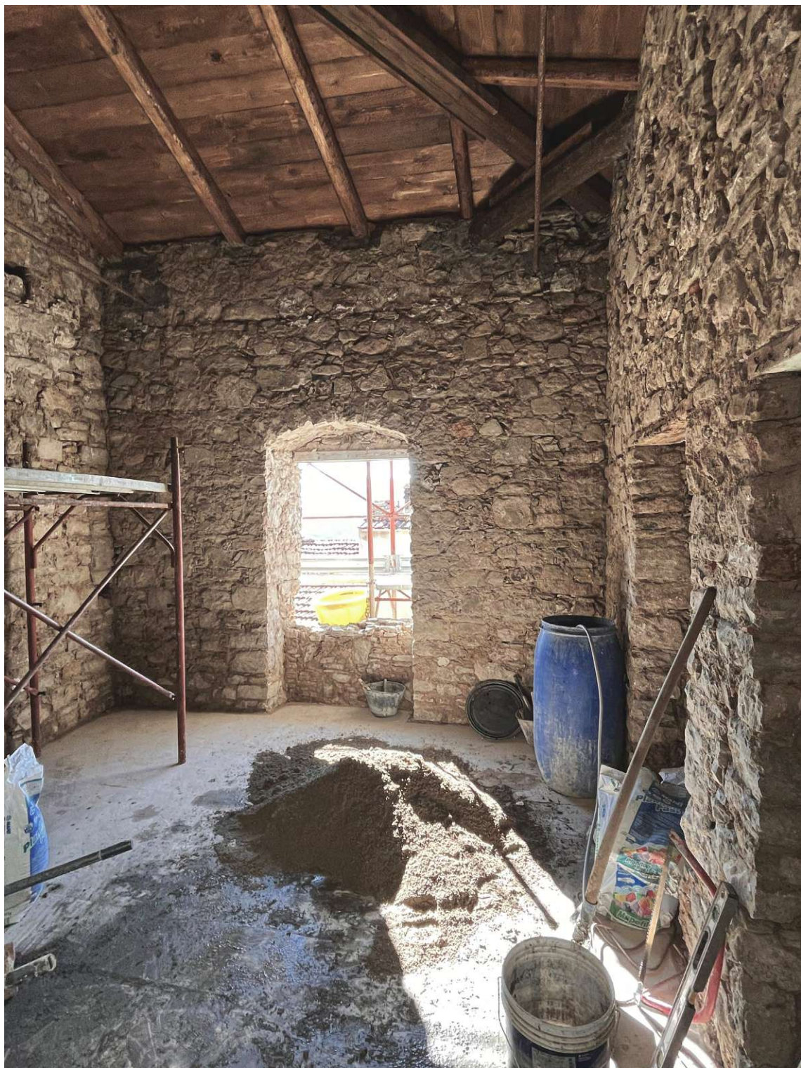
Fig.95 Construction work in Zungoli
