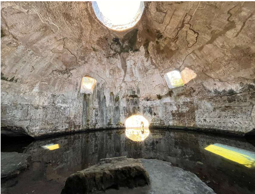
Fig. 34 Thermae die Baiae, Temple of Mercury. First quarter of 1 st century A.D. Domed Natatio, diameter 21,55m. Four niches diagonally placed not visible due to bradyseismic activities of the region. Notable absence of brick in the building of the dome.
