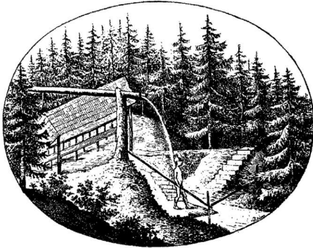
Fig. 10 Back to Nature: Priessnitz's Shower in the Silesian Woods. A source is captured and channeled through pipes open to the sun. The shower is taken on a wooden platform built out over the stream. Half a century after Rousseau's Back to Nature, the romantic outlook helped to win acceptance for the water therapy of Priessnitz and others. (Philo vom Walde, Vincenz Priessnitz, Prague, 1884), Giedion, 1970
