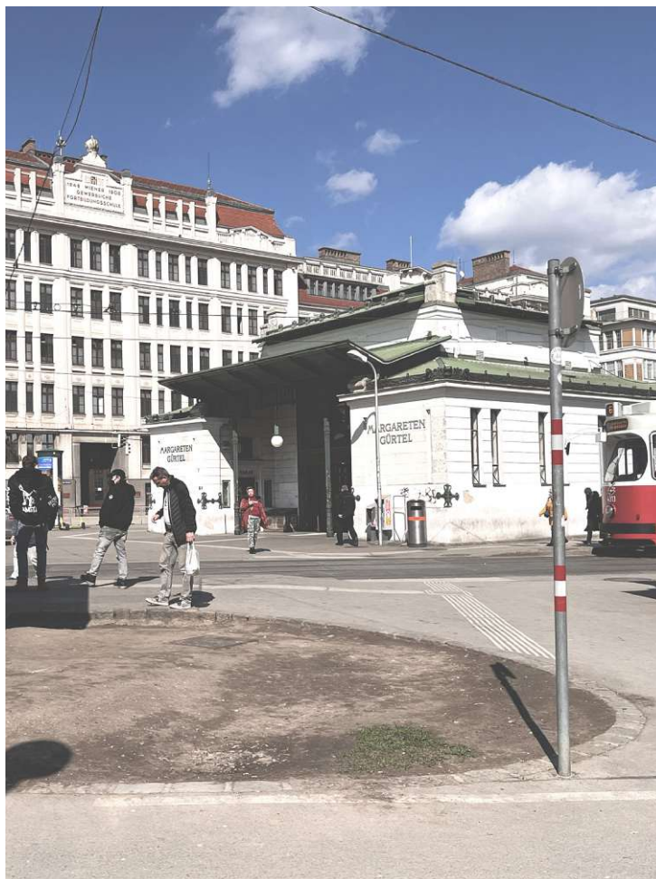
Fig. 71 One of the Otto Wagner's metro stations - U4 Margareten, former commercial training school in the background
