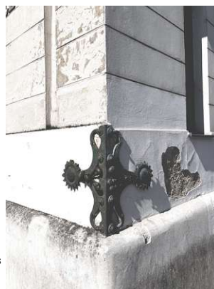
Fig. 79 Detail of the wall's corner at the station.
