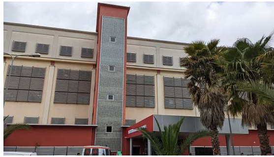
Figure 5.1: A building in the University Hospital Centre "Mother Teresa" (QSUNT) [Image: G.Hofmann]
