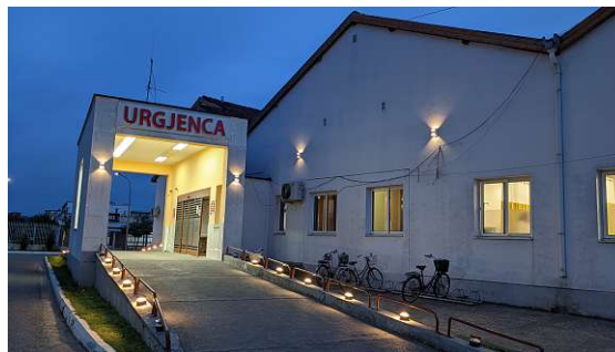
Figure 6.1: The emergency building in a regional hospital in Albania [Image: G.Hofmann]
