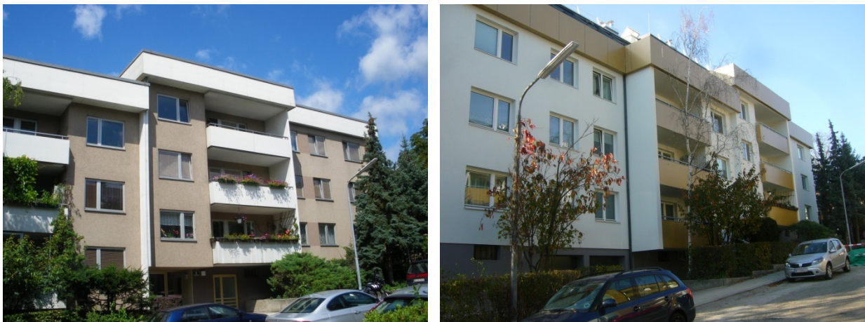
Figure 9: V_RES_BOKU2 before renovation (left), and after renovation (right) (Heidenreich, 2014, 2015).
