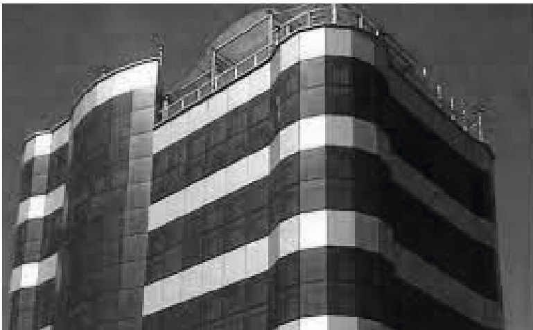
Fig. 39 Overview of the facade, https://barok-hotel.business.site/
