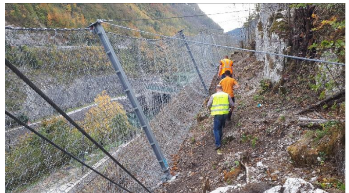
Figure 7 Inspection rockfall protection fence Kastenreith (OEBB-Infra)
