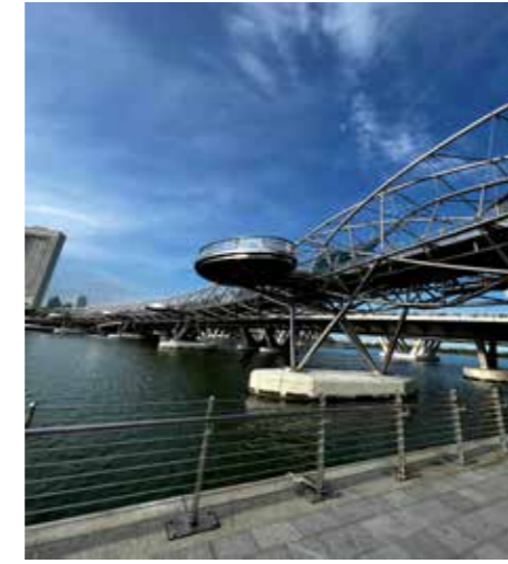
Abb.14: Singapur, Helix Bridge
